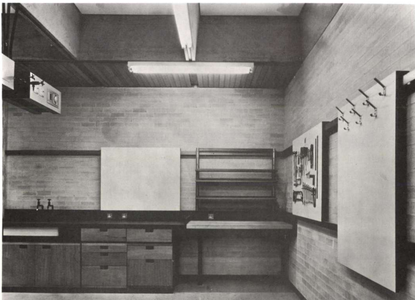
Fig. 14 below Birmingham University. Typical laboratories with a services boom on the left Photo: C. Westwood
