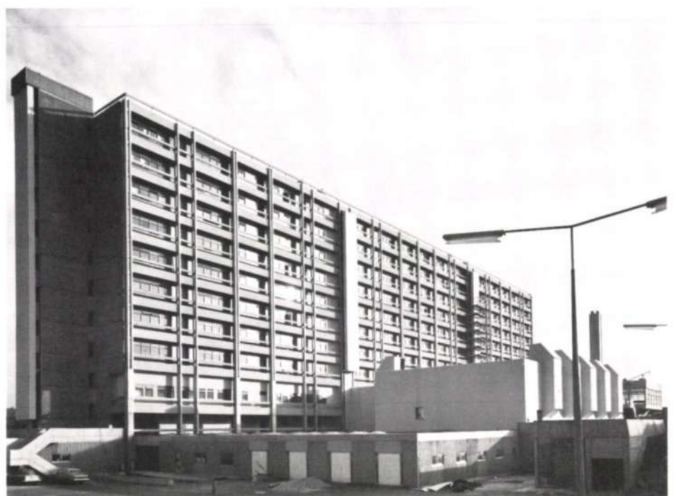
Fig. 8 below West elevation of main hospital block (Photo: W. Ralston Ltd.)
