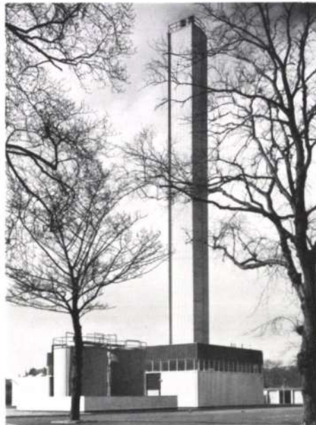
Fig. 7 left Boiler and chimney (Photo: W. Ralston Ltd.)
