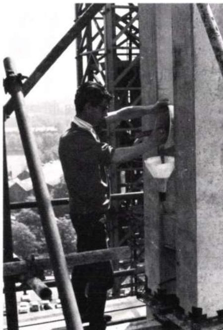
Fig. 11 Operative pouring Certite column joint (Photo: Keppie Henderson & Partners)
