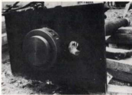
Fig. 3 Anchor plate for 1000 tonne tension in external columns of main frame work. (Photo : Laurent Rousseau)
