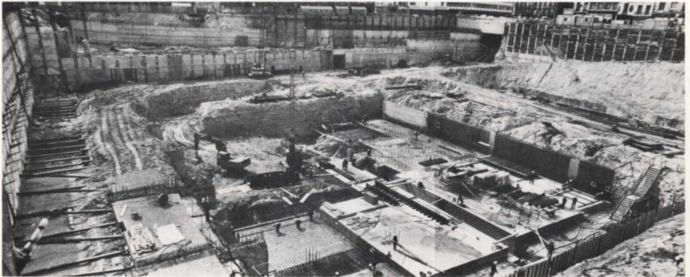
Fig. 4 Couvelage and buttress for toe of Berlinoise wall (Photo : Laurent Rousseau)
