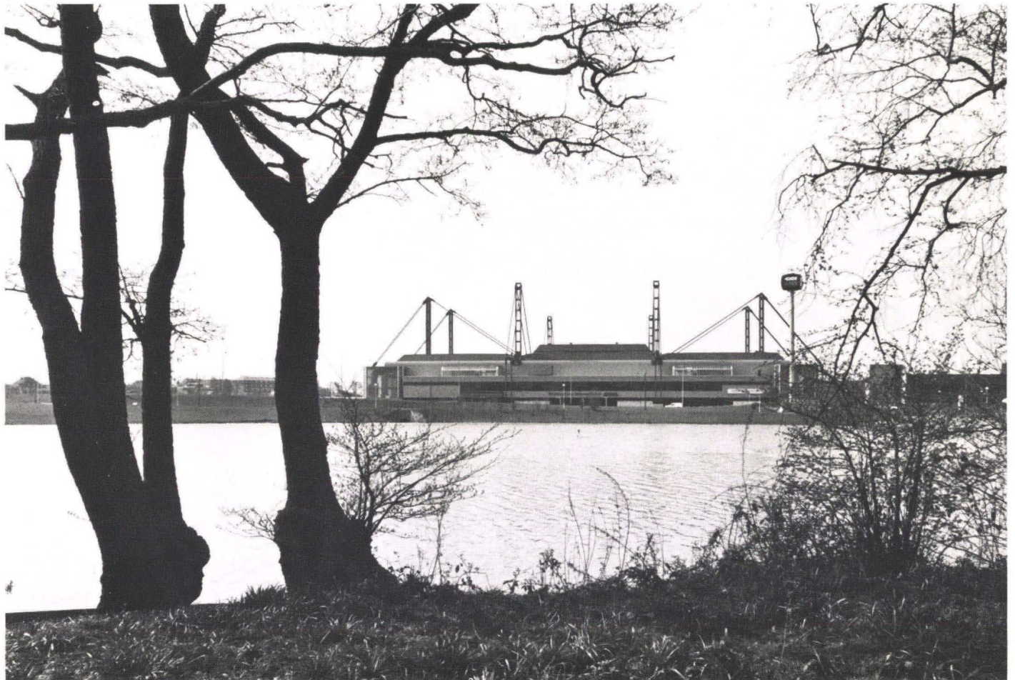
Fig. 1 Hall 7 from across the lake (Photo: Harry Sowden)
