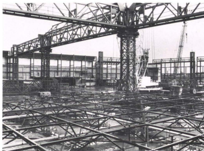
Fig. 6 Main hall under construction showing temporary support trestle (Photo: Harry Sowden)
