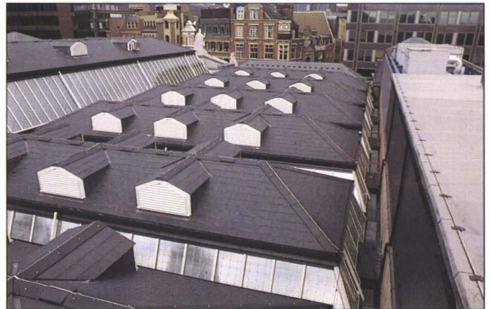
19. Roof showing cooling towers
