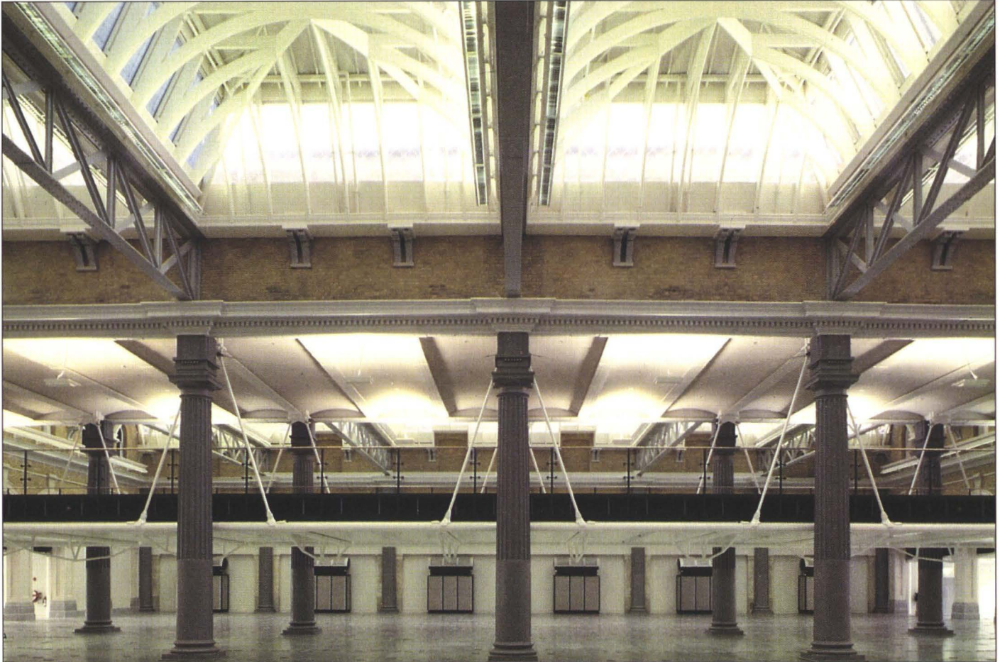
8. Interior showing new demountable mezzanine floor
