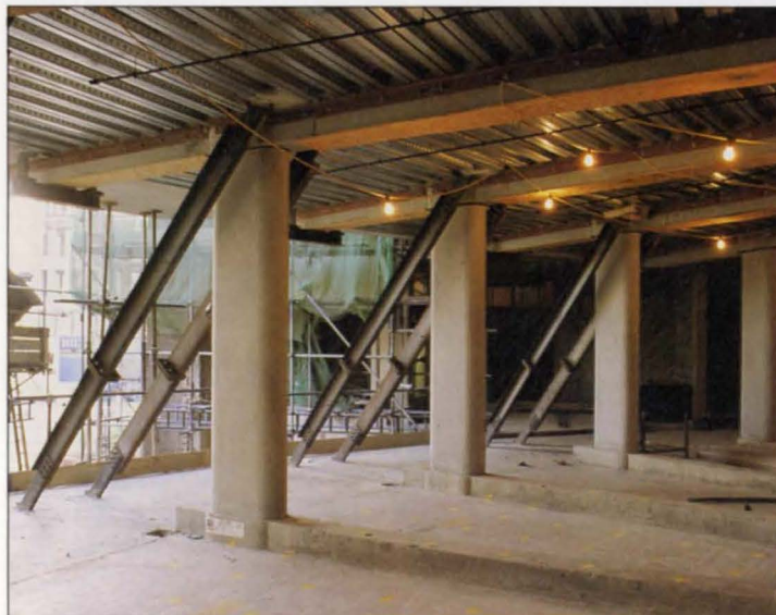
9. Quadrant showing circumferential route before laying of services.
