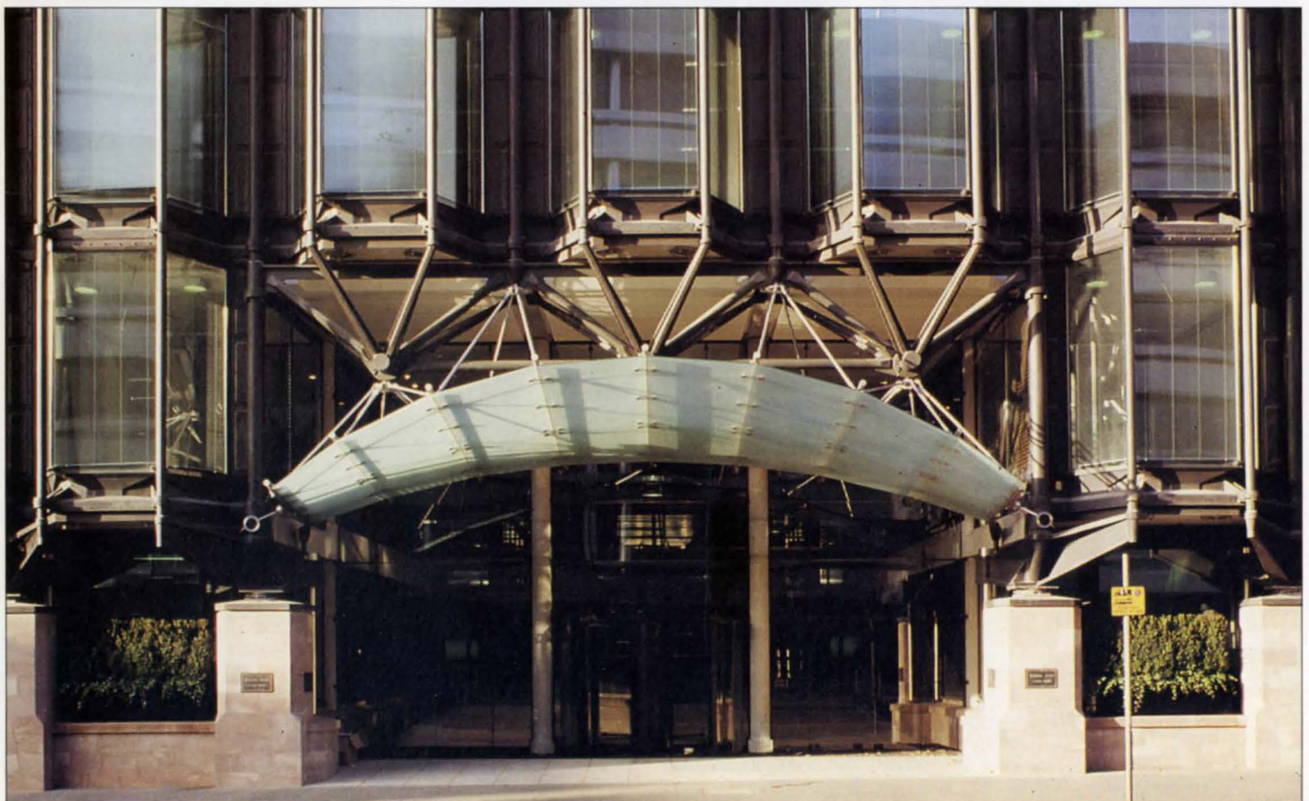
Below 3. New main entrance.
