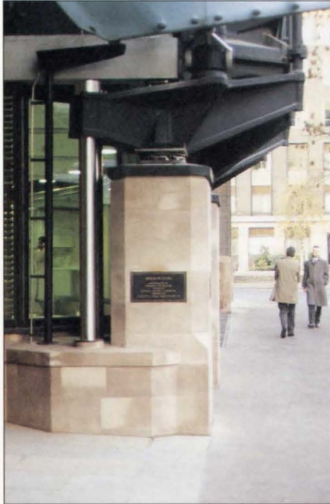
Left 14. Façade support bracket, with stainless steel tension rod on left and below 15. Gunmetal support bracket.
