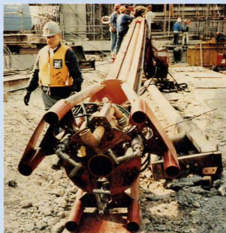
B. (below): Specially-developed hydraulic auger.
