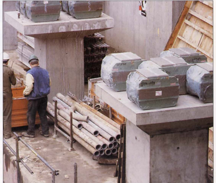
12. Acoustic isolation of new offices.
