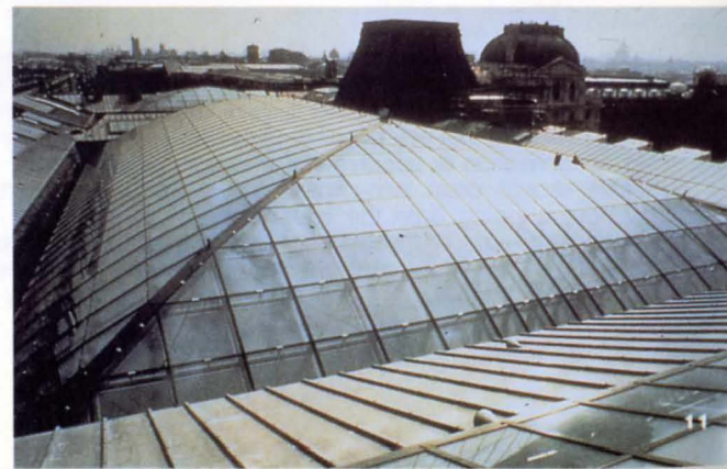
6. Roof of Cour Puget with Khorsabad roof in the background.
