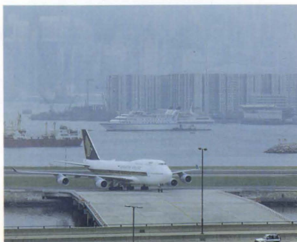
4. Aircraft taxiing onto bridge.
