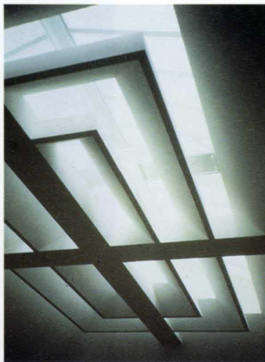
9. Typical square gallery: structural crossbeam supports light-directing plaster blades.
