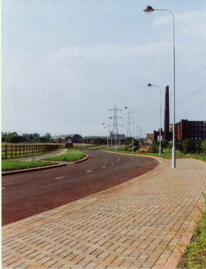
◀ 4. New road alongside canal, looking north, showing block footway construction.
