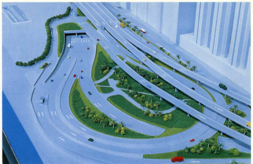
9. Part of model of grade-separated interchange between tunnel approaches and Route 7 (note tunnel portal in upper left of picture).
