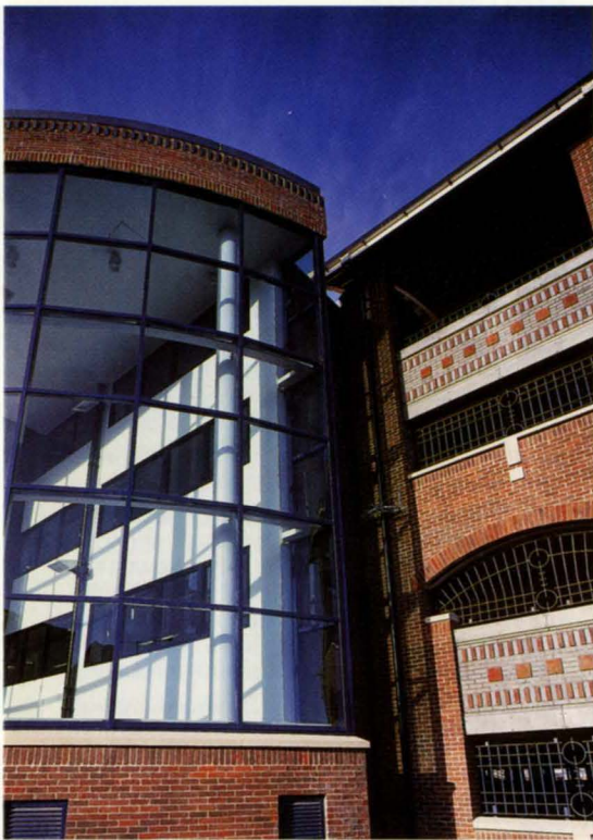
2. Stone dressed brick work detail, metal security grilles to the lower floors can be seen at right.
