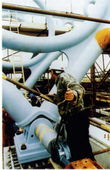
14. Inserting arch pin.
