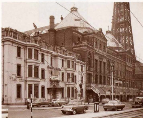
2. The original buildings c.1960.
