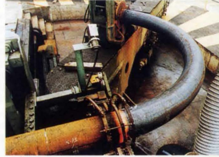
12. Induction bending in progress.
