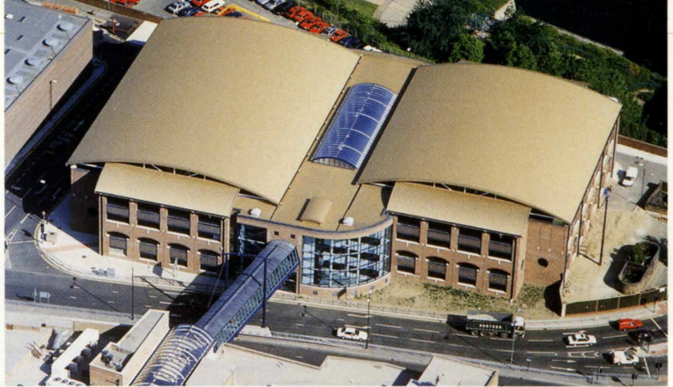
4. Aerial view: two metal-clad arched roofs span the parking areas, pedestrian bridge is in foreground.
