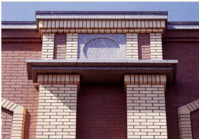
1. Brickwork detail on the refurbishment.
