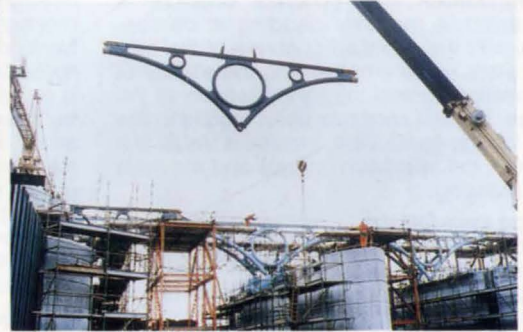
13. Arch erection.
