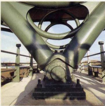
9. Detail of pinned arch supports.
