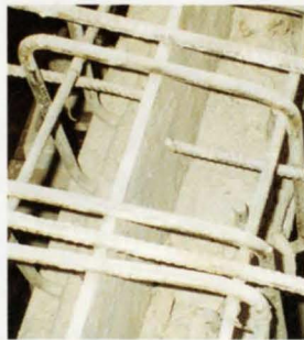
6. Close-up of original inverted T-beam.
