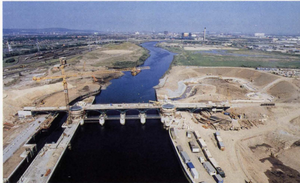
15. The bridge under construction: early 1994.
