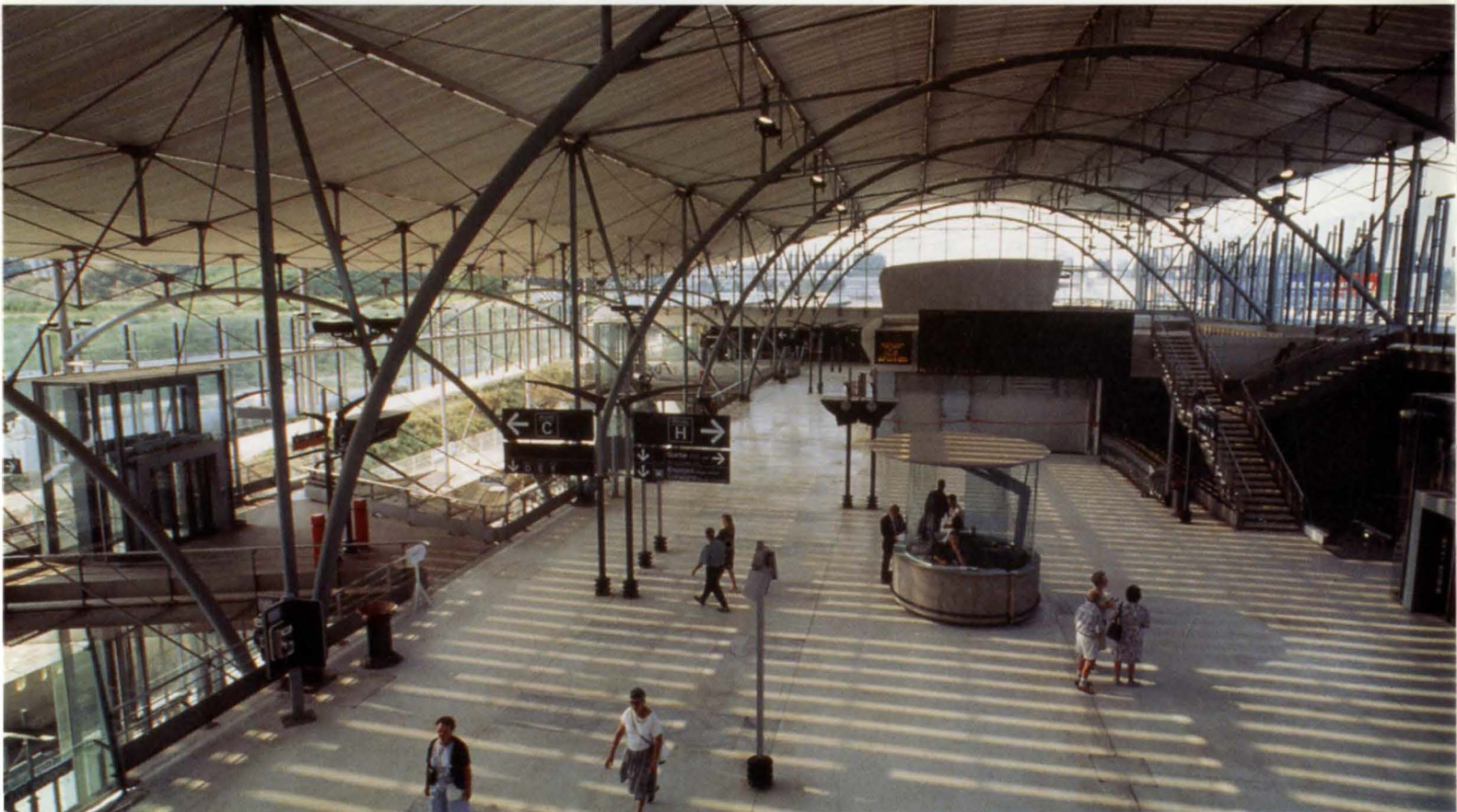
11. Interior of the station looking down on the main concourse.
