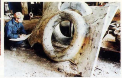
11. Casting condition survey.
