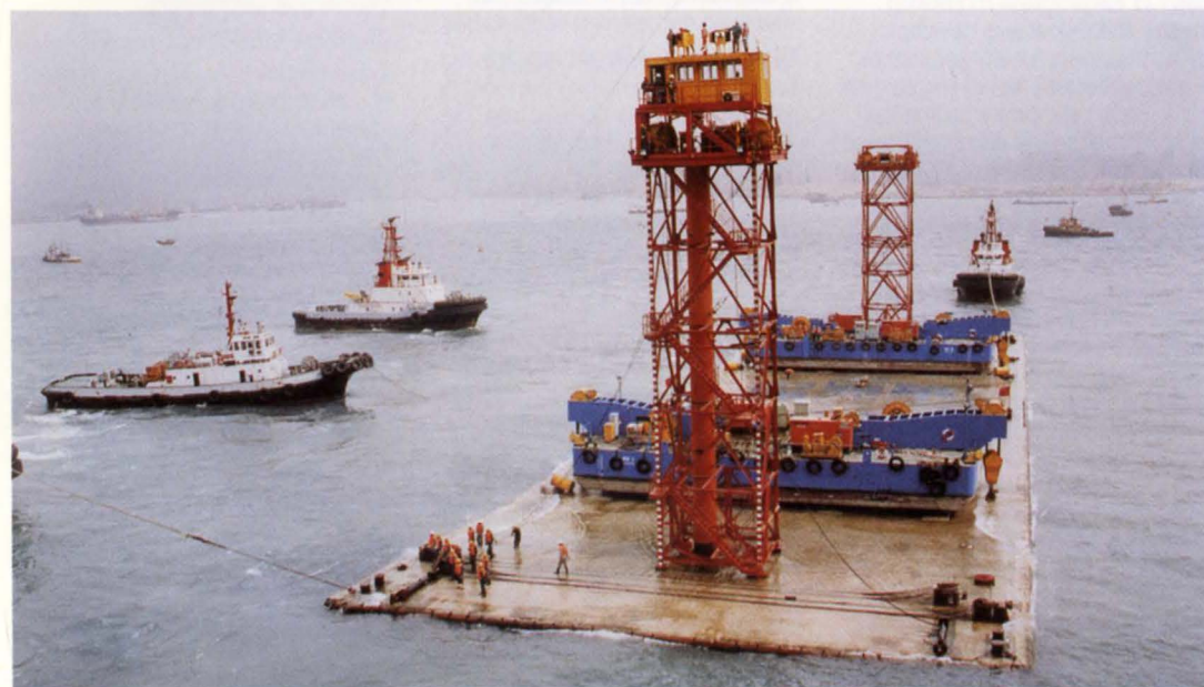
8. Tunnel unit 1 being floated into position at ventilation shaft (Hong Kong side), 15 March 1995.
