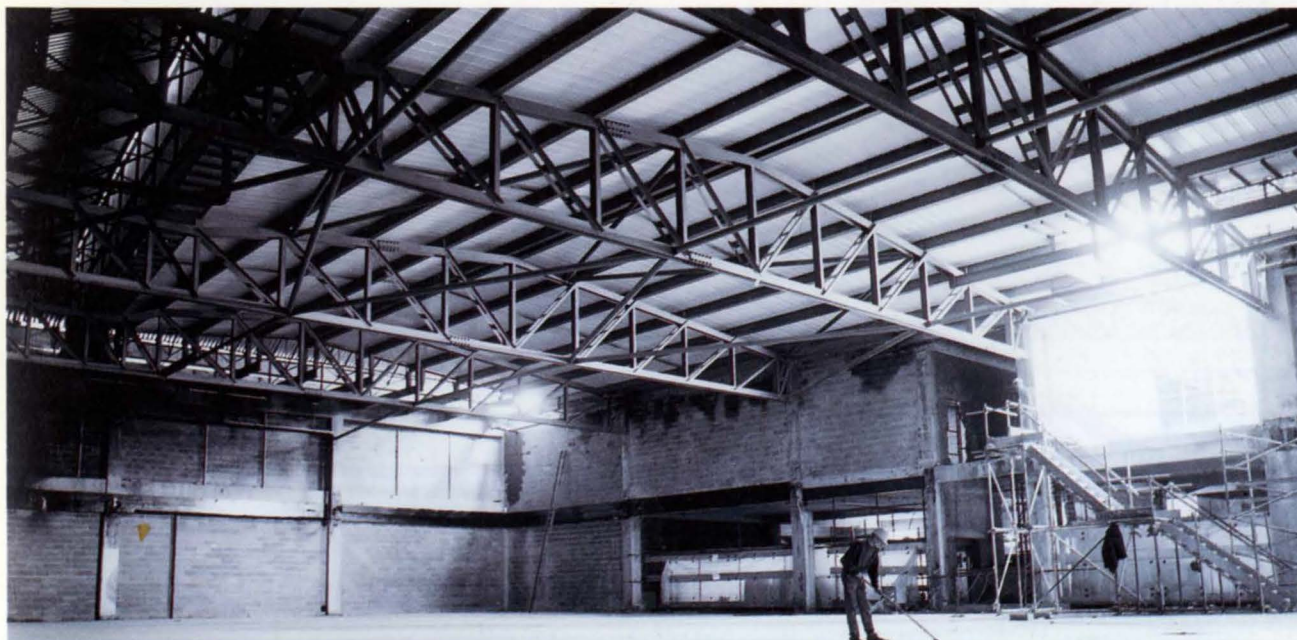
4. New two-storey void created at first floor level.
