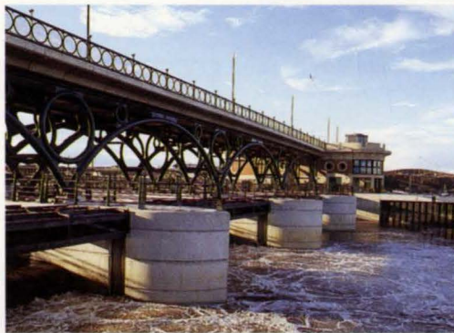
8. Concrete barrage piers.
