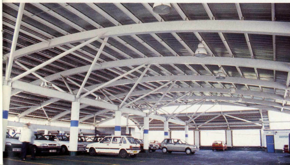
7. Parking bays: open plan floor provides uninterrupted views with minimal use of internal columns.
