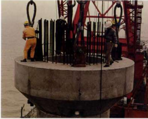
15. Attaching lifting frame to jetty caisson.
