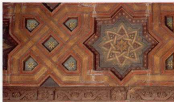
2. Reference Room painted cast plaster ceiling: pre-earthquake.
