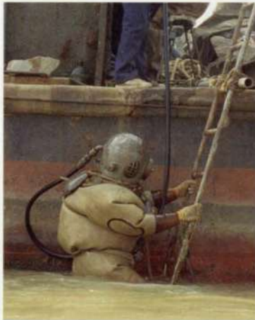
12. Diver placing levelling stone for caissons and culverts.
