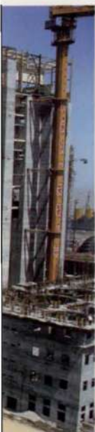
5. Slipforming unit 1 boiler and turbine hall, November 1993.
