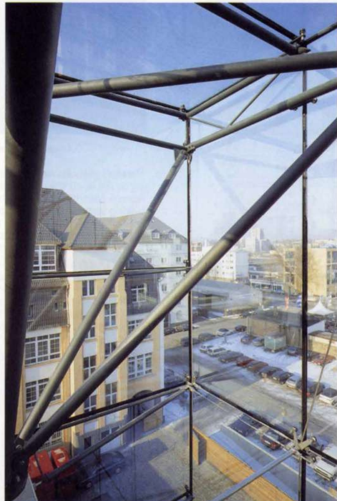
7. Testing the clamping detail.
