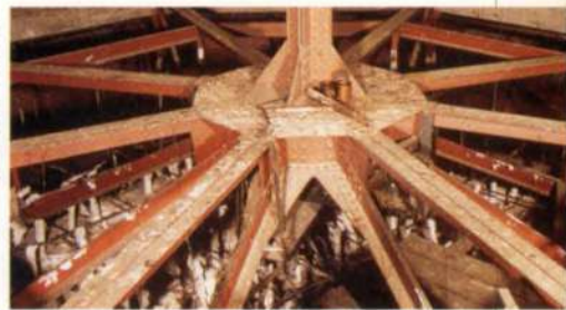
B. Plaster-coated hangers suspend ceiling panel from black iron frame and steel structure above.
