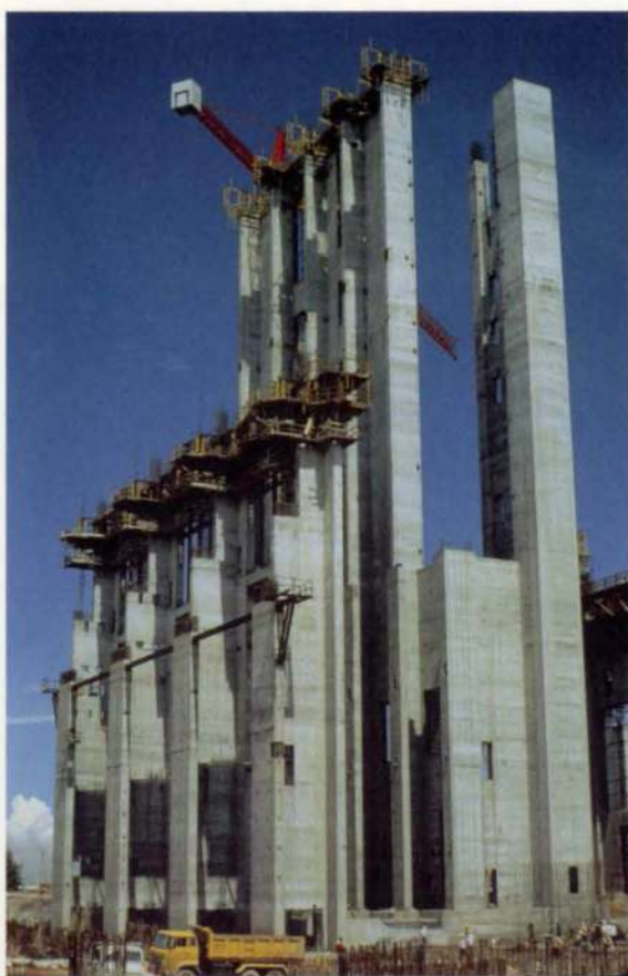
5. Slipforming unit 1 boiler and turbine hall, November 1993.
