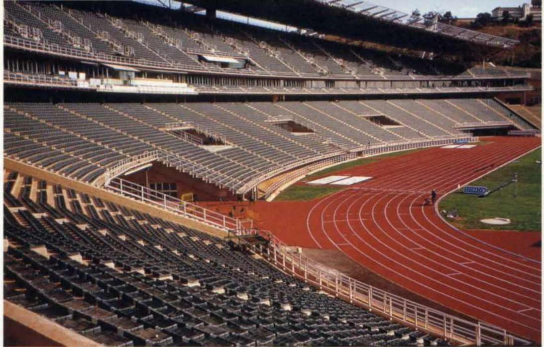
17. Completed interior of the stadium, showing wide pre- and post-event vomitories and (Left to right, mid-way up the lower bowl) the three dedicated terrace areas for media, VIPs, and officials.
