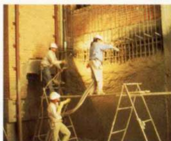
7. Shotcreting the Reference Room.
