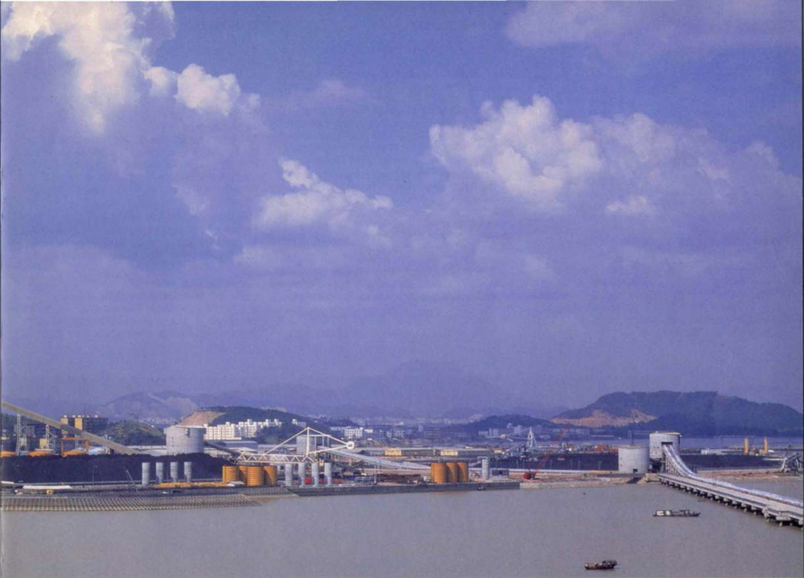
Shajiao B jetty access arm left foreground, Shajiao C jetty access arm extreme right.(photograph taken from Shajiao C jetty)
