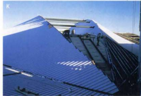
• Finally, the purlins, roof sheeting, and ceiling were installed (K).
