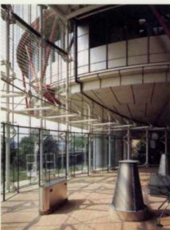
B. Bullet-proof screen, fan coil unit, and 'pepperpot' air diffuser in entrance hall.
