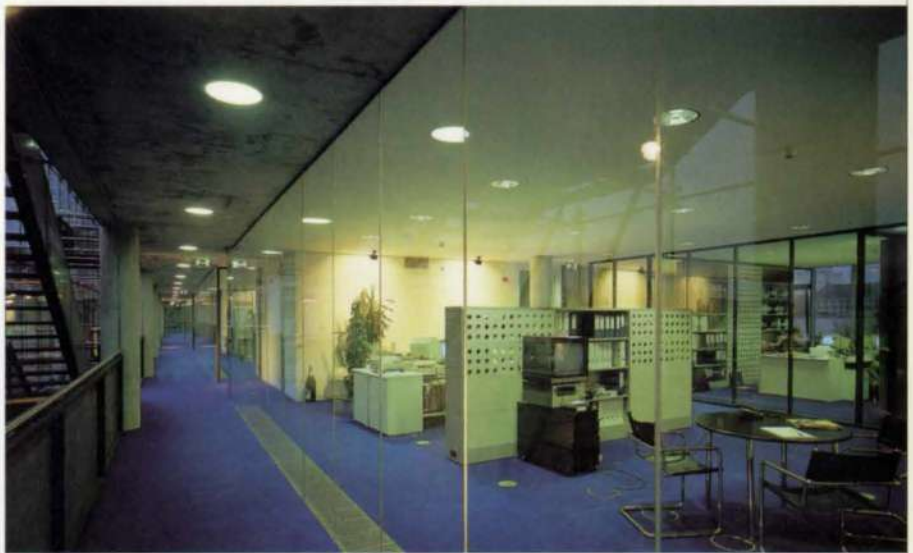
C. Office interior, showing single-glazed partition and supply air floor outlets.
