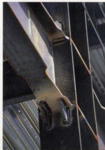
13. Outpatient clinic: moment connection after welding.
