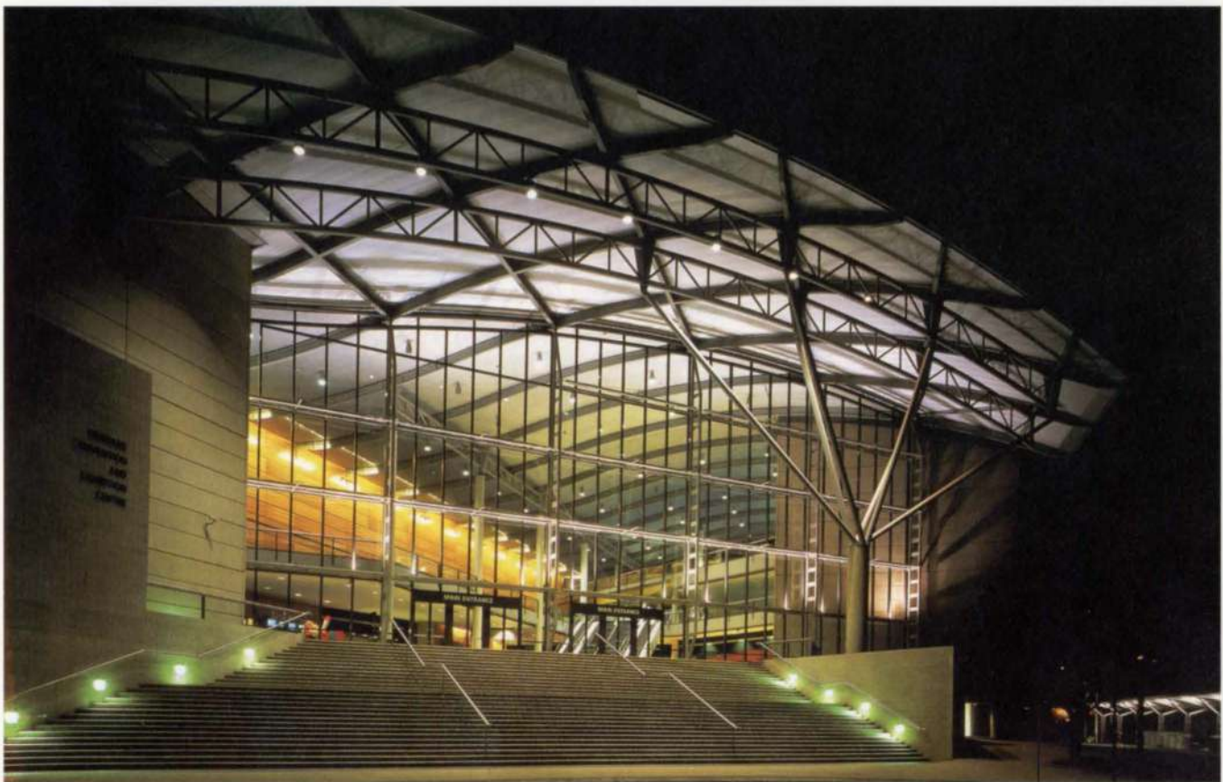
4. Main foyer entrance
