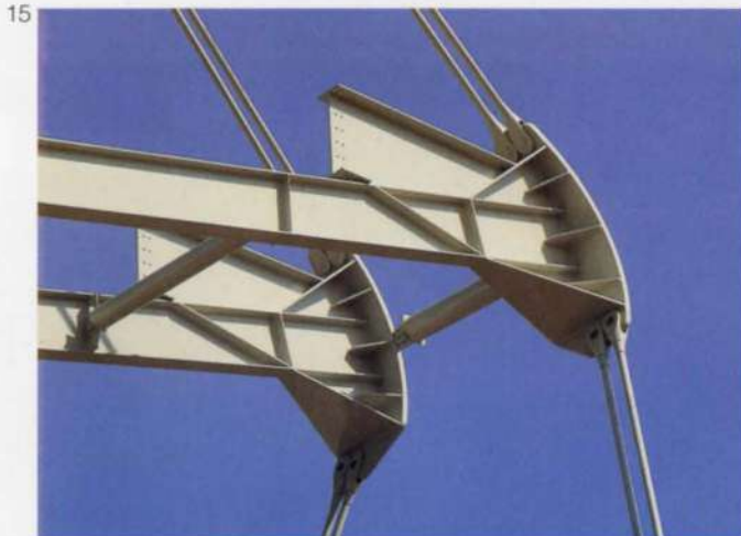
15, 16. Bracing element and A-frame, as built.
