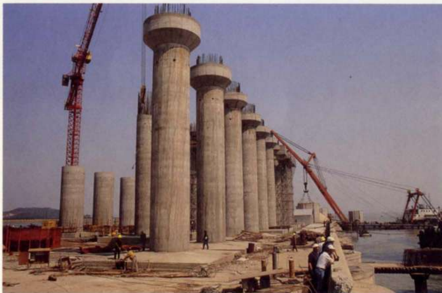
13. Slipformed jetty caissons awaiting placement, March, 1994.
