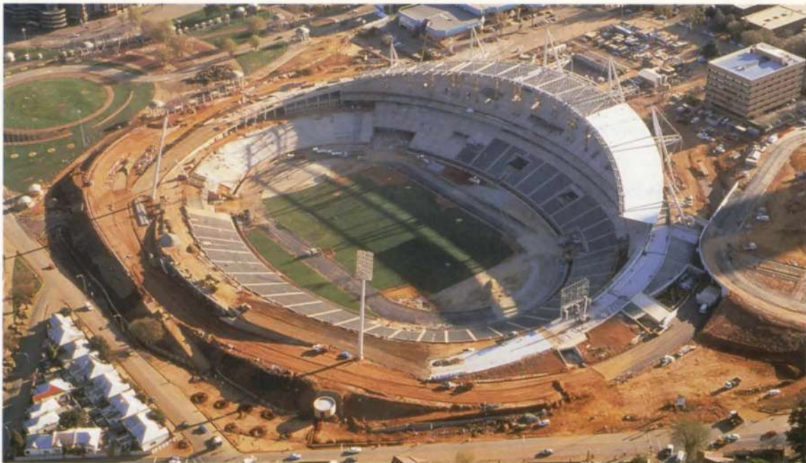
10. Site progress, October 1995.
