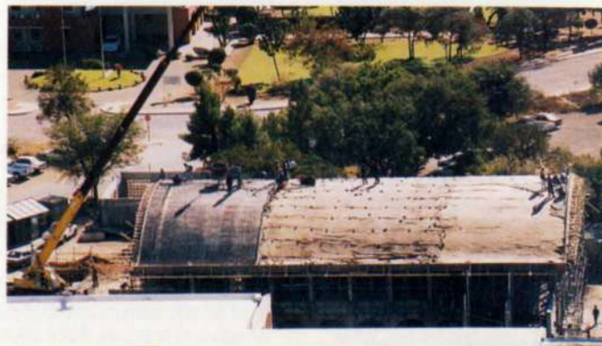
4. New building under construction.
