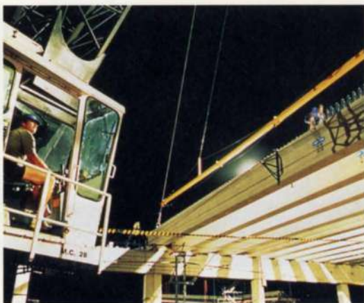
8 Left: 38m long precast, prestressed concrete girder being lifted into place above the inter-State railway. Note the steel bracing required to maintain stability of the girder whilst being lifted.
