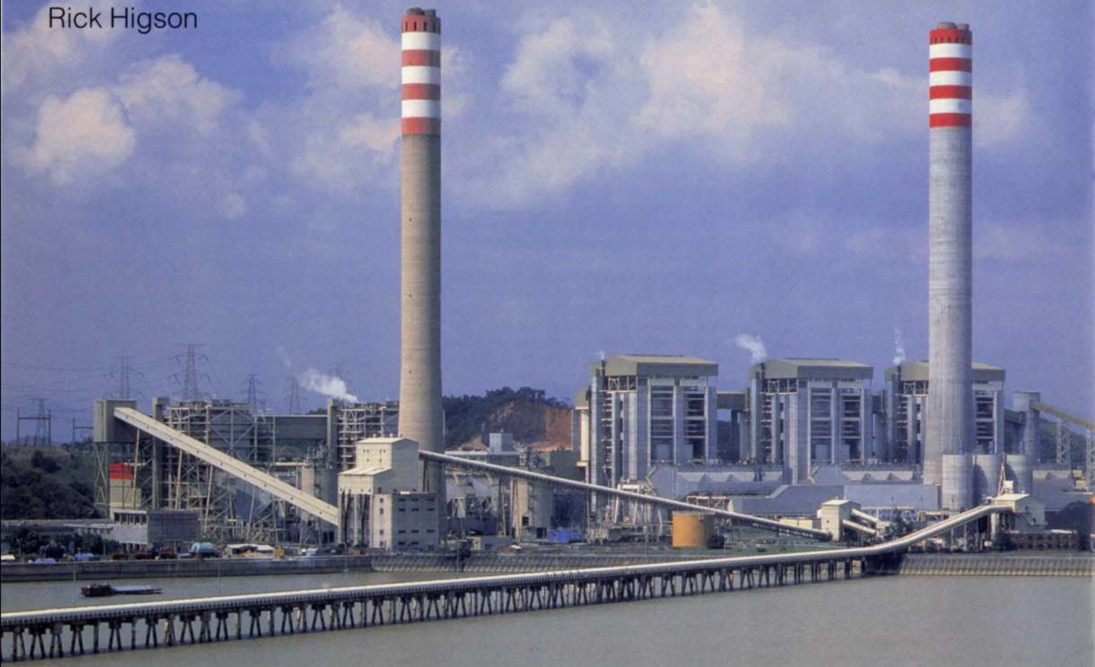
1. Left to right: the two 350MW units and 210m chimney of Shajiao B, and three 660MW units and 240m chimney of Shajiao C;
