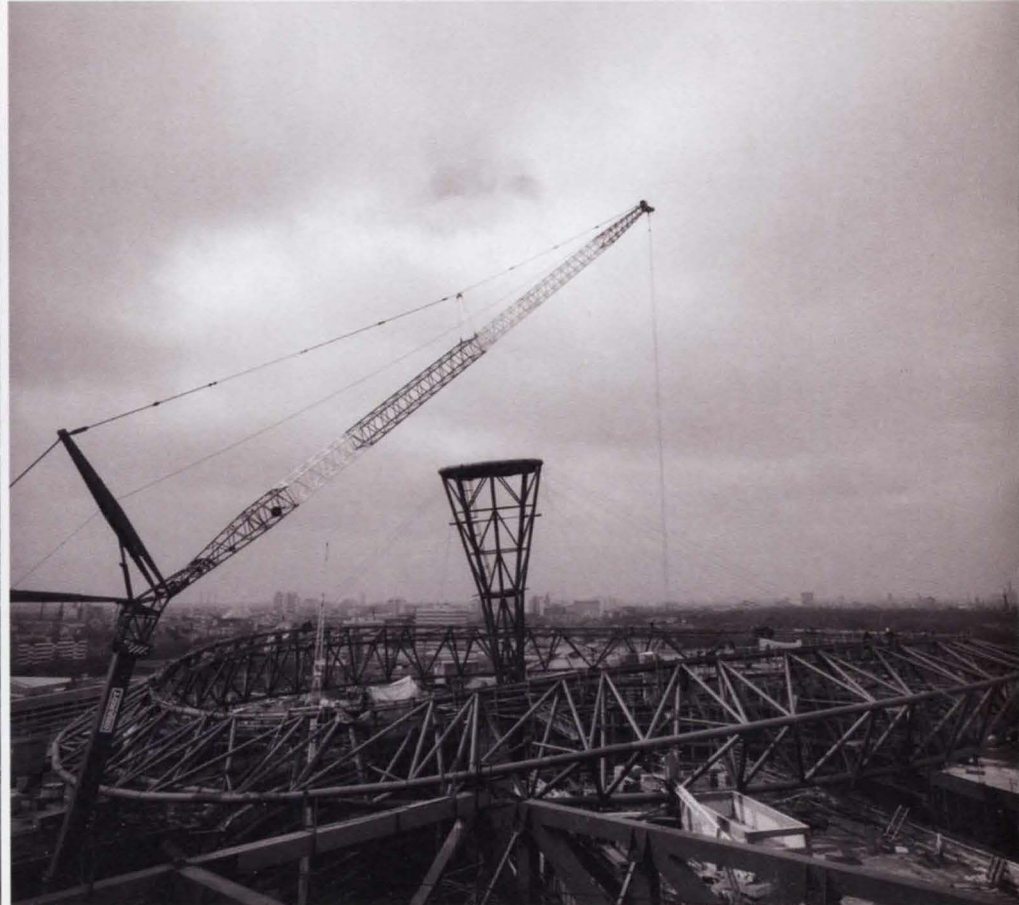
(c) Prefabricated kingpost supported in scaffolding.
