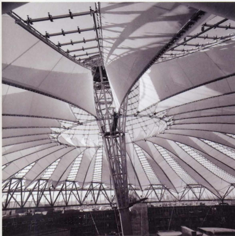
(j) Prestressed roof with free floating valley ring.
