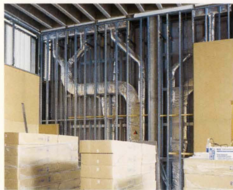
7. Air-conditioning ductwork being concealed behind thick walls.
