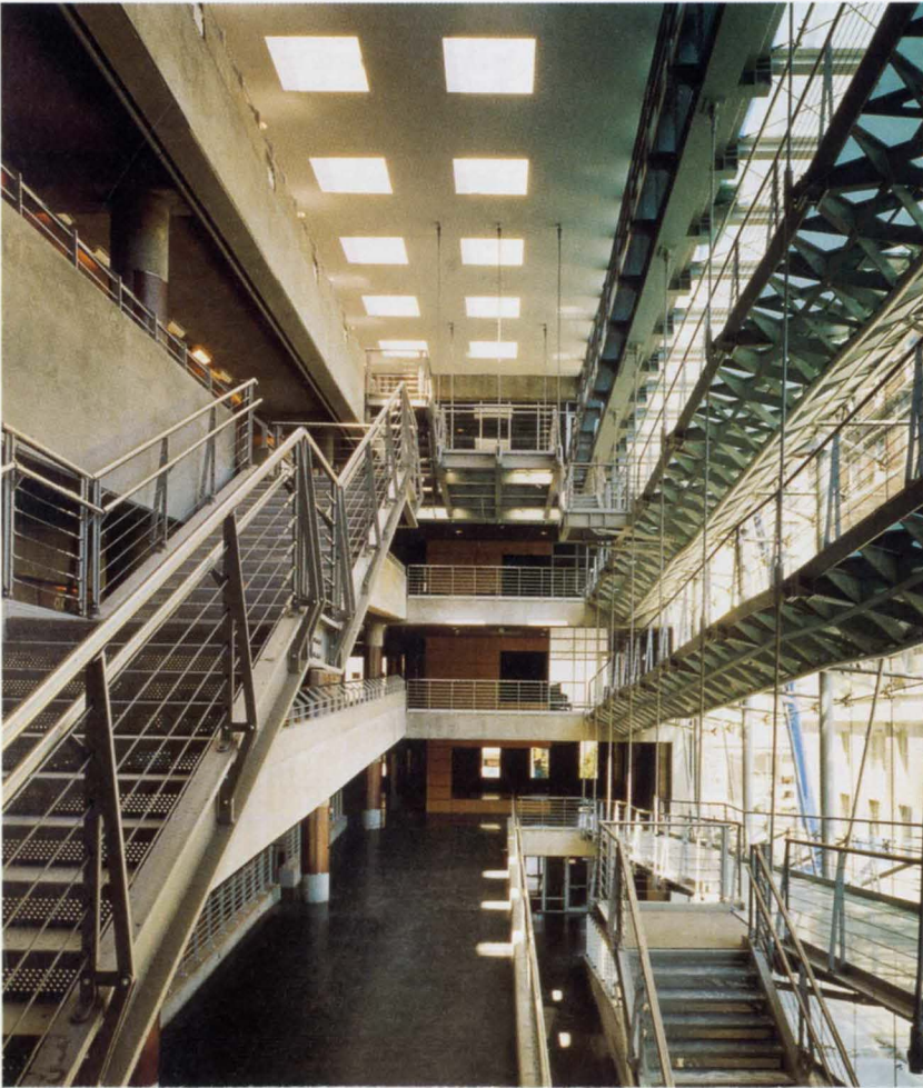
4. Internal view of glass wall ramps and stairs.
