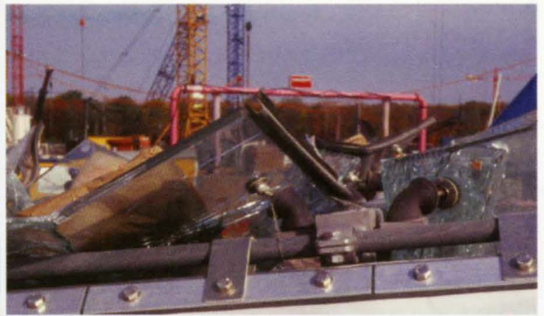
11 above: Broken laminated glass panel with 75kg/m 2 (16psf) loading.
