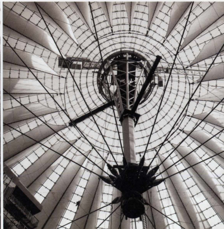
(i) Prestressing the roof by telescoping the kingpost (Jack force 15 000kN).
