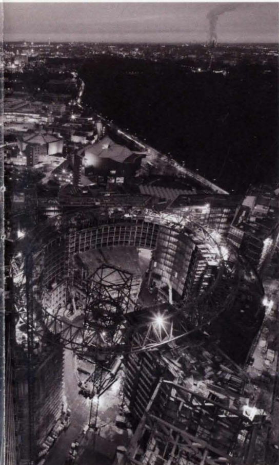
(a) to (k) Construction sequence of Forum Roof.
