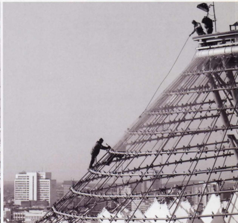
(k) Installation of the glazing.
