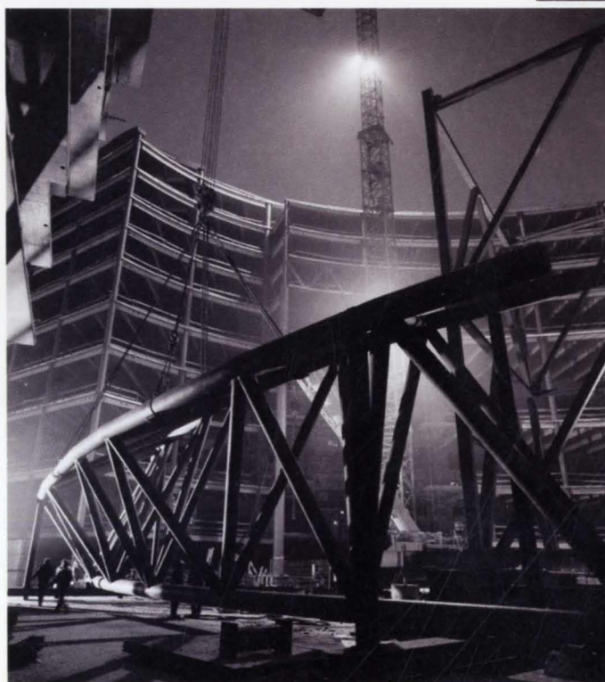
(a) Site-welded segment of the ringbeam ready for lifting.
