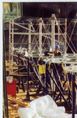
2 right: Beacon units prior to assembly
