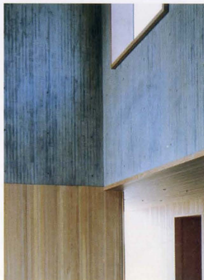
2. Timber cladding with boardmarking above.
