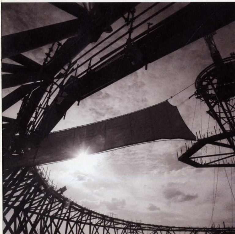
(d) Fabric segments being craned into position.
