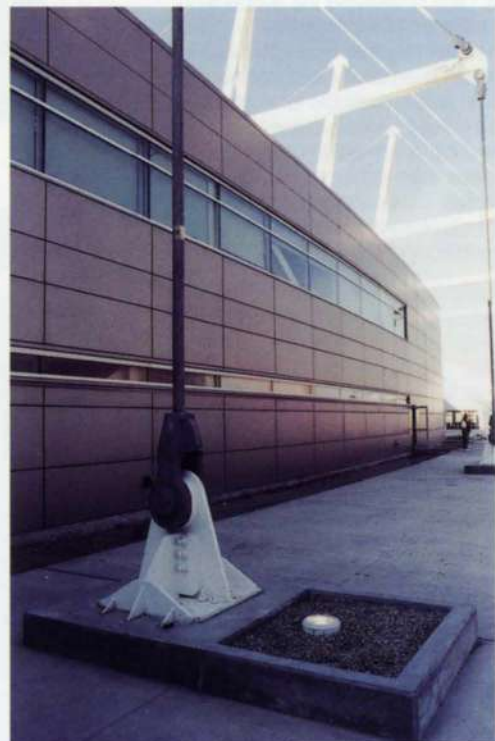
8. Tie down connection detail.
