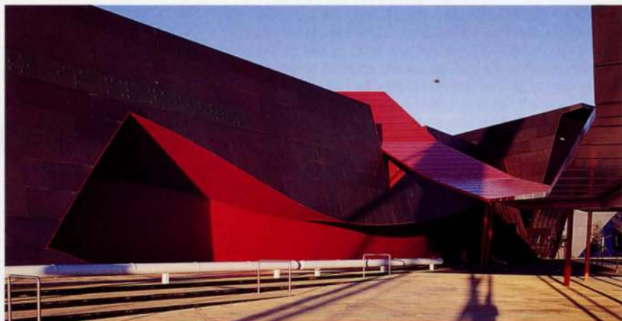
14. 'Loop' canopy and main entrance tunnel.
