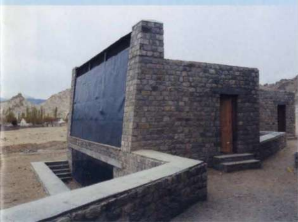
11. Completed solar-assisted VIP latrine.
