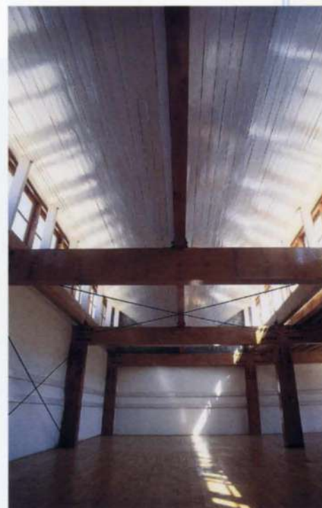
12. Timber structure to roof of lower kindergarten, optimising daylight.
