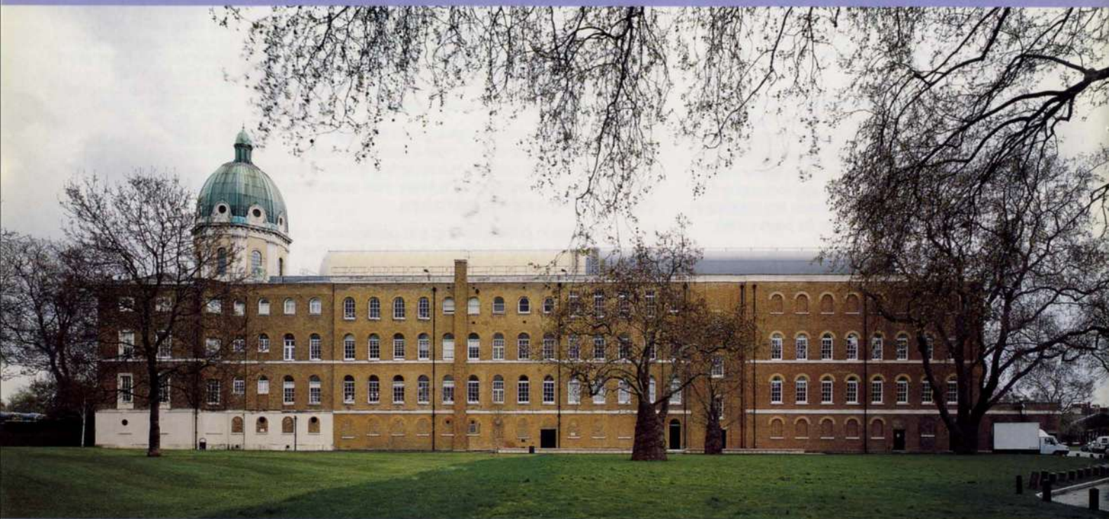
1. West façade of completed building.
