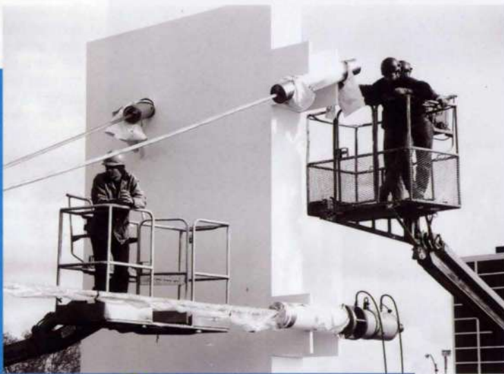
2 above: Schematic of arc and cable system. 3 left: The four cables converge at this common stainless steel connection at the free end of the arc: the long horizontal enters from the left; the three short cables exit from the right and attach to the tall steel pier. 4 right: Connectors to the steel pier. 5 below: Interior of the arc at dusk, showing cable connections to steel pier on the right.
