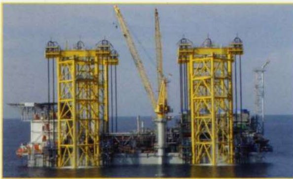
7. Pumping during installation of skirted base.
