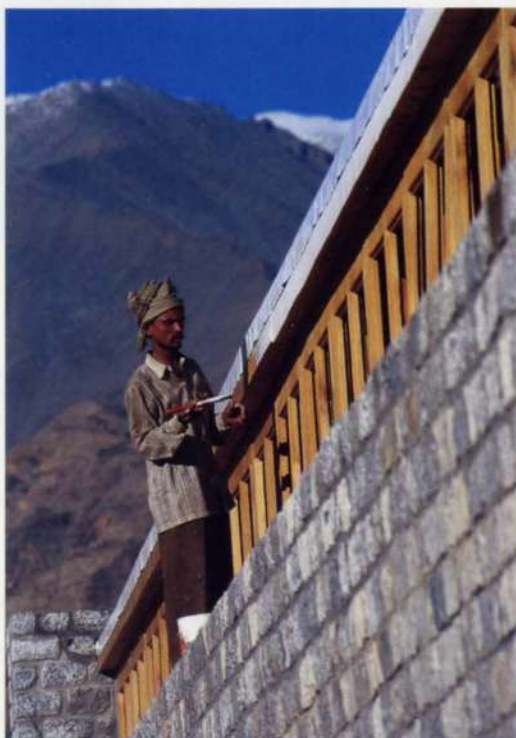
17. Painting the roof eave above timber-framed windows.
