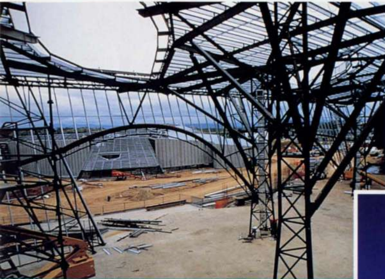
9. Main Hall steelwork. 10 right: Four-legged towers supporting the 'loop'.
