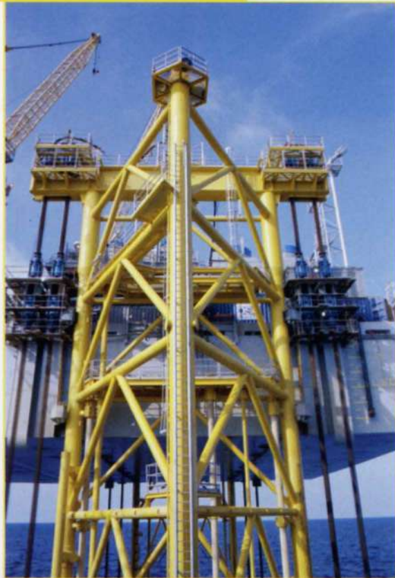
8. Deck raised to final elevation.
