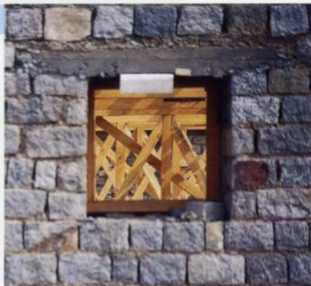
18. Local stone and timber: appropriate materials.
