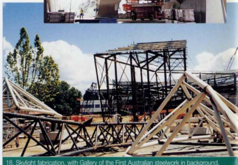
18. Skylight fabrication, with Gallery of the First Australian steelwork in background.
