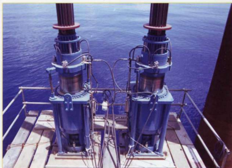
6. Base lowering jacks.
