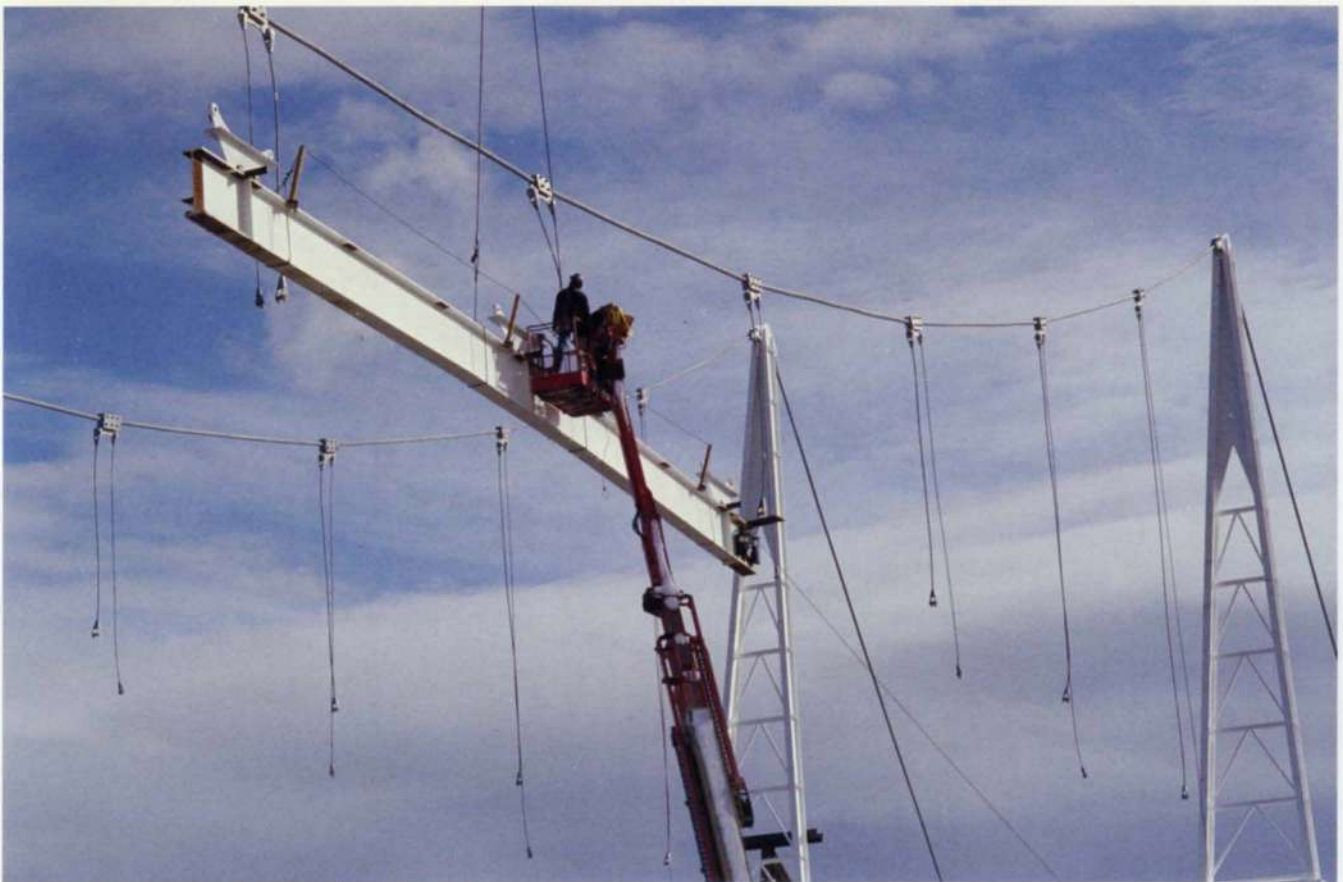
4. Hanging roof beam from the cable.
