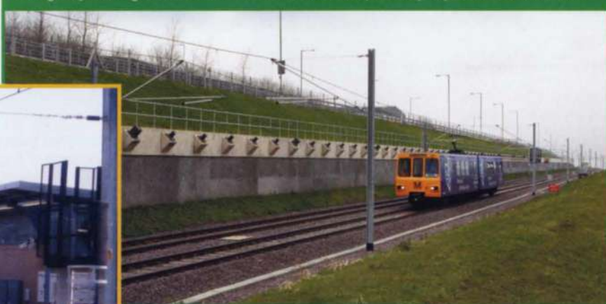
10. New highway retaining structure and rail infrastructure at European Way, adjacent to Pallion Station.
