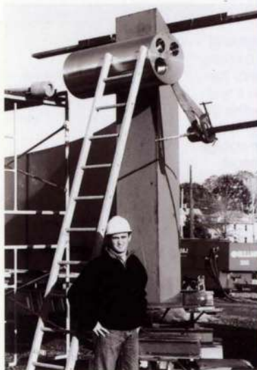
2 above: Schematic of arc and cable system. 3 left: The four cables converge at this common stainless steel connection at the free end of the arc: the long horizontal enters from the left; the three short cables exit from the right and attach to the tall steel pier. 4 right: Connectors to the steel pier. 5 below: Interior of the arc at dusk, showing cable connections to steel pier on the right.
