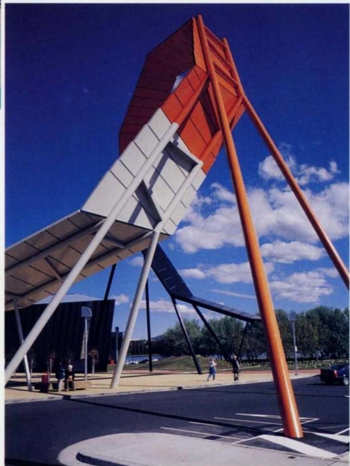
9. Main Hall steelwork. 10 right: Four-legged towers supporting the 'loop'.
