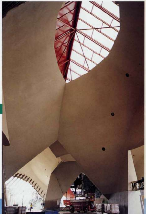
17. Skylight in the Main Hall.
