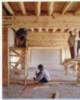
5. Construction in progress.
