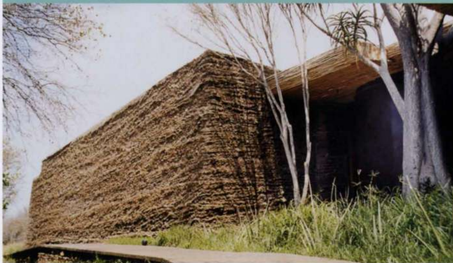
11. The completed compacted earth wall.
