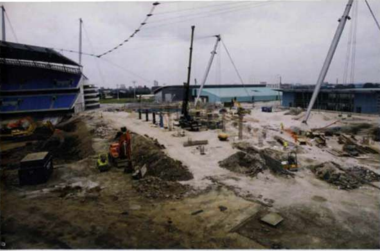
5. left: Removal of temporary seating, 2 September 2002.
