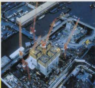
11a-d: Self-climbing core formwork construction sequence.
