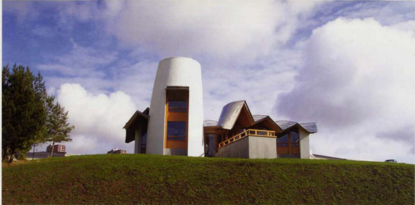
7. Facing the Tay estuary, showing raised viewing platform in front of the kitchen, alongside the tower.
