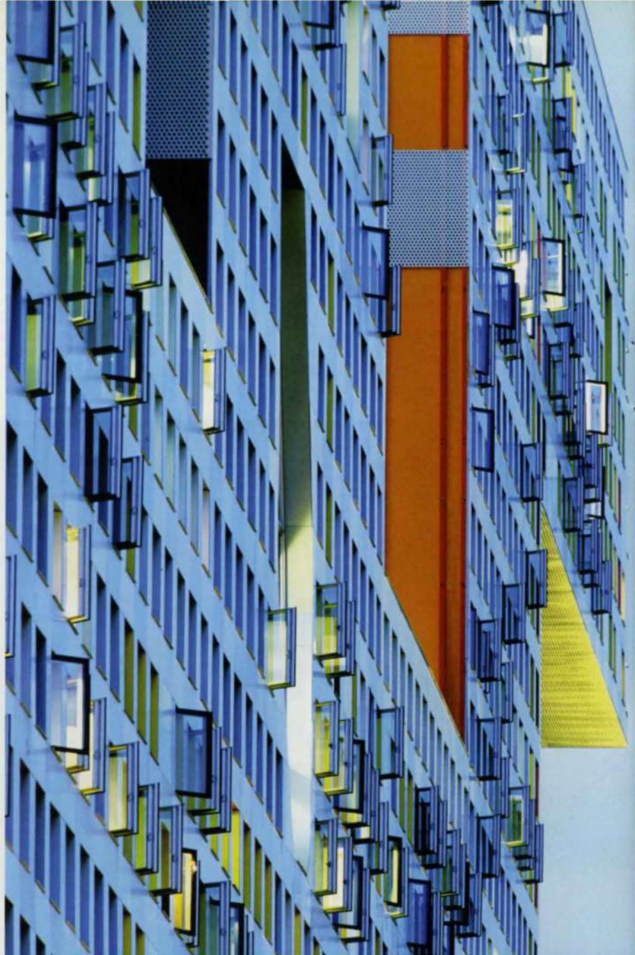
1. Close-up of the south façade, showing the operable windows in use by students in summer.
