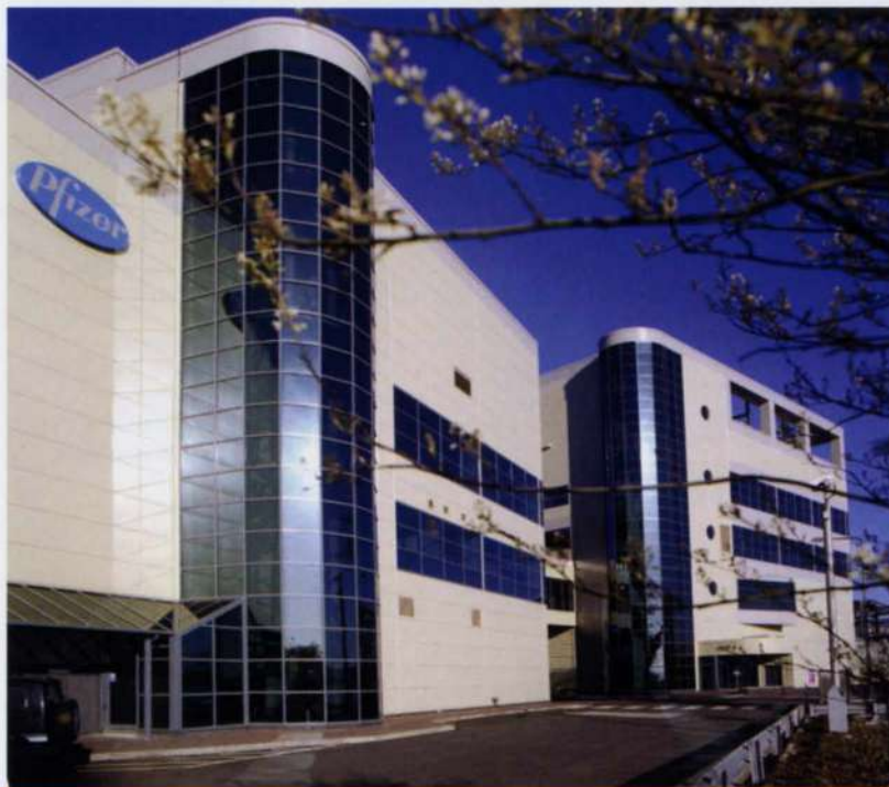
1. The finished goods building with the production building in the background.
