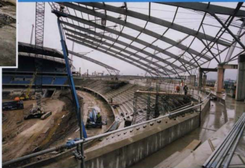
6. below: Progress on the North Stand, 21 January 2003.
