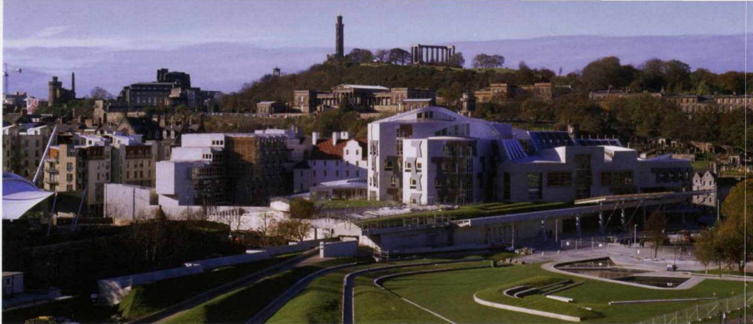
25. The SPB in its setting of new landscaping.
