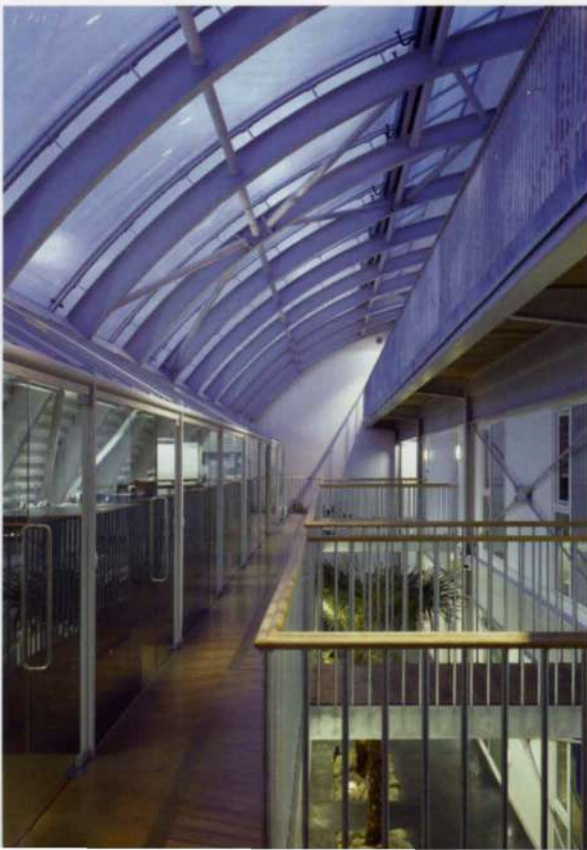
3. Upper level walkway and offices beneath skylights.
