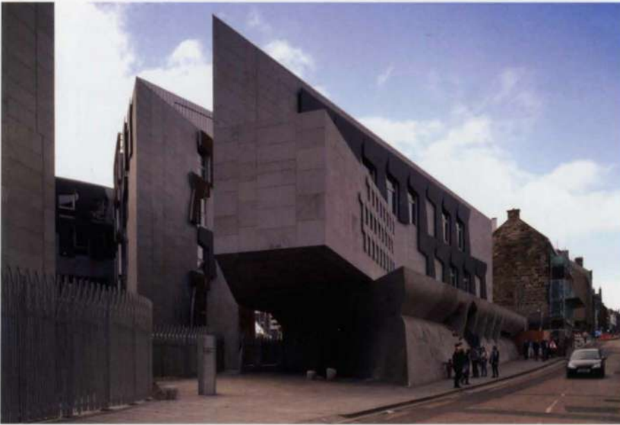
12. Entrance to the Canongate building showing the first floor cantilever and the Zen Garden.
