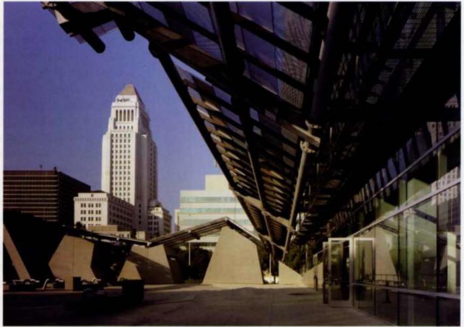
2. Plaza view from entry canopy looking north toward City Hall.
