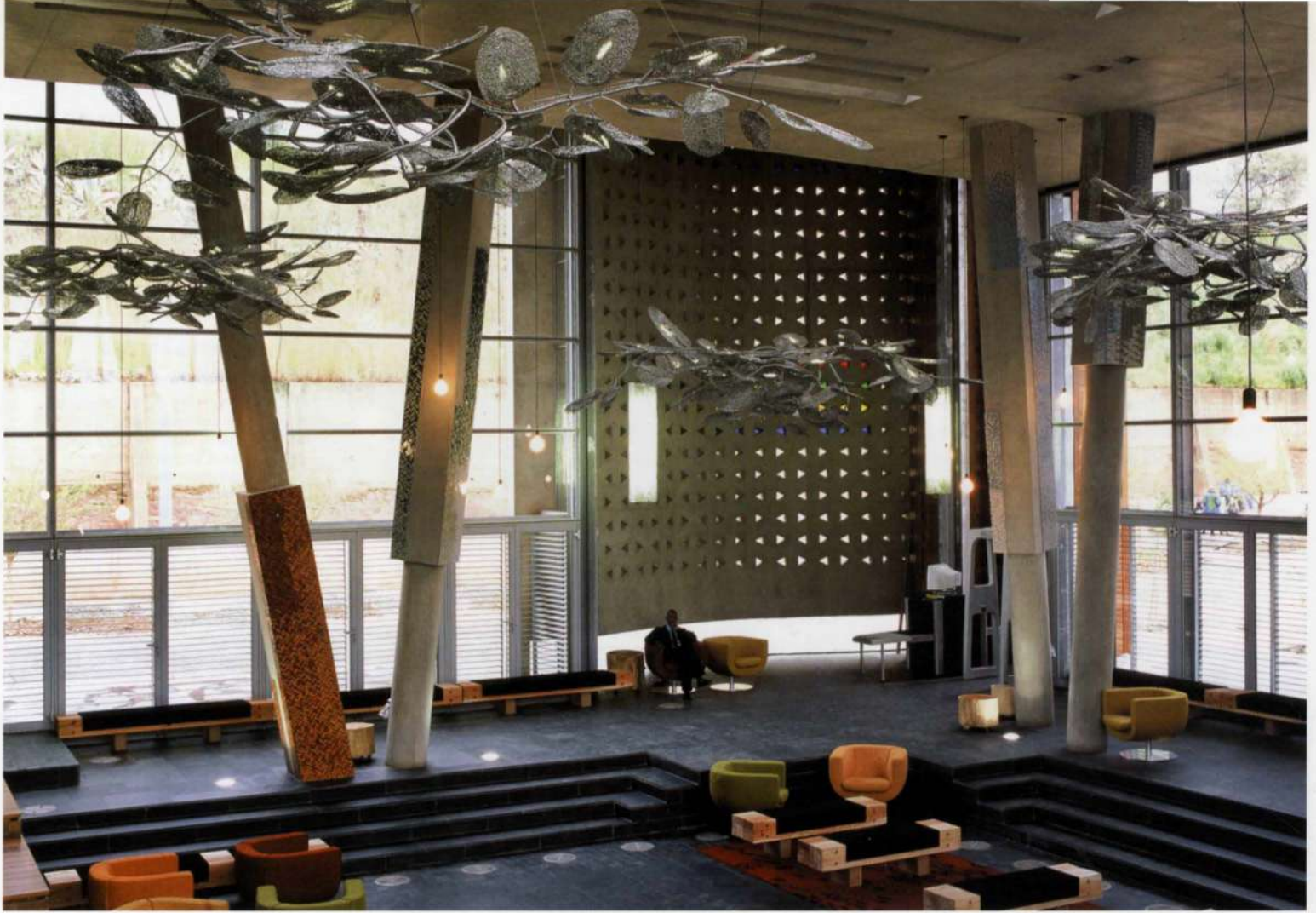
10. The entrance foyer to the Court, showing sloping columns, 'bar code' openings in the roof slab, and the curved concrete wall with triangular openings, all in off-shutter concrete.
