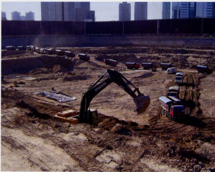
14. Site work begins, September 2004.
