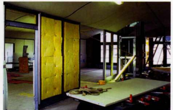
4. The Ofcom test installation: the dielectric cladding was polyethylene, the FSS substrate was polyester, and the core was extruded polystyrene.
