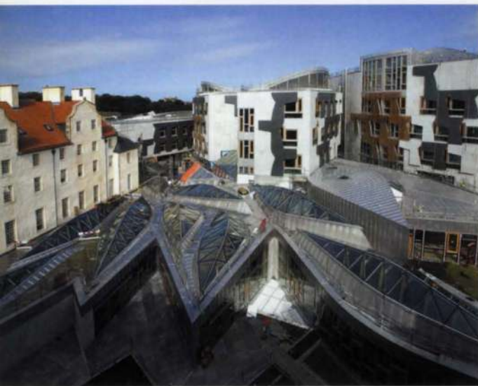
17. External view of foyer roof.
