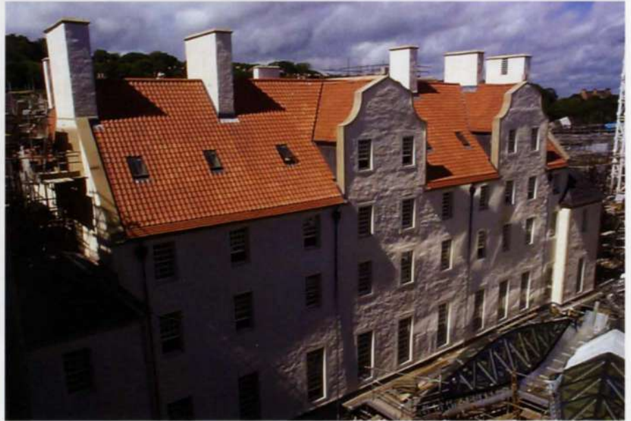
24. Queensberry House after refurbishment.
