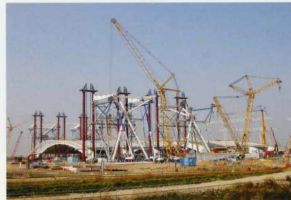
9. Roofing material in place prior to erection.
