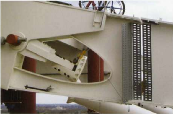
21. Adjustable connections.
