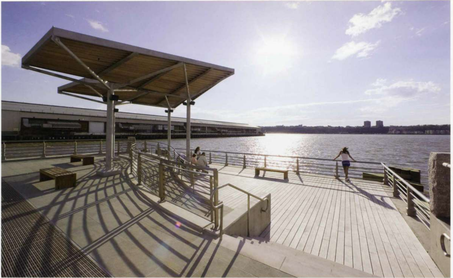
8. Pier 95 at Clinton Cove Park, Segment 7.
