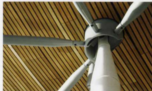
17. Roof column head.
