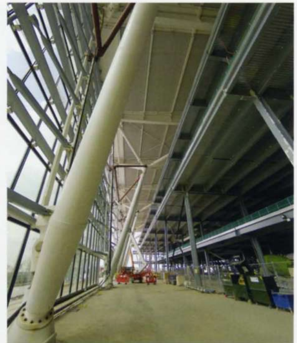
2. Dramatic full-height circulation space.
