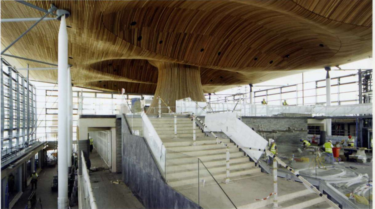
5. Canyon and public entrance under construction.
