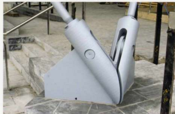
18. Ground anchorage of inclined roof tie.
