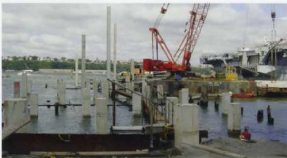
12. New hybrid precast prestressed piling for Pier 84, Segment 6, threaded amongst the remains of the old timber piles.
