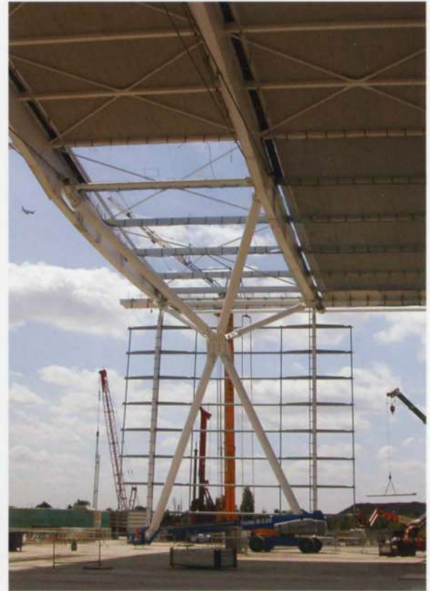
13. Bracing in roof plane and abutments.
