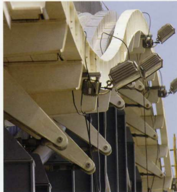
7. Joint at head of south façade.
