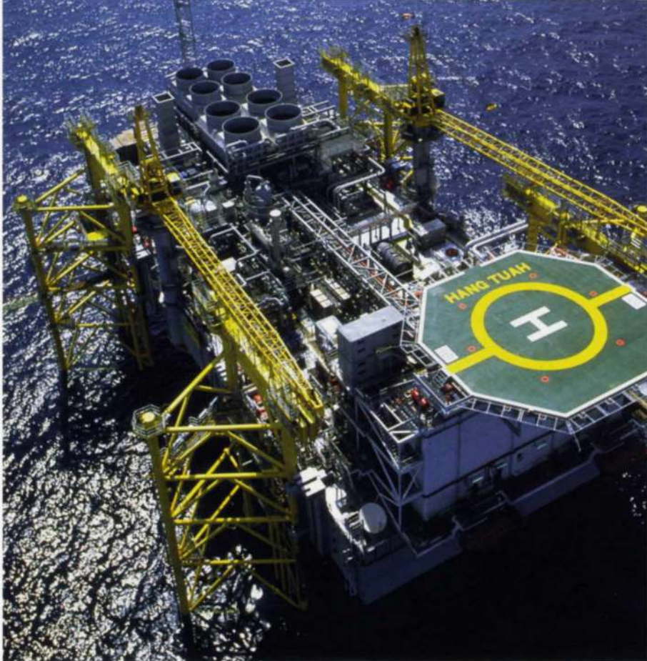
14. Arup Energy's ACE self-installing platform concept 15 operates as a movable offshore gas production unit, providing flexibility to develop scattered pockets of gas across 1600km 2 of the West Natuna Sea.
