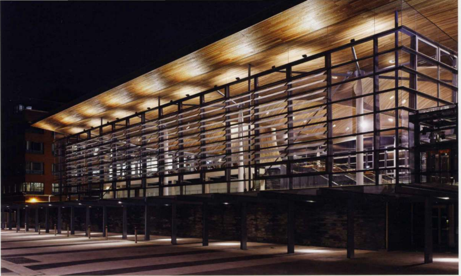
22. The glazed façade: side view at night.
