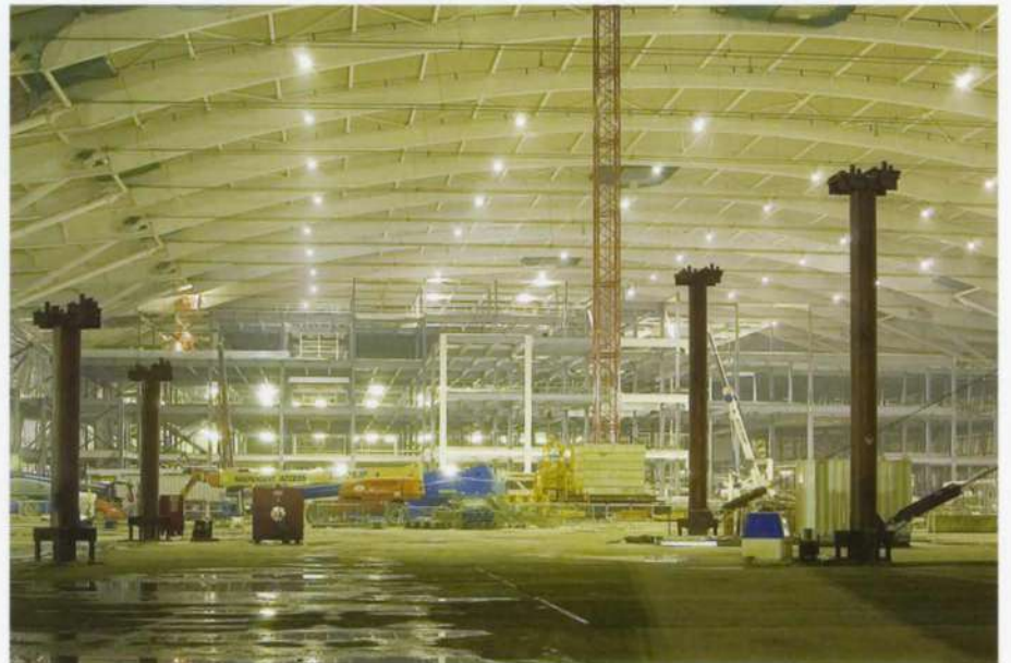
11. Central section clad and prestressed, May 2004.
