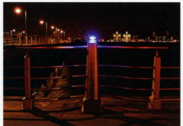
10. The Arup-designed coated stainless steel railings.
