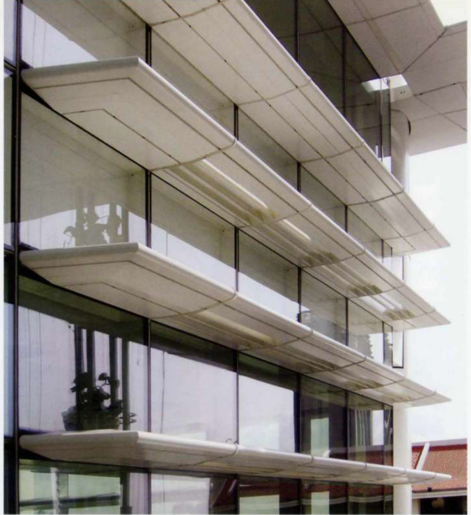
13. Exterior sunshades in place.
