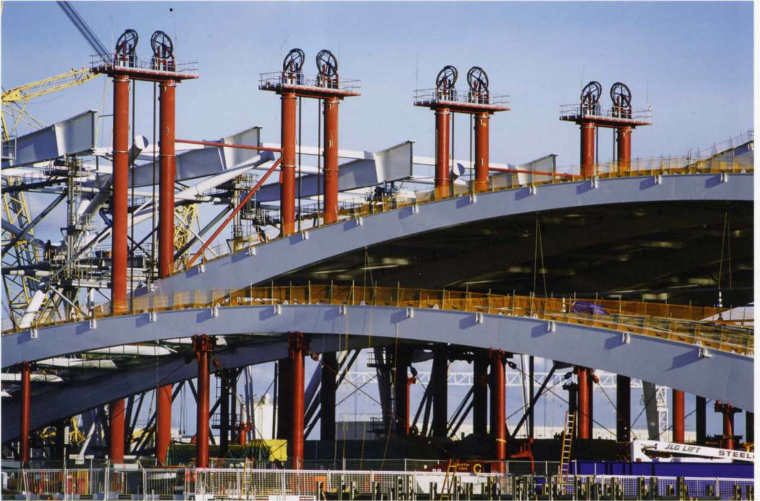
10. Jacking of roof elements.
