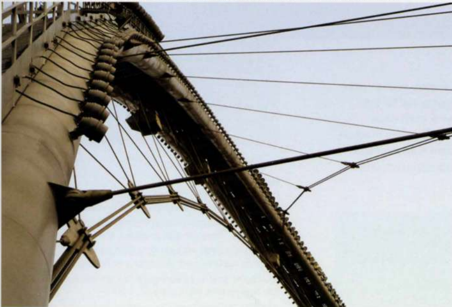
16. The lighting arch supports an array of sports lighting, as well as a loudspeaker array.
