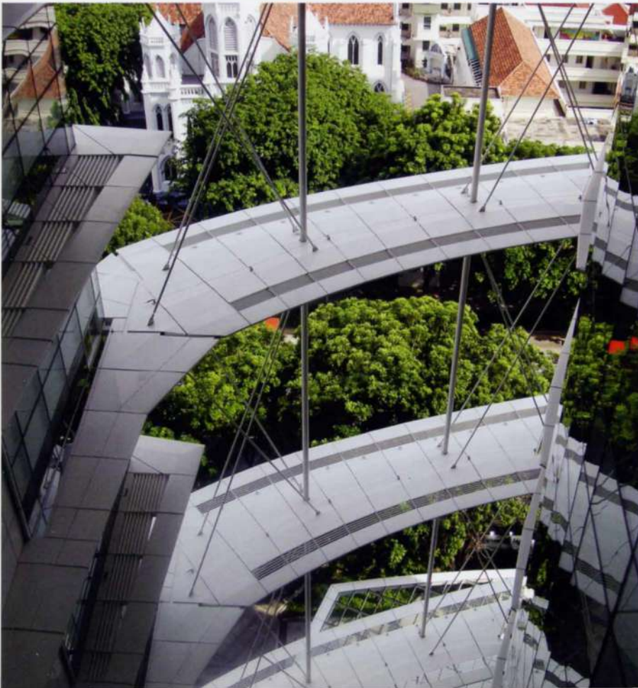
17. Sunshades in position in the laneway.
