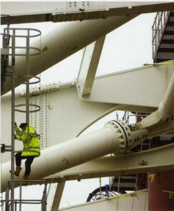
22. Conjunction of rafter with top of abutment frame.
