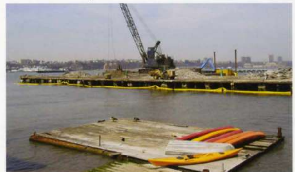
7. Pier 64 in Segment 5 cleared of its old shed.
