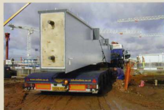
8. Rafter section arriving on site.
