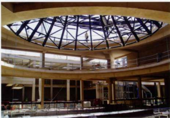
6. Underside of funnel, showing ring beams and cantilevers.
