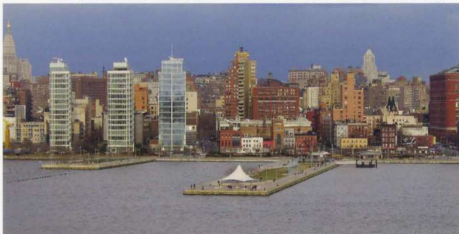
2. Piers 45 (right) and 46 in HRP's Segment 4, looking east against its Greenwich Village backdrop.
