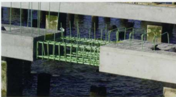
13. Precast pile caps at Pier 84, November 2004.
