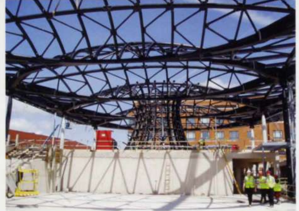
20. The roof under construction.
