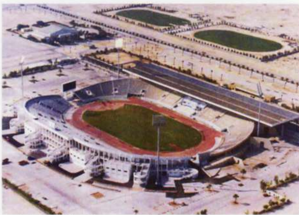
2. The stadium before upgrading.
