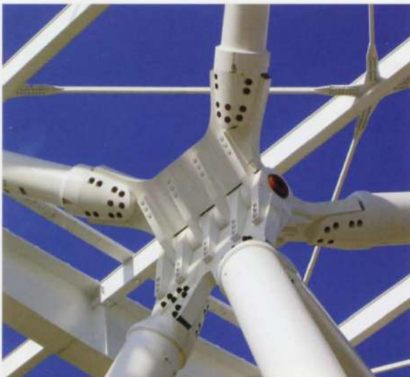
16. Connection of arm to torso.
