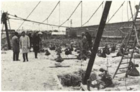
Fig. 2 The cable net with sandbags
