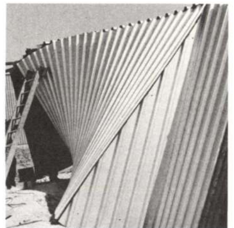
Fig. 10 Detail of the aluminium edge cladding
