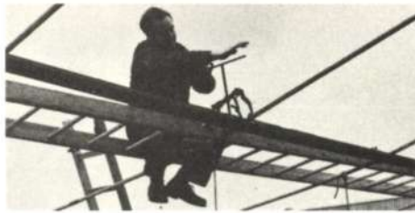
Fig. 3 Attaching the double angles
