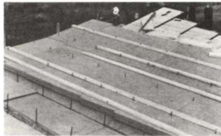
Fig. 5 Connecting the Sillan fibre glass panel
