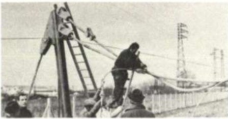
Fig. 1 Connecting cable to boundary cable
