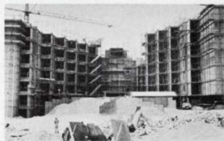
Fig. 9 Riyadh: back of service core (Photo: The contractors)
