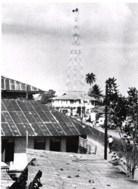
Fig. 12 Completed Heavy route tower
