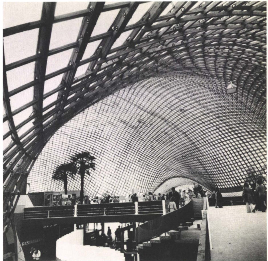
Fig. 6 Timber grid shell at Mannheim (Photo : Ove Arup & Partners)
