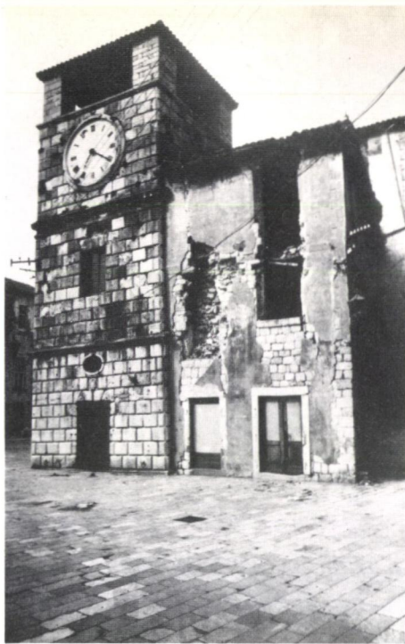
Fig. 7 Kotor: Clock tower nearly intact adjoining building badly damaged
