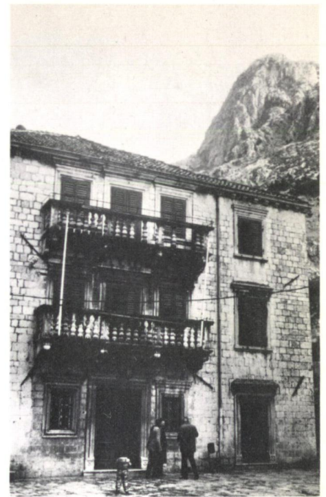
Fig. 5 Kotor: Maritime Museum Building, note tie rod anchors
