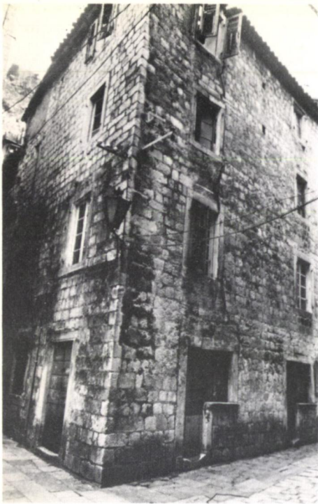
Fig. 6 Typical example of minor damage at Kotor
