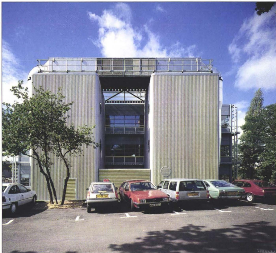
16. North side of the building showing pods, air-handling plant, ducts, and ground floor plantroom.
