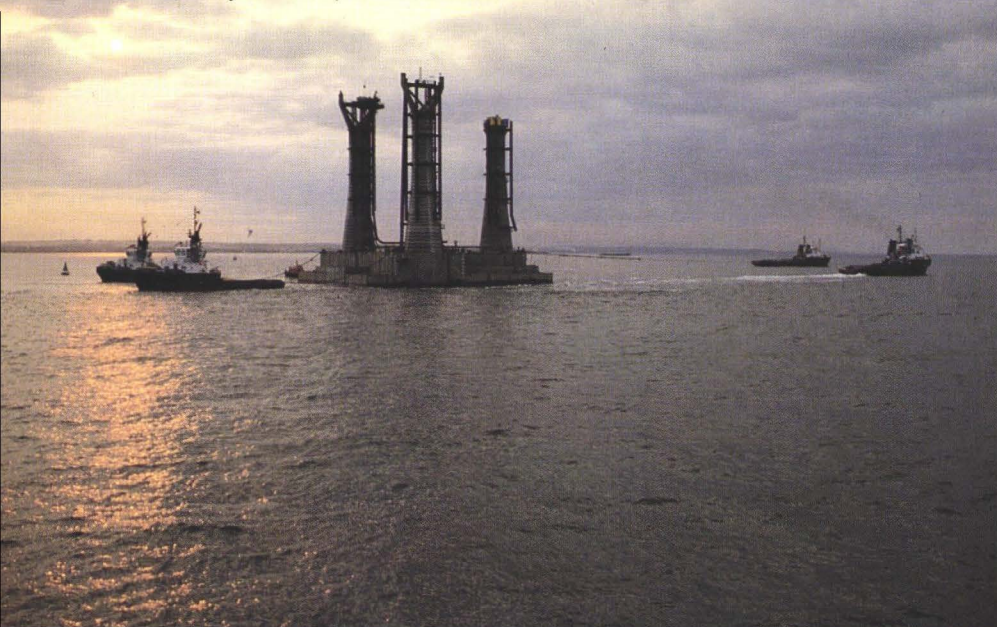
21. Offshore installation: start of flooding closed cells.
