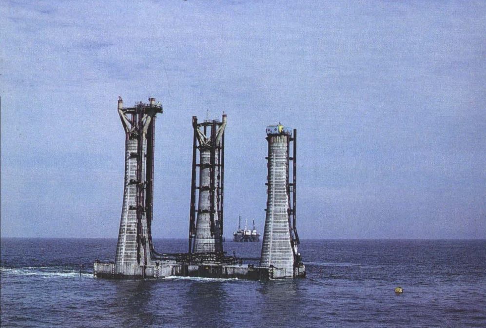
21. Offshore installation: start of flooding closed cells.
