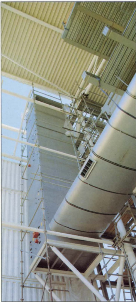
8. Left: Air-handling unit for envelope space feeding primary elliptical duct.
