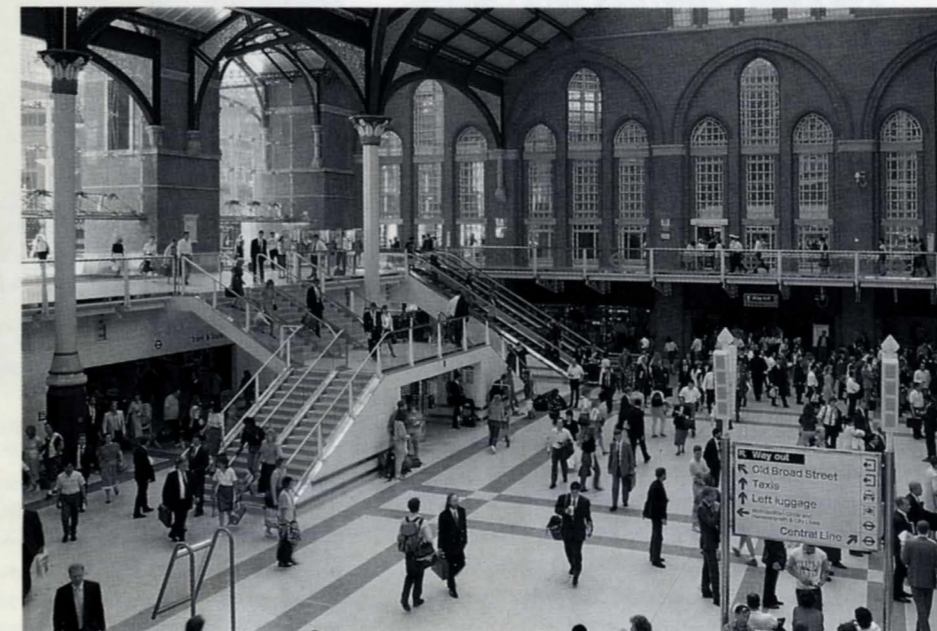
The Arup Transportation group designed the pedestrian circulation at Liverpool Street Station, London.
