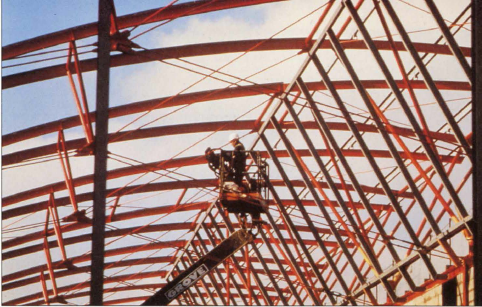
6. Installation of ties.
