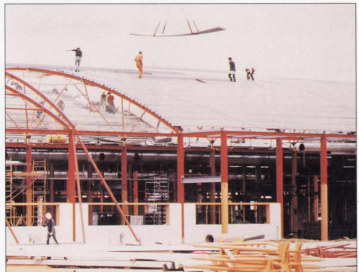
5. Right: Placing the inner cladding deck.
