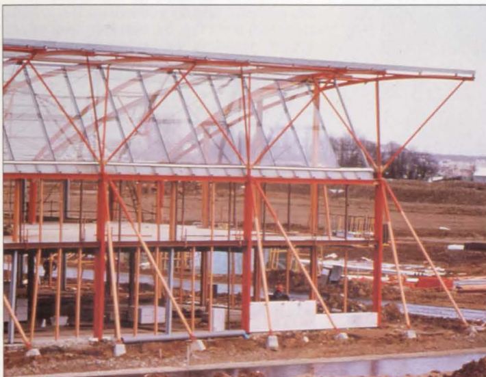
5. Right: Placing the inner cladding deck.
