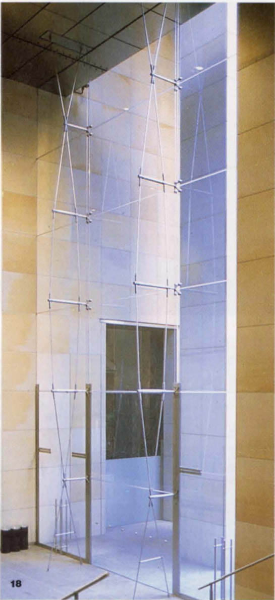
11. Courtyard loggia screen.
