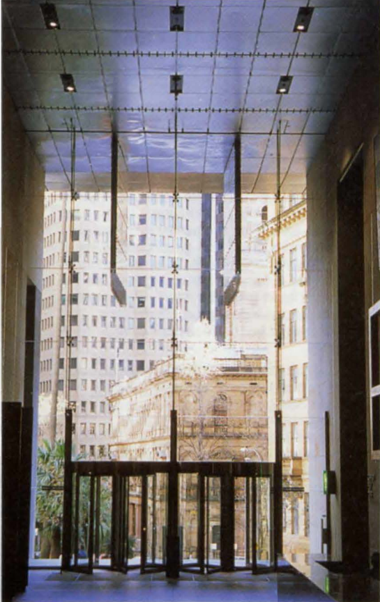
10. Loggia screen to exterior (Farrer Place).
