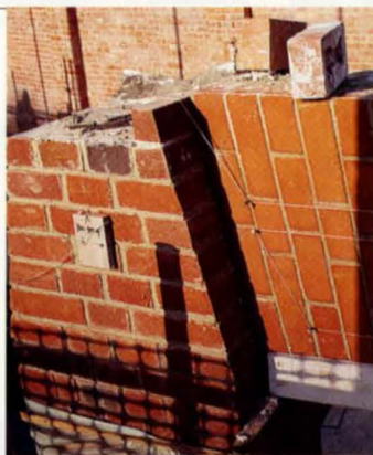
◀ 4. Brickwork detail on arch.
