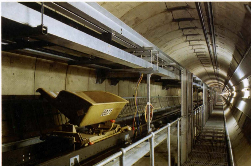
11 Below: The completed main tunnel at an early stage of fitting-out, showing the walkway, both baggage tracks, and one of the 400 destination-coded vehicles.
