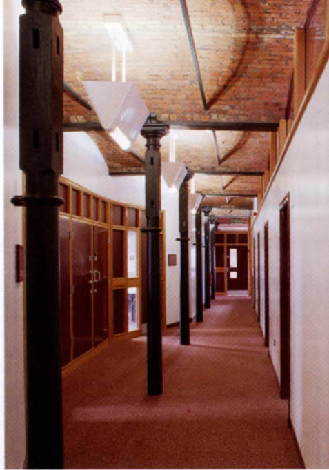
7. Typical upper floor corridor.
