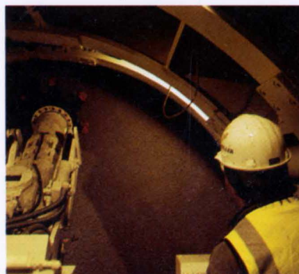
8. The roadheader inside the tunnelling machine, ready for excavation.
