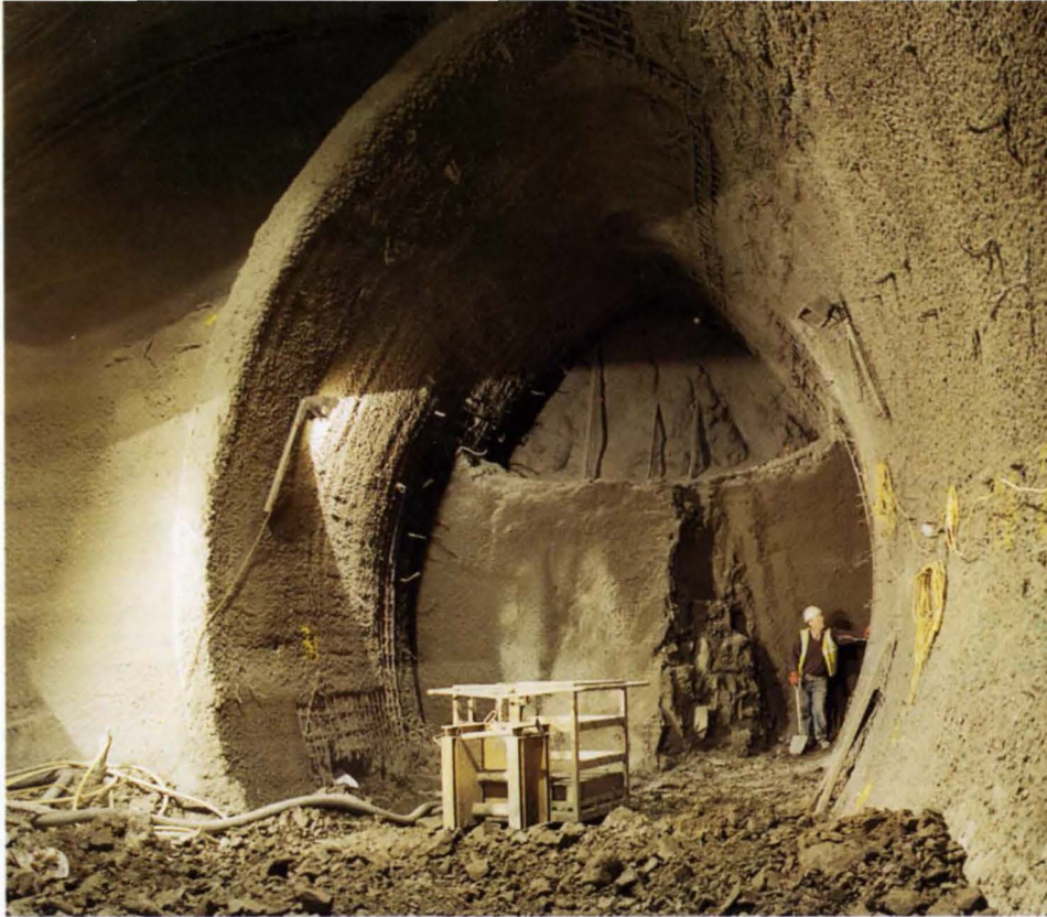
9. 8.3m diameter NATM chamber at Terminal 1, during excavation and primary lining of side wall drift.
