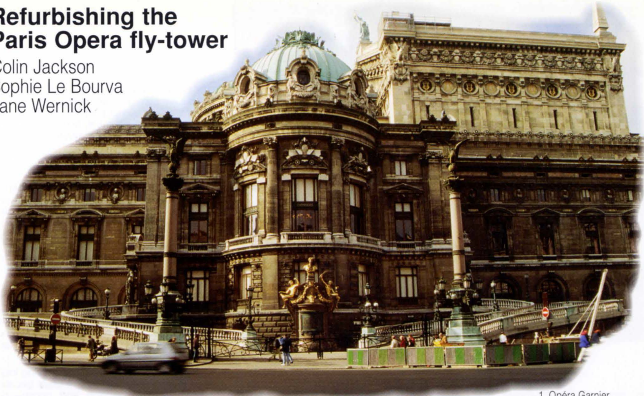
1. Opéra Garnier, showing fly-tower on the right.
