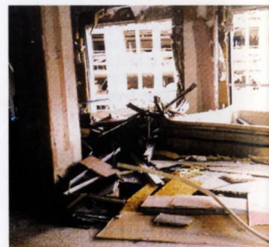
9. Bomb damage at Bishopsgate.
