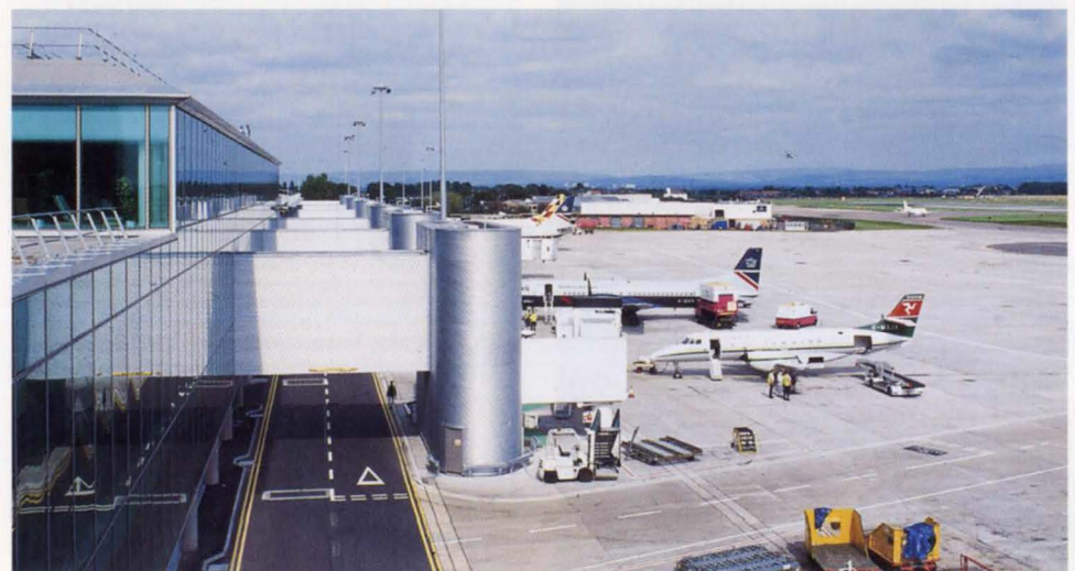
5. New stands and apron.
