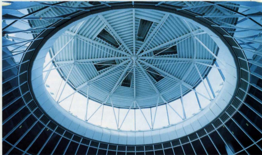
13. Clerestory frame above new international lounge, T3, containing smoke ventilators.
