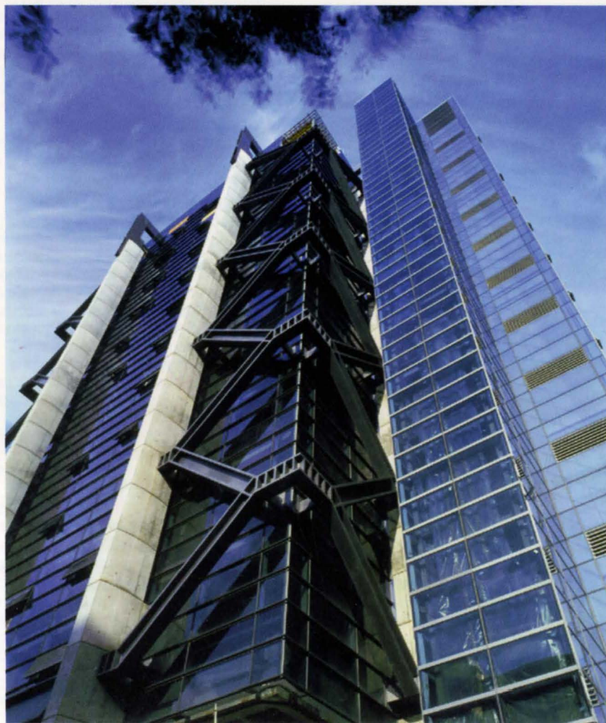
8. Corner detail of building as constructed.
