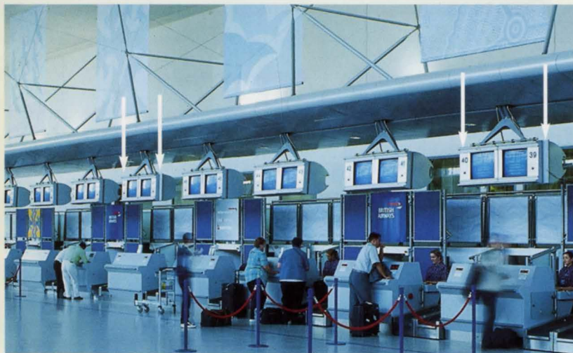
11. Completed T1 BA check-in hall showing Penton MC-402 column loudspeakers on the row of monitor housings (arrows indicate typical positions.)
