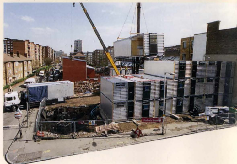
6. Example of paired modules being installed.
