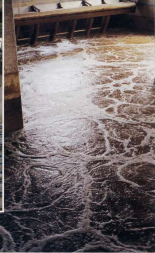
14. Treatment basin in aeration cycle.
