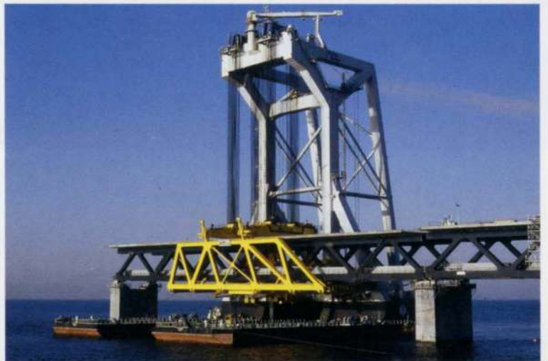
17 right: Svanen placing approach girder.
