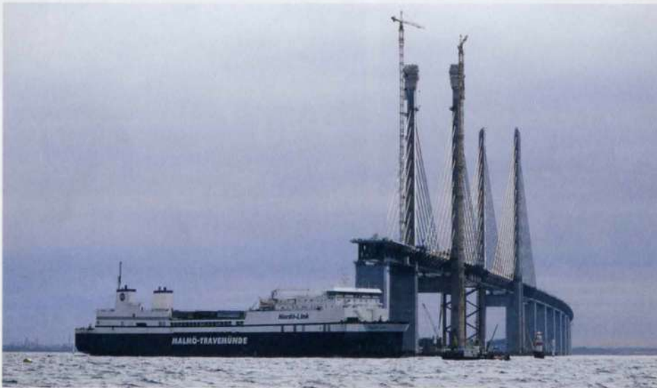
22 left: The original navigation channel was used until main span was completed.
