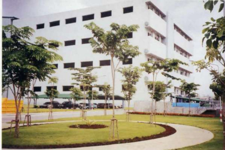
8. The treatment plant.
