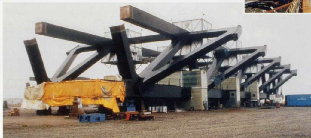
11. Main span girders were fabricated in Karlskrona.
