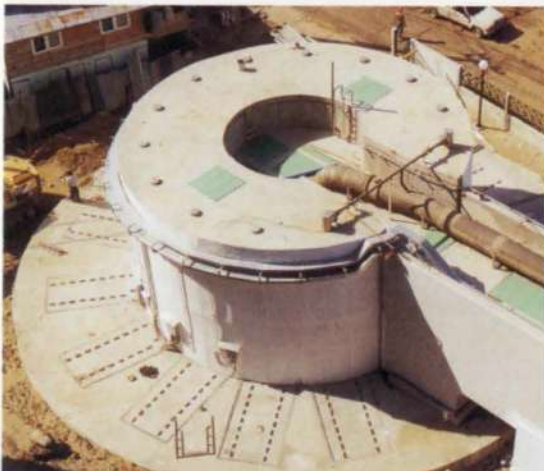
9. Inlet pumping station.
