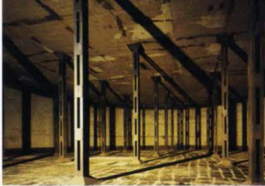
19. One of three similar chambers which contained oil tanks for the power station. These may form a future phase of Tate Modern.
