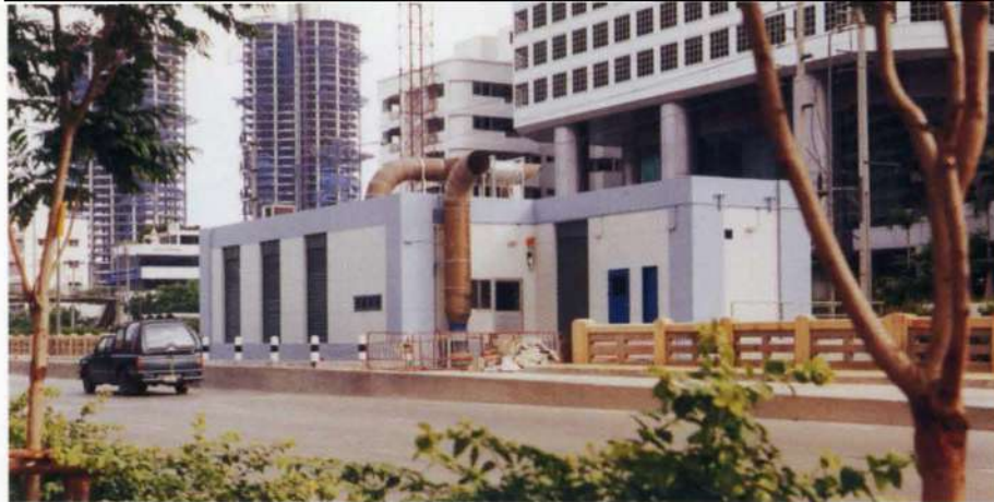
6. Collector system pumping station built over khlong.
