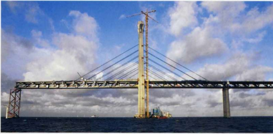
20. The main span was erected in four sections supported by temporary towers.
