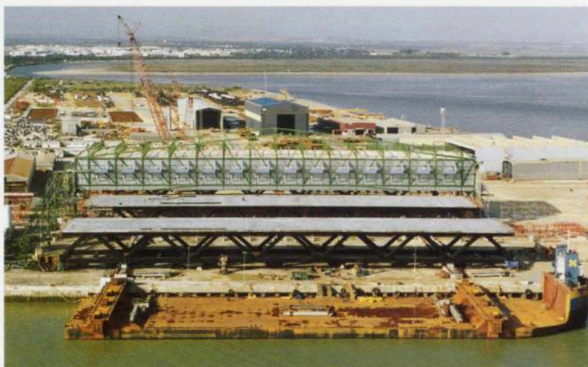
8. Two completed girders are ready for being transferred to ocean-going barge.
