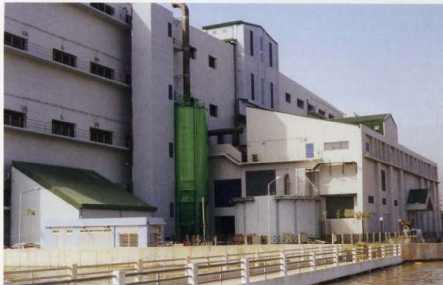
18 below: Treatment plant seen from Khlong Chongnonsee.
