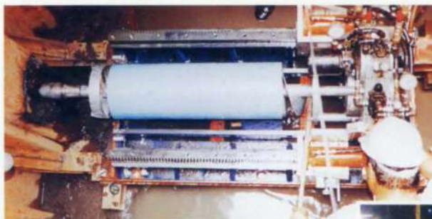
3. Direction drilling for small diameter pipe.
