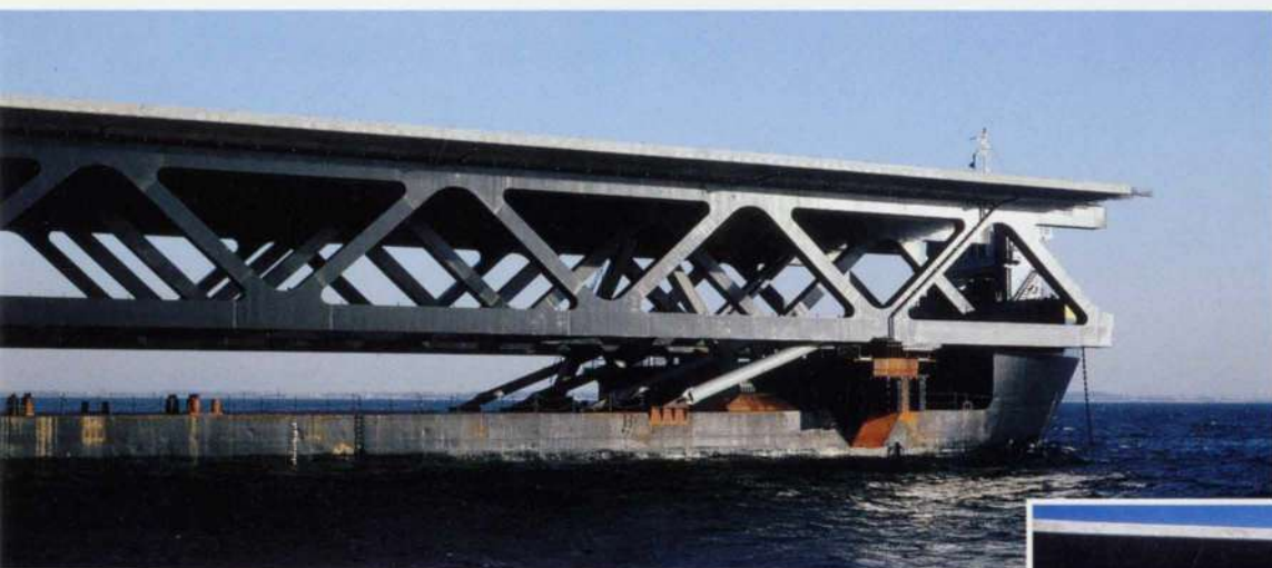
9. Approach girders on barge en route for Malmö.
