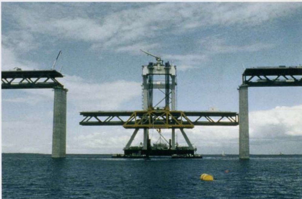
19. The last girder is placed.
