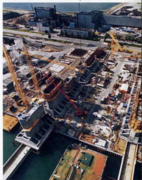
4. Caissons were cast at the Malmö yard.
