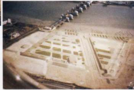
5. Aerial view of site after completion of the remedial works.
