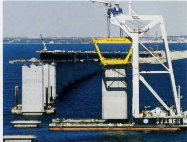
15 below: Svanen placing pier shaft.
