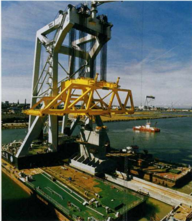
14. Svanen lifting caisson at the Malmö yard.
