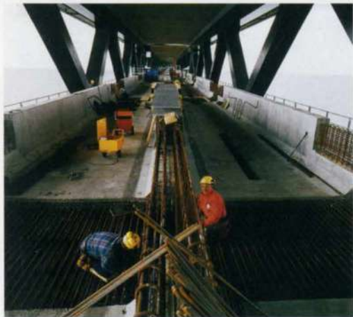
18. Completing the railway deck in approach bridge.
