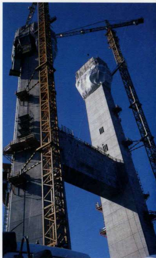
12 above, and 13 below: The main pylons were cast in situ.
