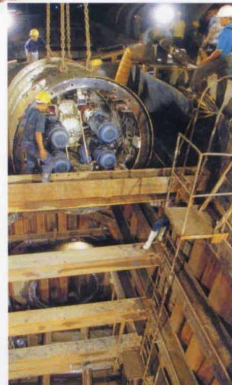
4. 2.25m diameter pipe jack being lowered into excavation.
