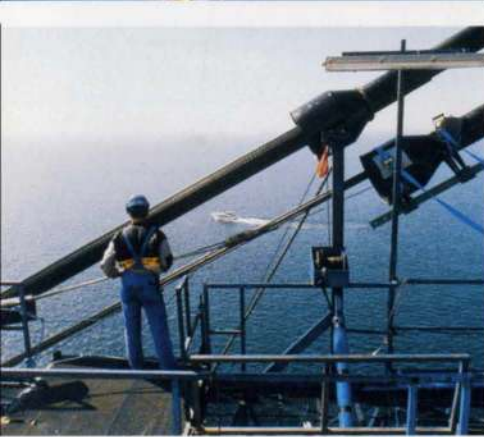
24 above: Placing the main cables.
