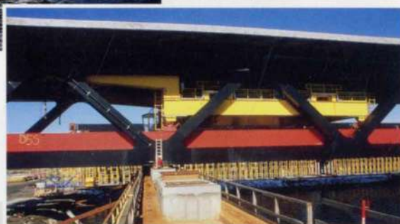
10 below: The lower deck in the approach girders was completed in the Malmö yard.
