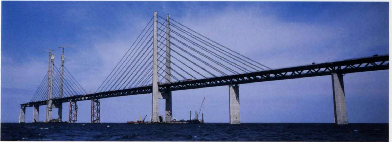
21 above: The main span nearing completion.
