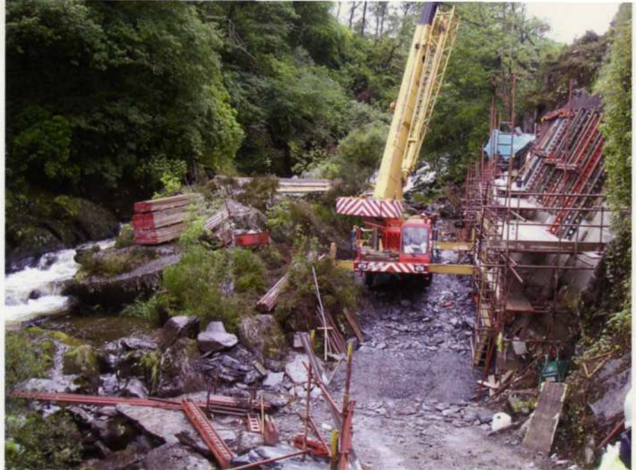
6. Constructing retaining wall No. 6 at Pont-y-Pant.
