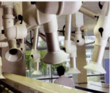
8. Laboratory air extractors.
