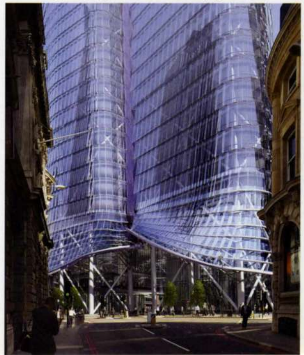
3. Complex canopy entrance to the Bishopsgate Tower.
