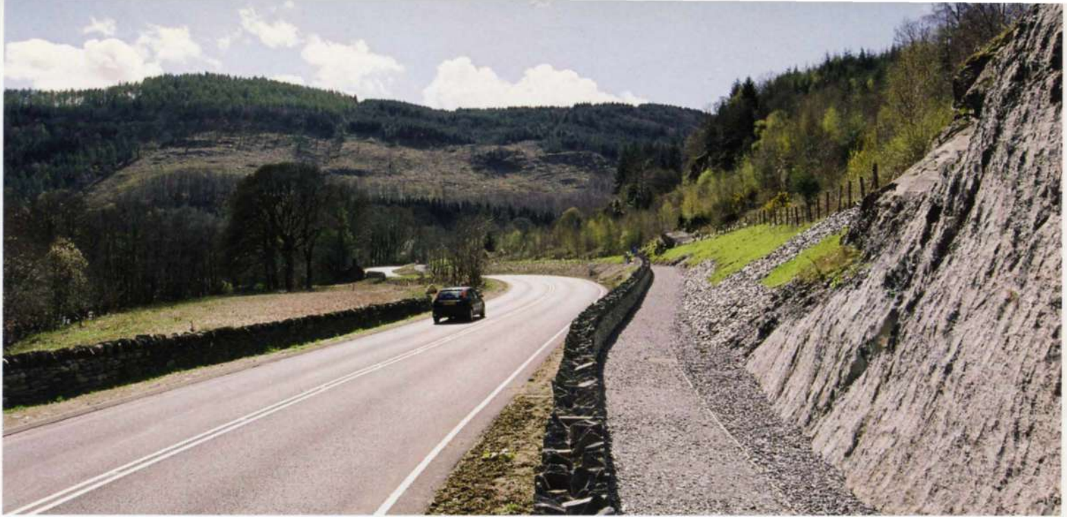
1. The new community route alongside the improved road.
