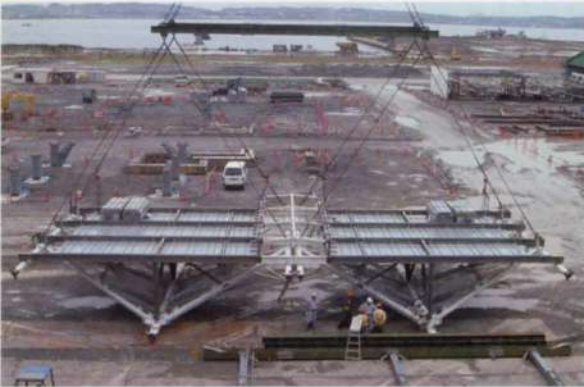
14. Roof truss module ready to be raised.
