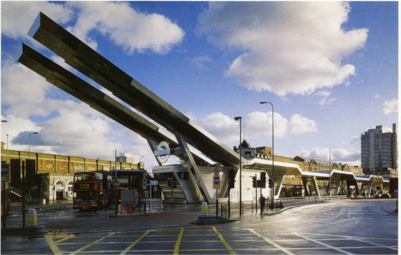
5. View from the apex down the 'Ribbon' concourse.
