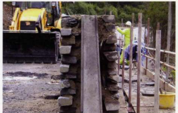
4. Stone-clad containment parapet.
