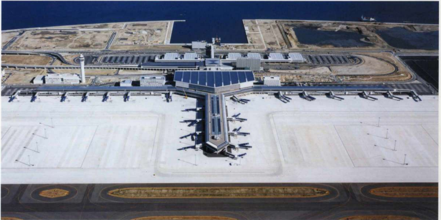
1. The new terminal building complete, on its island location.
