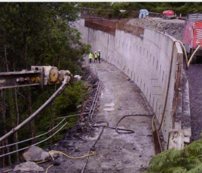
5. Anchored panel wall.
