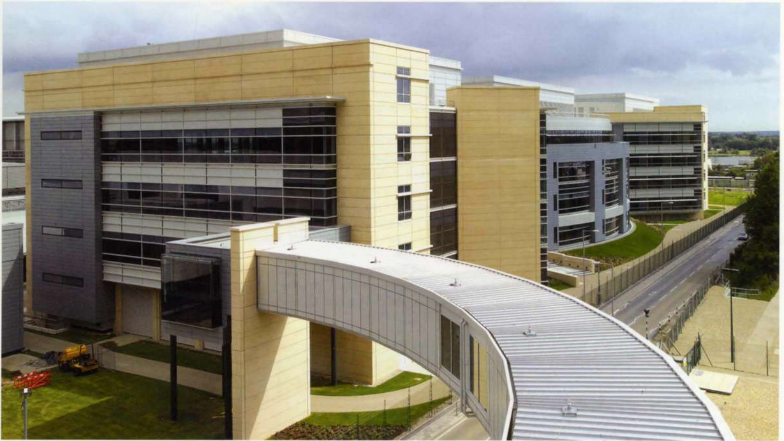
13. Connector link bridge and western elevation.
