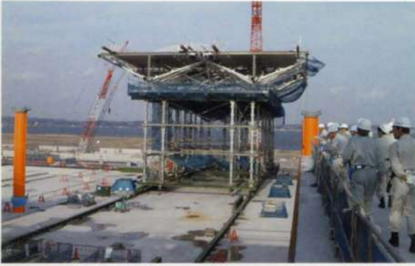
13. The first roof truss modules in position.
