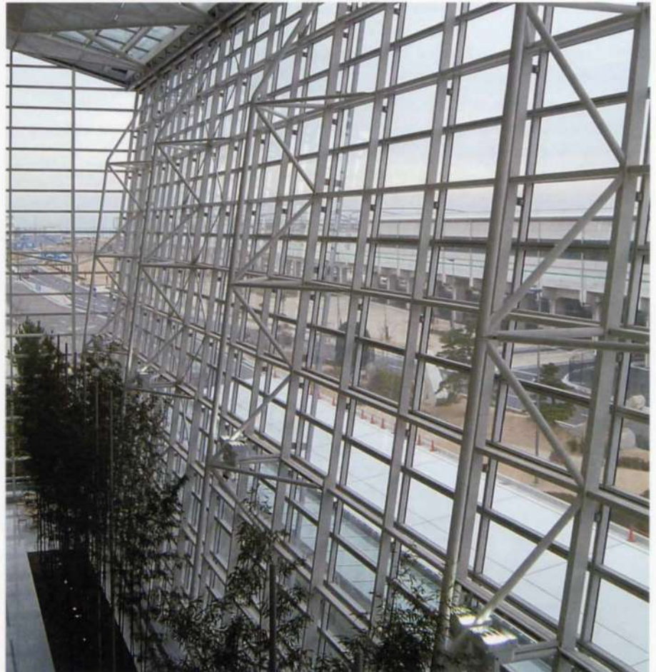
15. Façade support structure at the 'welcome garden'.
