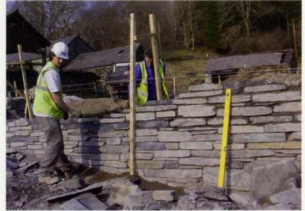
3. Constructing boundary walls.
