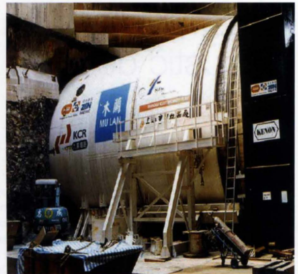
3. Front shield of TBM in launch shaft.
