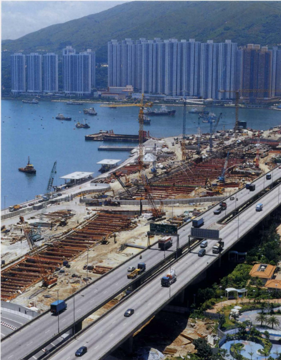
18. The Tsuen Wan bypass elevated highway runs along the north-east side of the site. The risk of the excavation works causing excessive ground movements that might affect the structure were mitigated at design stage by the choice of preloaded struts and by adjusting the railway alignment to bring the structure outside the zone of influence of the excavation.
