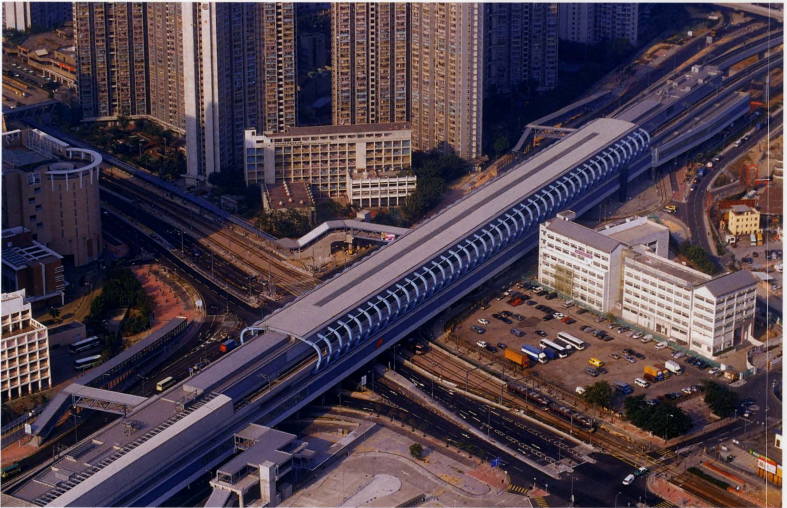
21. Roof cladding at Tin Shui Wai station.
