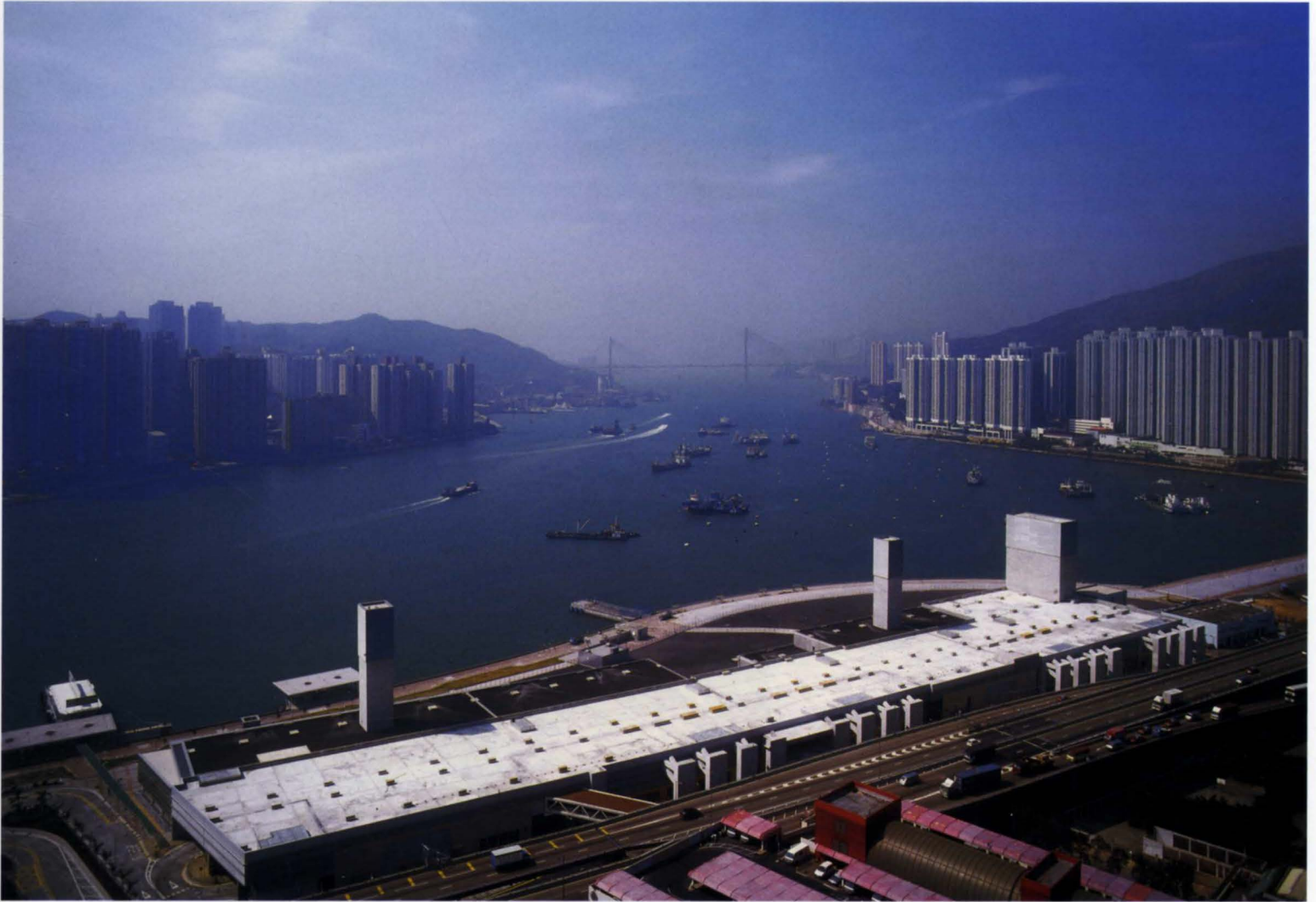
22. North-east elevation of Tsuen Wan West station, with Tsuen Wan bypass in the foreground and Rambler Channel beyond. In the distance is the cable-stayed Ting Kau bridge carrying road traffic into the New Territories to the north, part of the complex of bridges built to handle traffic to and from the new Hong Kong International Airport.
