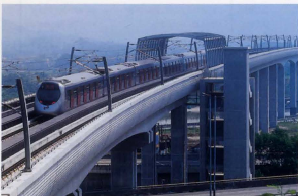
2. Part of the West Rail viaduct at Au Tau.
