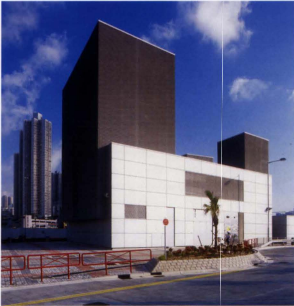
15. Southern transformer building.
