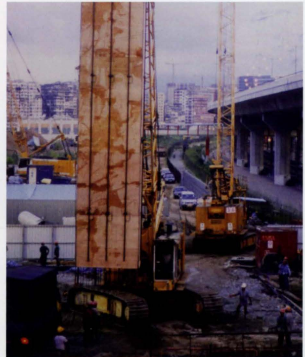
5. De-bonding liner to barrette test.
