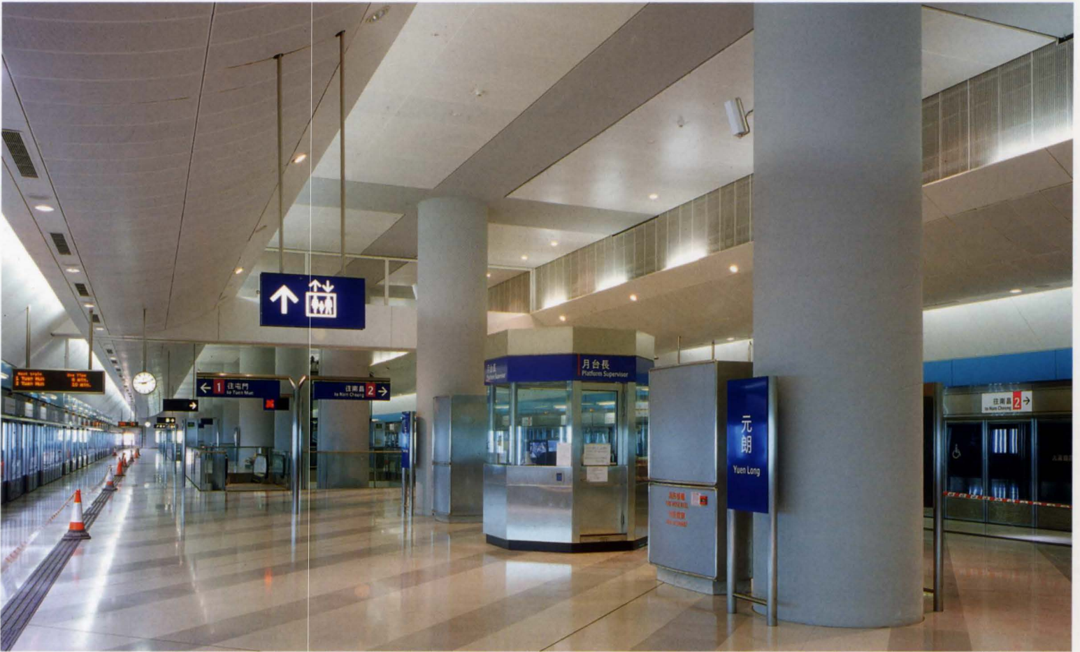
1. Yuen Long Station platform: sound absorption is by absorbent material behind the perforated ceiling panels.
