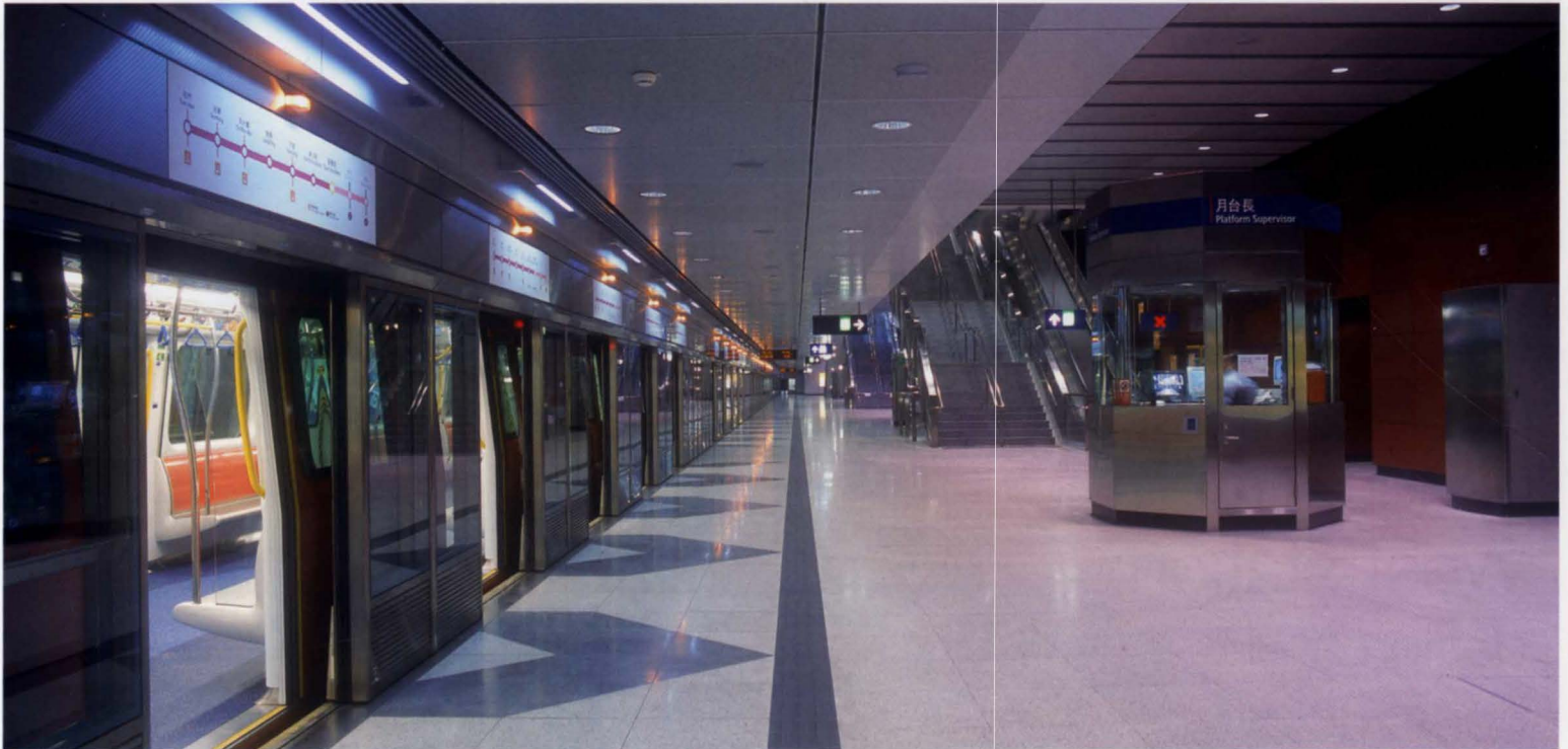
4. The platform extends to over 5m width between escalator/stair zones.
