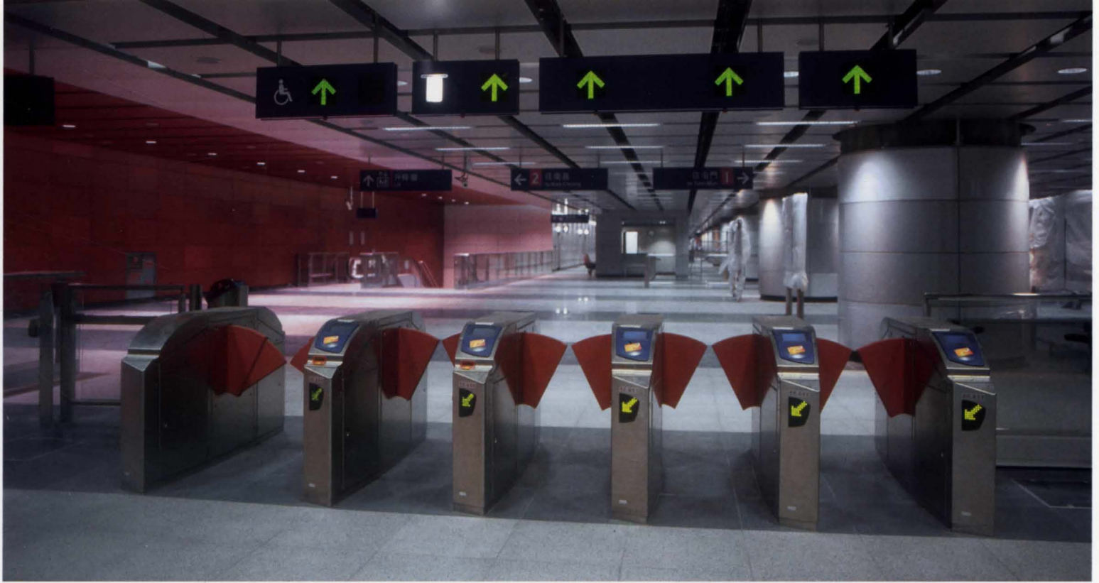
5. The concourse level, showing columns designed to carry future property development above the station.
