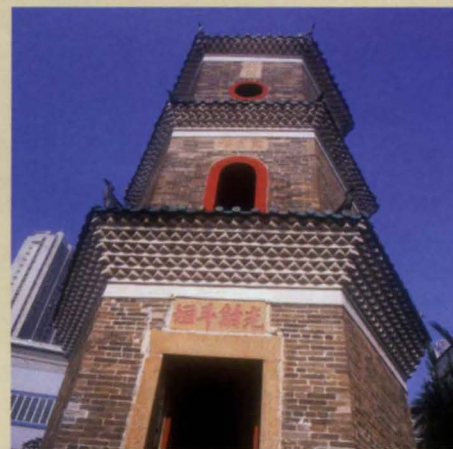
28. Tsui Shing Lau pagoda, showing ornamental brick corbelling.
