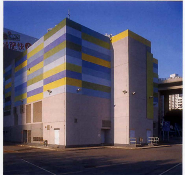
3. Chai Wan Kok Ventilation Building at south end of tunnel.
