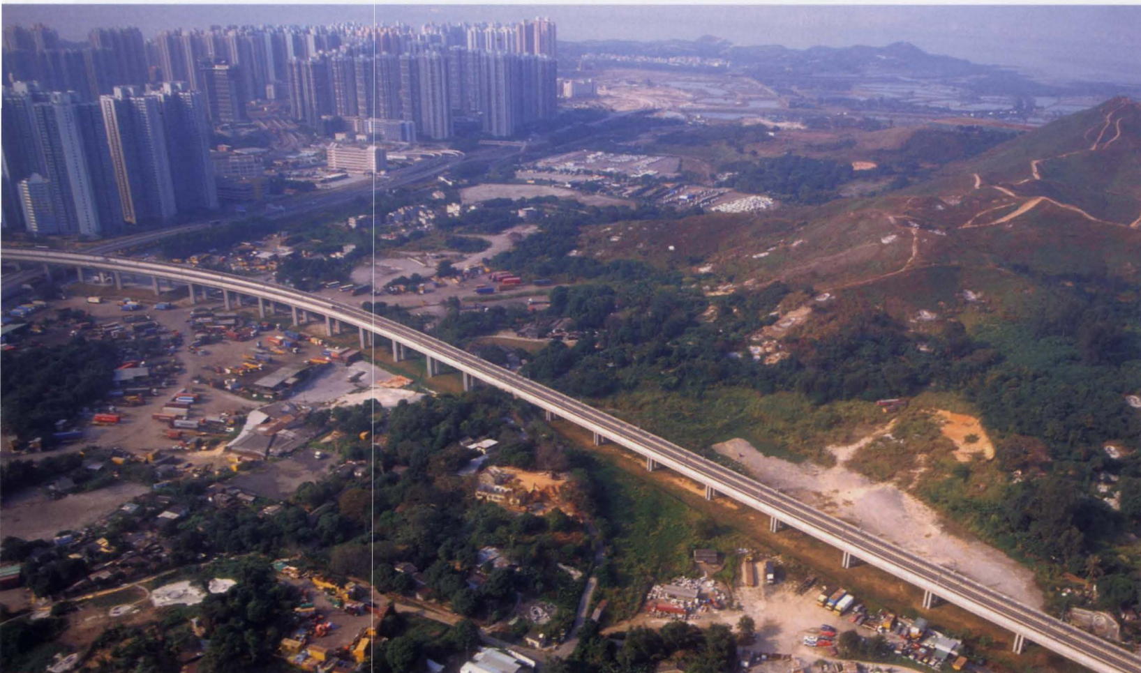
4. Yuen Long viaduct from the air, approaching Tin Shui Wai on the left.
