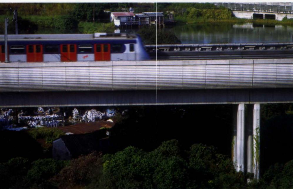
9. The parapet in use.
