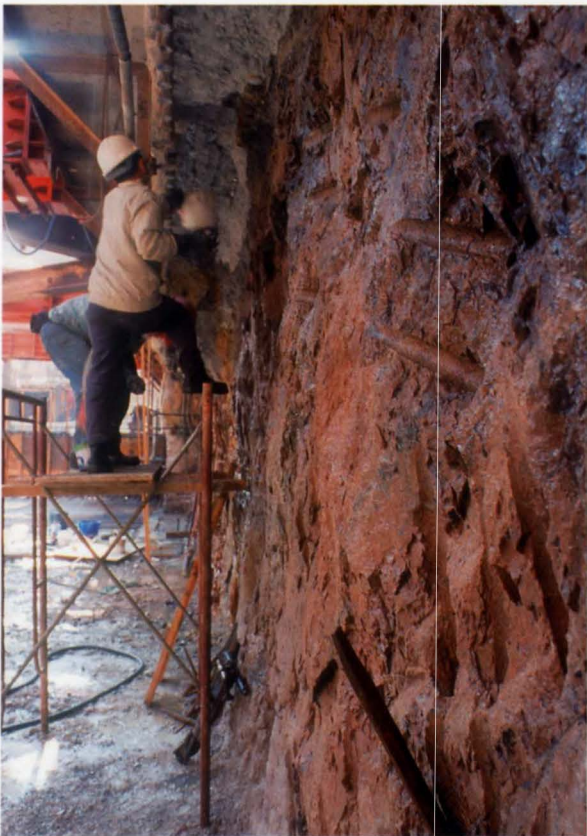
19. Underpinning of diaphragm wall panels.
