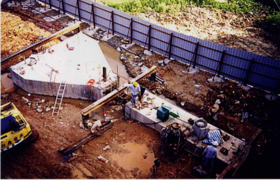
3. Lateral load test on pile groups.
