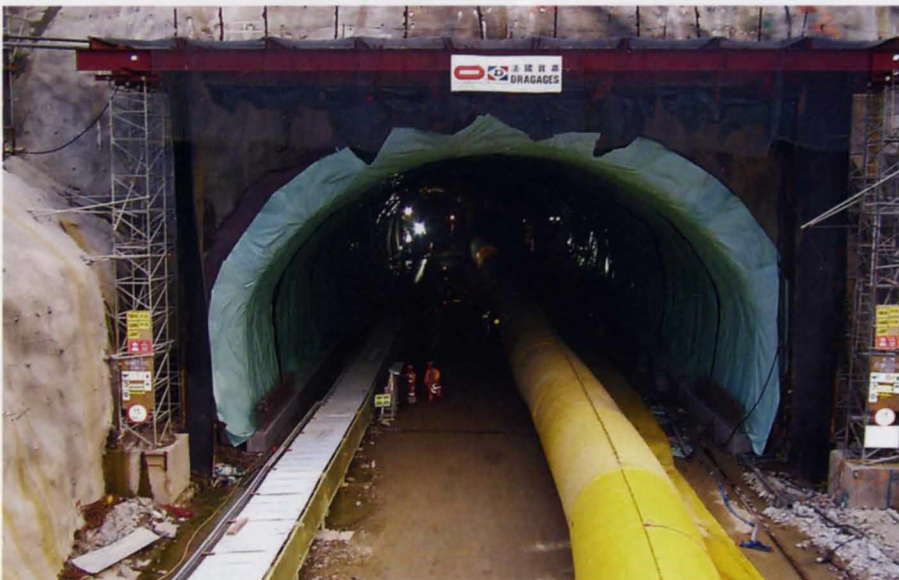
1. The Tai Lam tunnel north portal.
