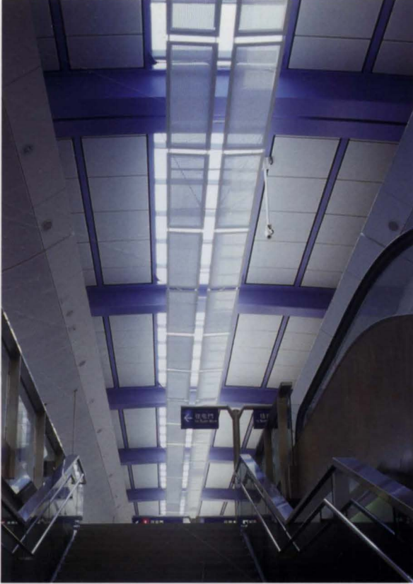
18. Central rooflight at Tin Shui Wai station.
