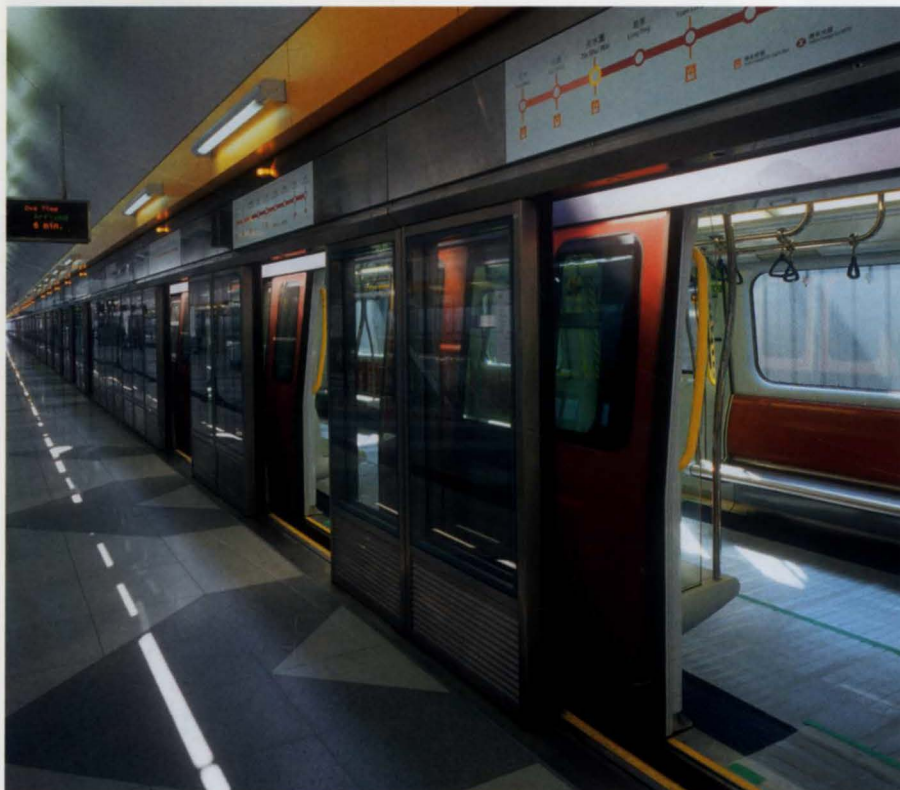
27. Train at rest in Tin Shui Wai station, with platform screen doors open.
