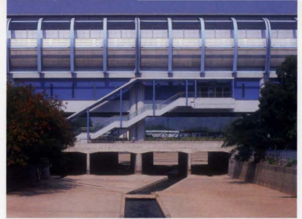
25. Long Ping station is constructed over stormwater collection channels (nullahs).
