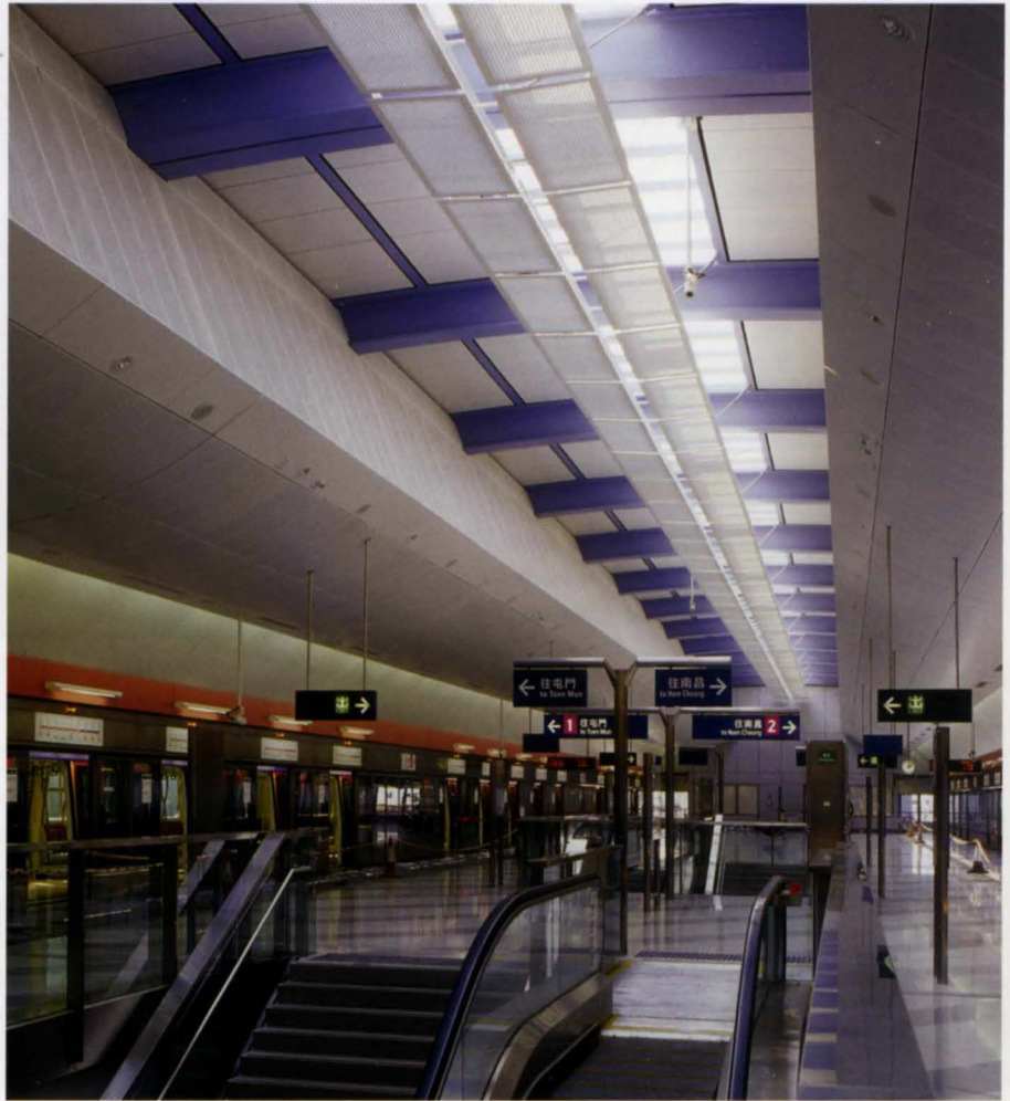
5. Acoustic ceiling panel at Long Ping station.
