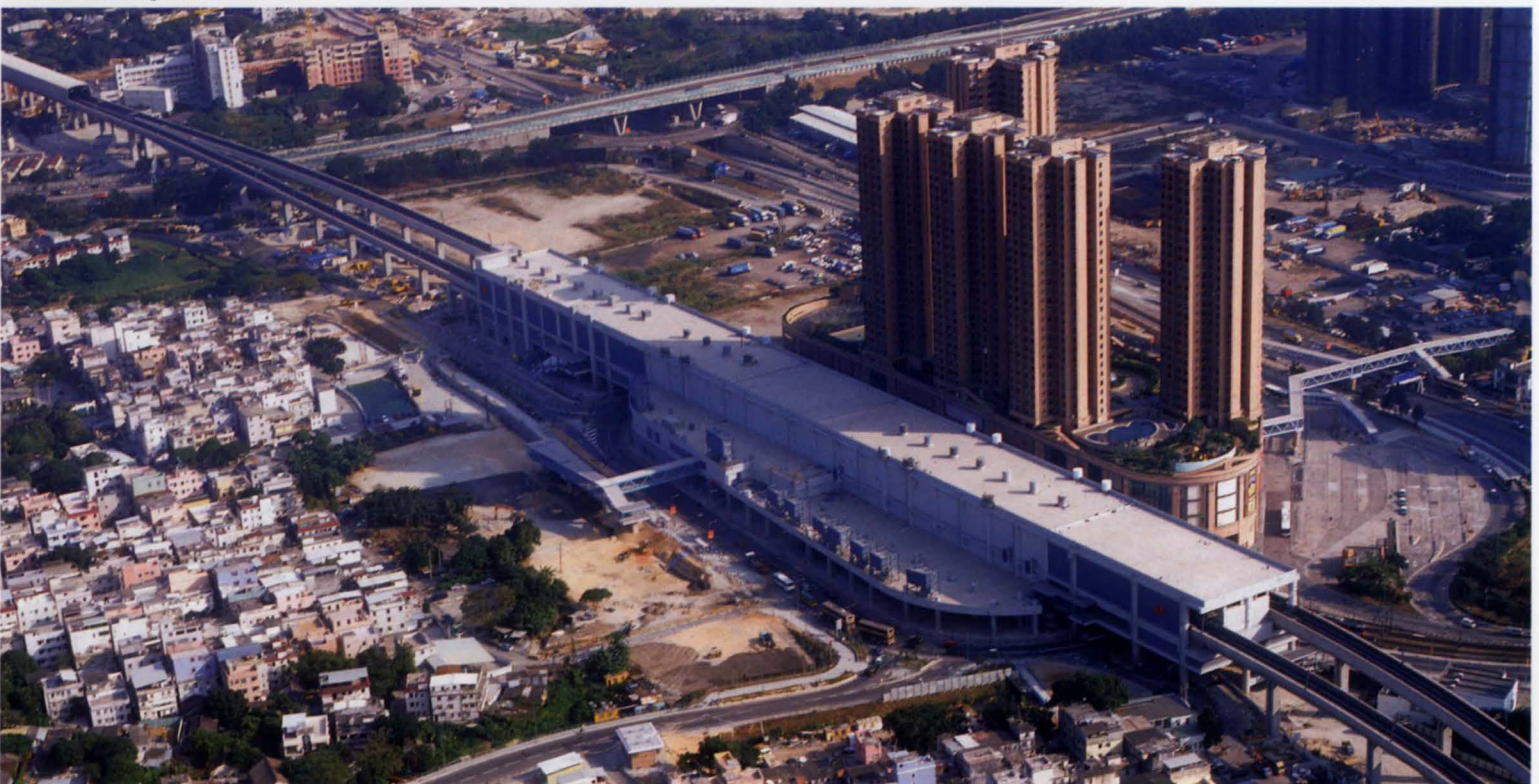
23. Yuen Long station in context.
