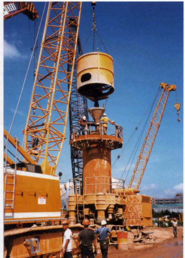
5. Large capacity rotator was used for pile casing installation and the subsequent casing extraction during concreting.
