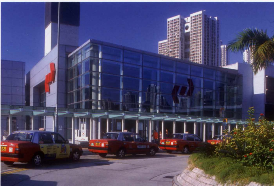
7. The main station entrance.
