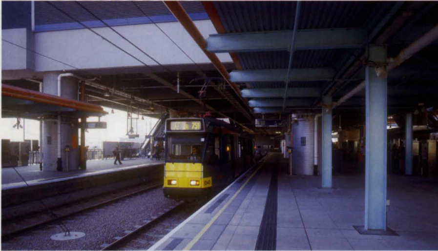
4. New LRT platforms beneath Tin Shui Wai station.
