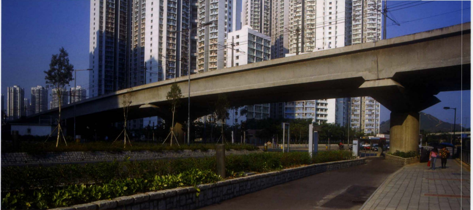
1. Viaduct across Tin Fuk road carrying light rail in and out of the at-grade platforms under Tin Shui Wai station.
