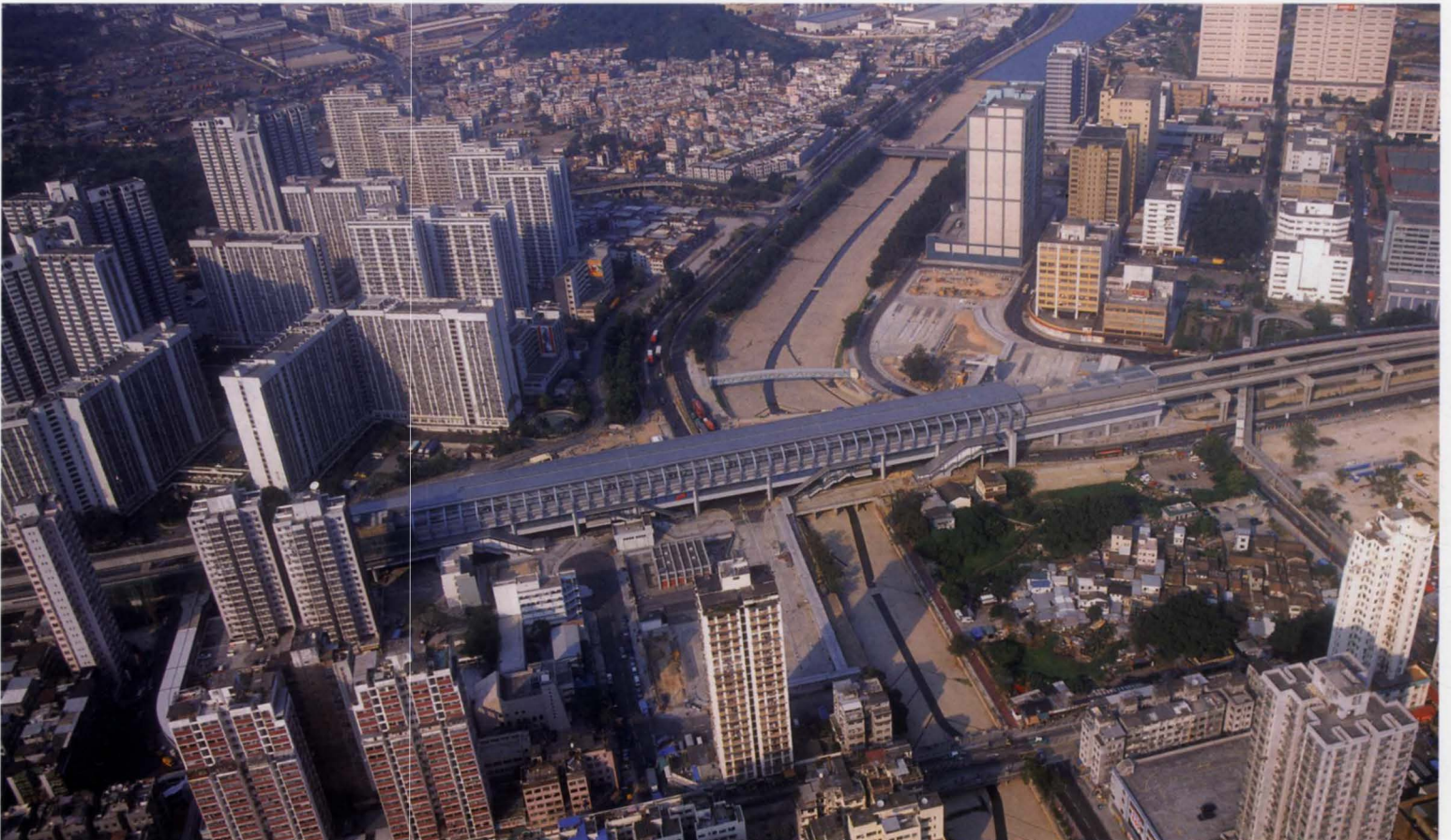
24. Long Ping station in context.
