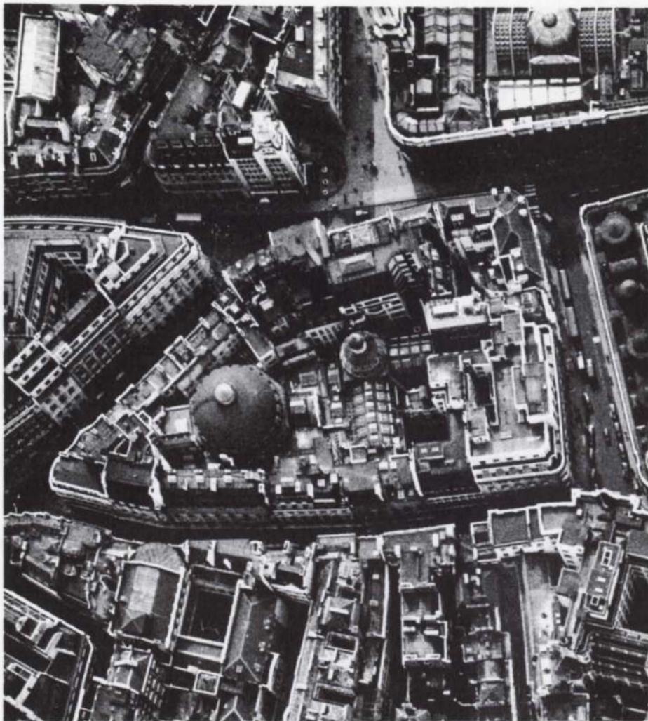
Fig. 1 The Stock Exchange before reconstruction, aerial view. (Photo: Fairey Surveys Ltd.)
