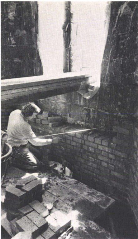
Fig. 14 Laying the brick lining (Photo: Poul Beckmann)
