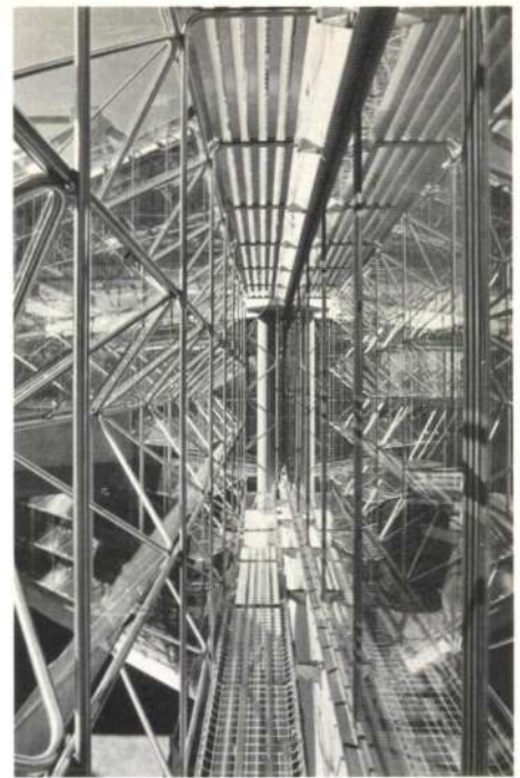
Fig. 5 Space frame sun shading (Photo: David Moore)
