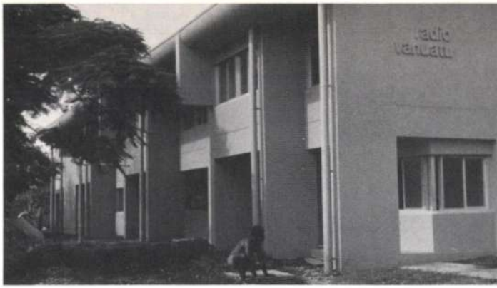
Fig. 4 Studio building showing the emphasis on sun shading to windows and rain water dispersal (Photo : H. Calverley)
