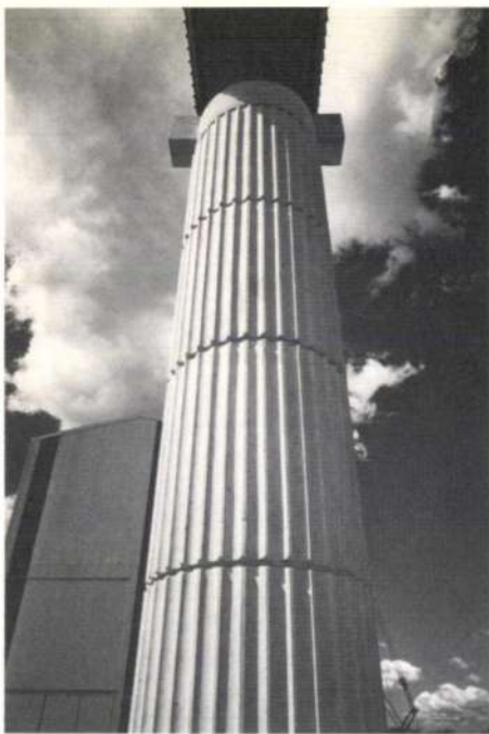
Fig. 8 Conveyor support shaft (Photo: Max Dupain)
