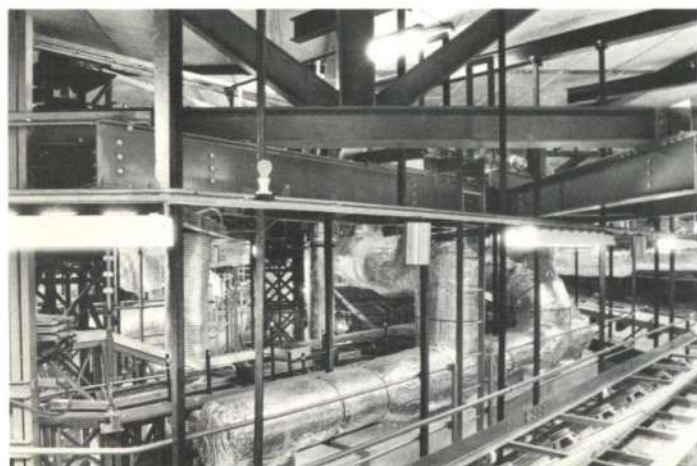
Fig. 9 Ceiling structure and services installations
