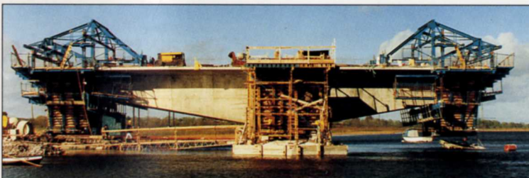
10. & 11. Cantilevering in progress.
