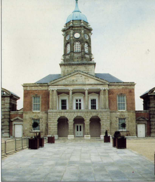
10. Castle Hall and Bedford Tower.
