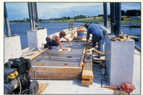
9. Installation of bearing plinth, temporary props.
