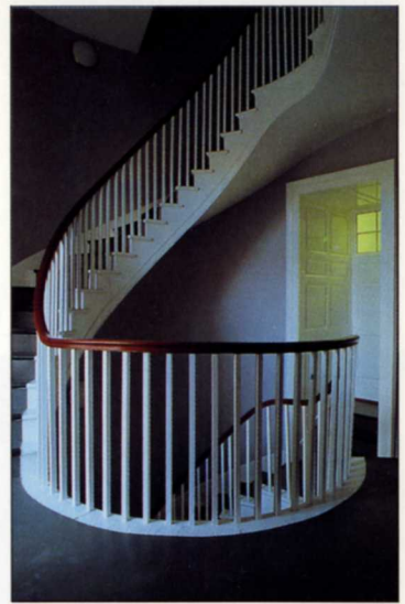
12. Bedford Tower: central stairs.
