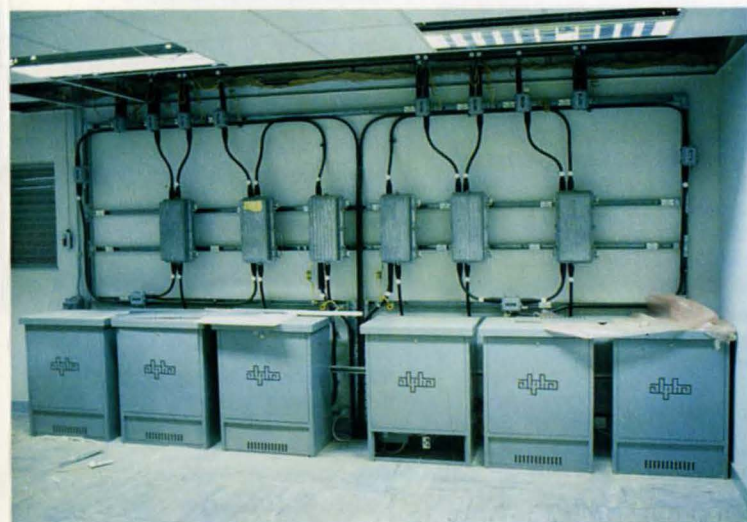
3. Toyota broadband installation. (Photo: Ove Arup & Partners)
