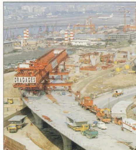
3. Launching girder near junction of Phases II and III, January 1990.
