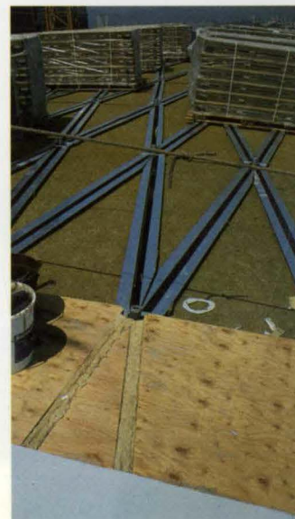
◀ 14. Layers of Deliberatif roof; top: insulation and vapour barriers in steel frame; middle: plywood panels; bottom: weather seal membrane (white).
