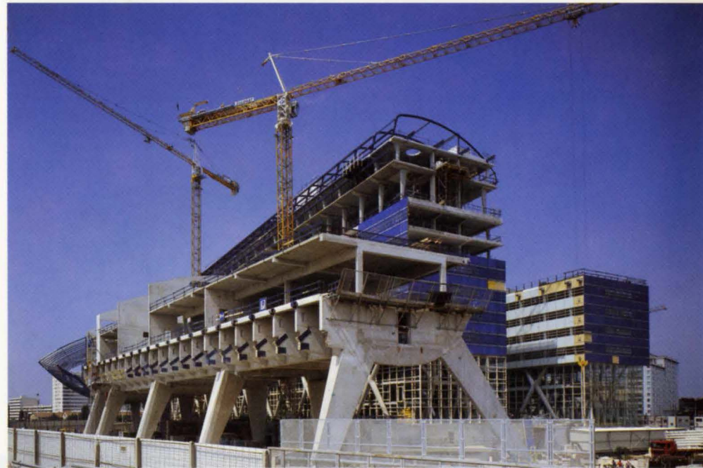
13. The Deliberatif under construction, showing the concrete platform.
