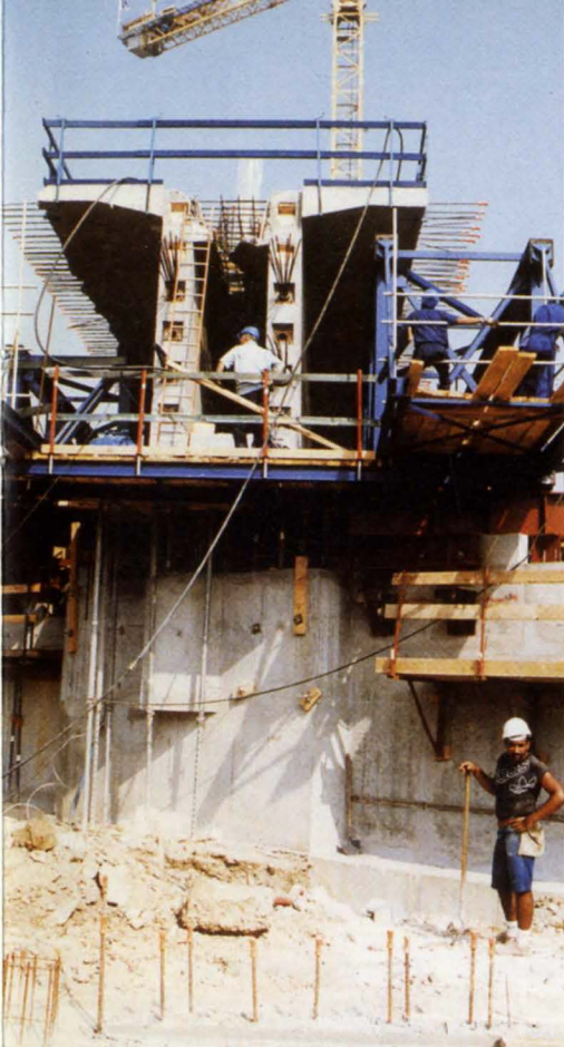
◀ 17. End view of transfer beam over metro station.
