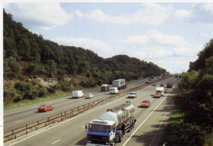
12. Existing rock cutting at Trentham in Staffordshire, on the M6 motorway.
