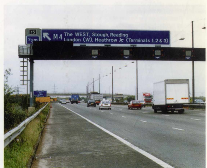
17. Typical gantry over a dual four-lane motorway, with matrix signals for lane control and a variable message sign.
