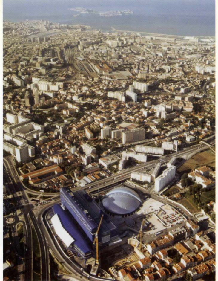
18. ▶ The Marseille context, viewed from the north east; behind the Hôtel is the Salle de Rock, a new community facility; in the foreground, a deep car park to serve both buildings.
