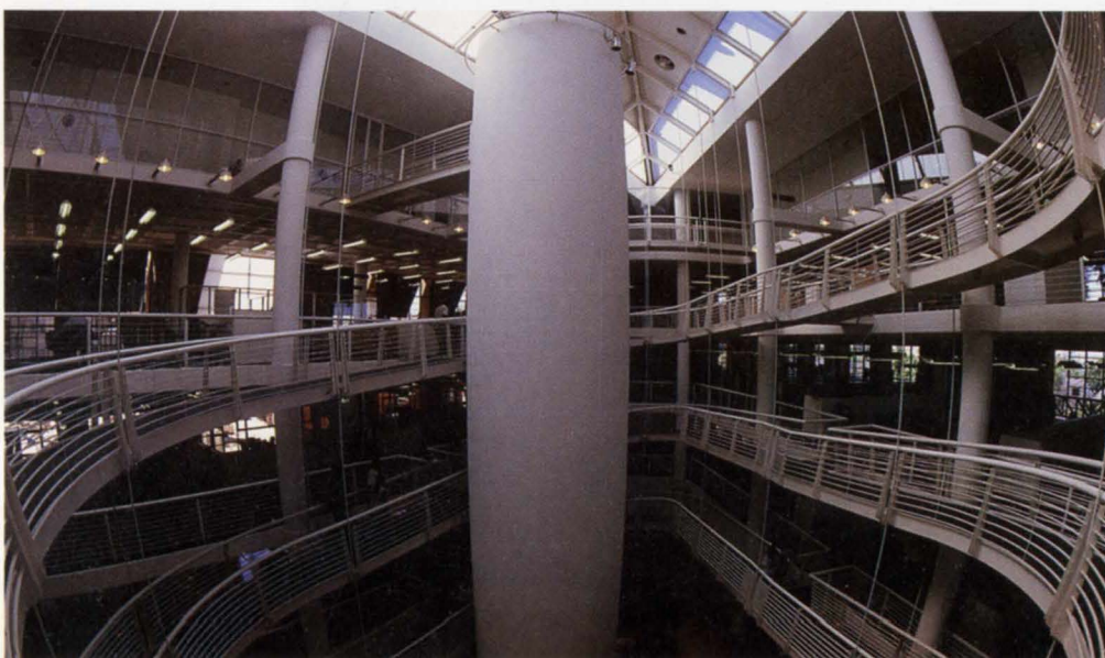
7. Lift core at atrium roof level encircled by pedestrian ramp.
