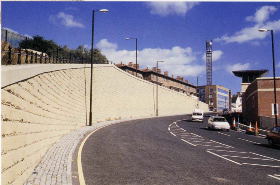
15. Below: Retaining wall K completed, September 1995.
