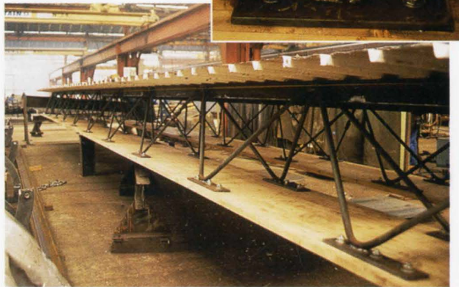
24. Prototype trusses ready for load testing.
