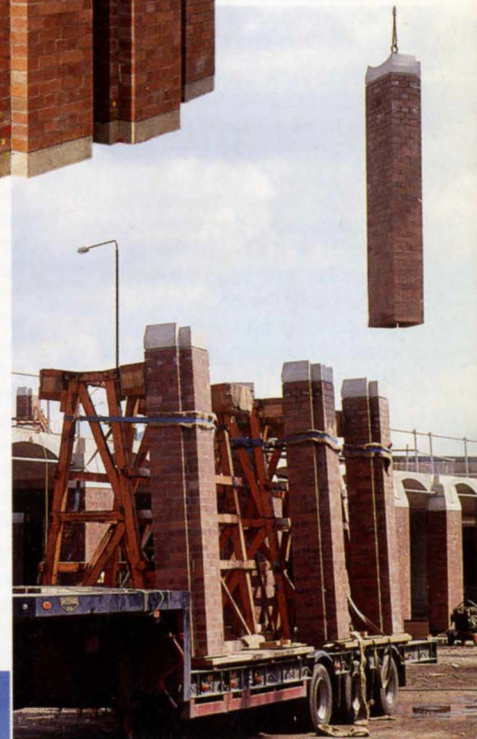
6. Lifting a brick pier.
