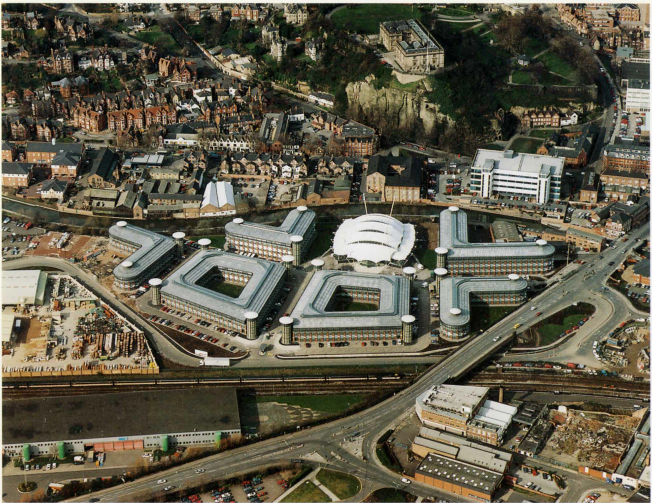
1. Inland Revenue HQ looking north; Nottingham Castle is at the top of the picture.
