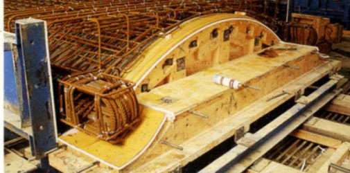
8. Timber mould for ends of units.
