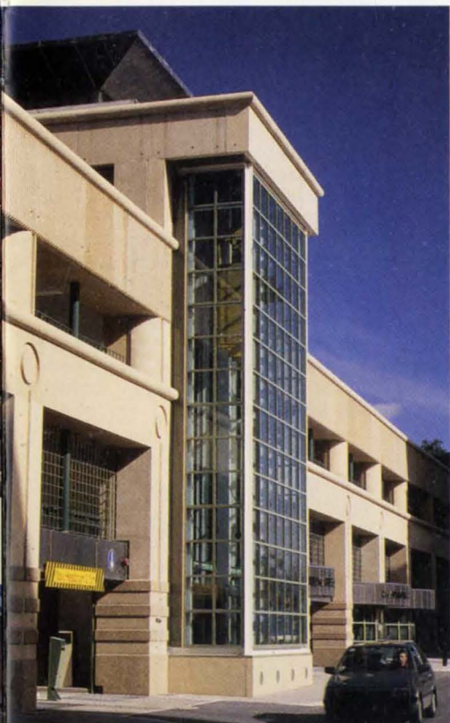
18. Above: Front elevation of multi-storey car park Phase 1, September 1995.
