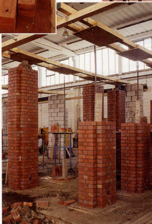
4. Brick piers under construction.
