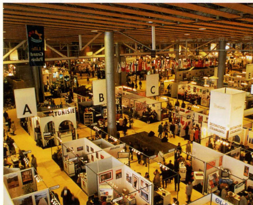
18. Exhibition Centre interior in operation. The braced rail below the ceiling supports the heavy acoustic partition, open here to utilise the combined hall area.
