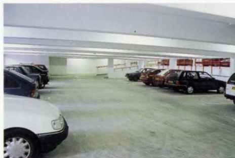
19. Interior of Phase 1 car park.
