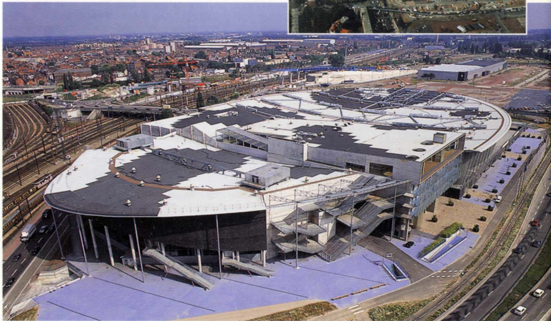
1. Aerial view to the south, with inset 2. showing the Lille Grand Palais in the foreground, and the Euralille commercial centre and TGV station beyond.
