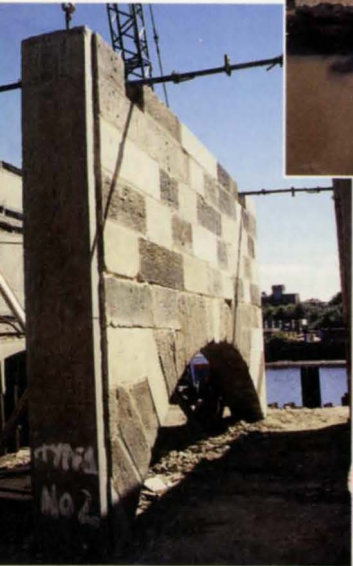
6. Left: Precast stone-clad arched panel, June 1994.
