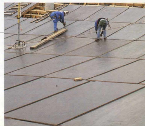
8. Right: Articulating modular formwork panels being assembled for the Zenith gallery floor slab.
