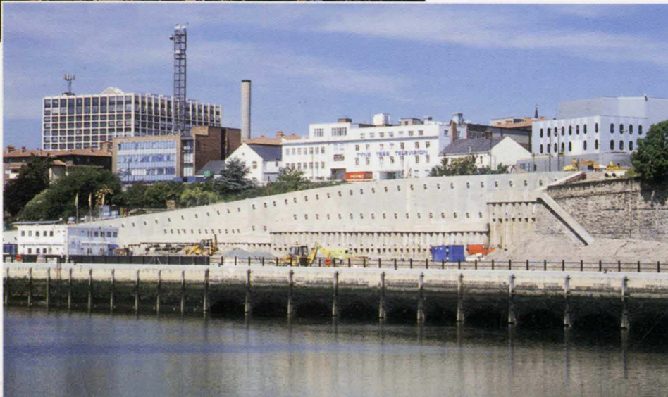
17. Completed retaining wall D, June 1995.
