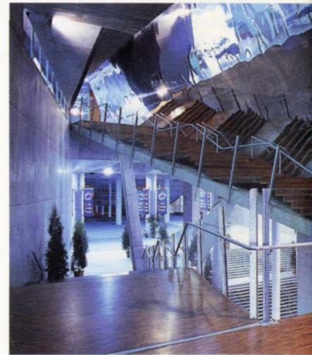
5. Above: The overlapping ramped main staircase of Congrès, enclosed by inclined stainless steel clad walls.
