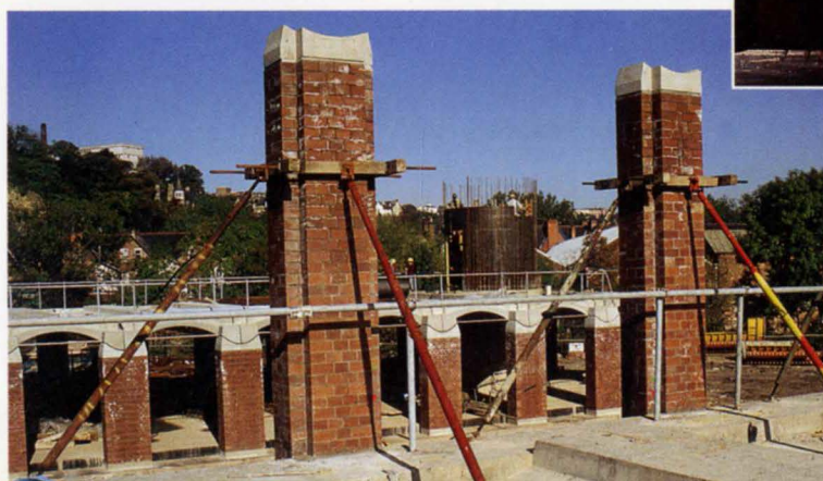
7. Brick piers ready for floor units.
