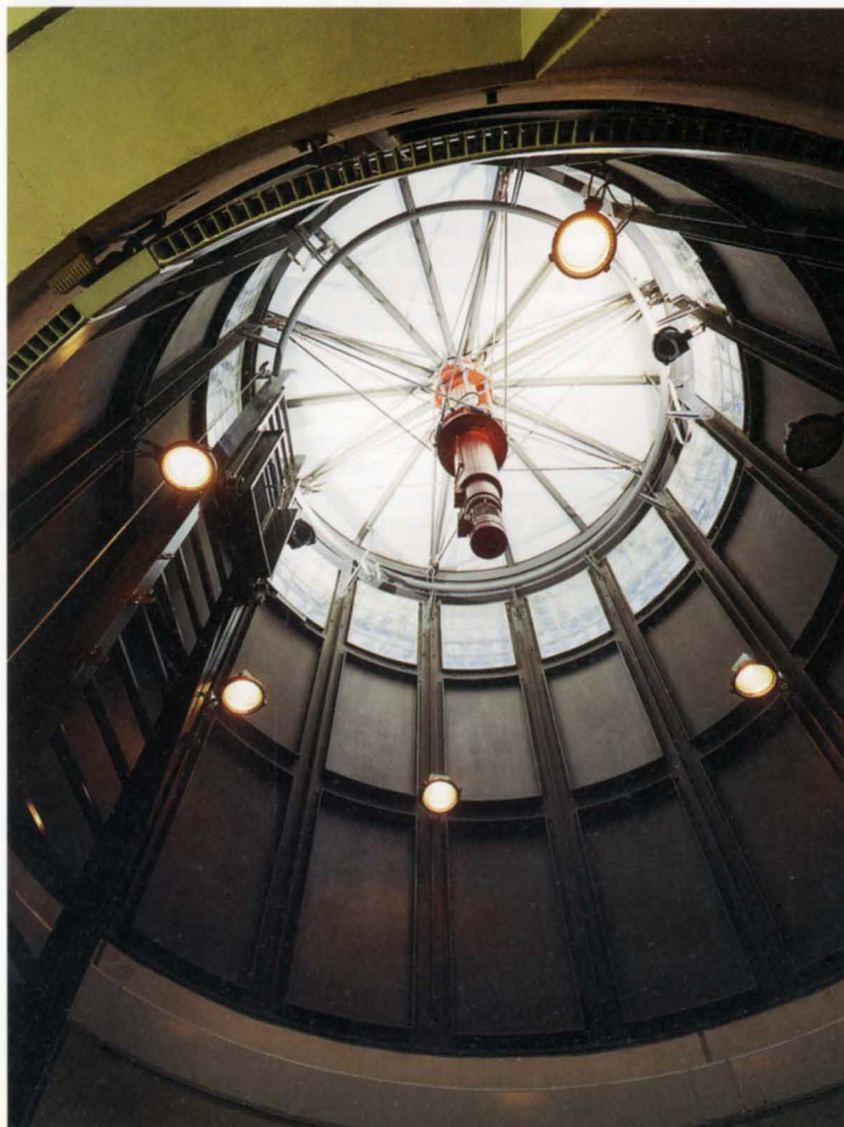
19. Inside a glass stair tower.
