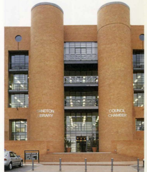
4. East elevation entrance from the forum, showing cylindrical stair and lift cores.
