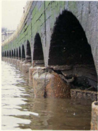
4. Quaywall - existing structure, February 1993.
