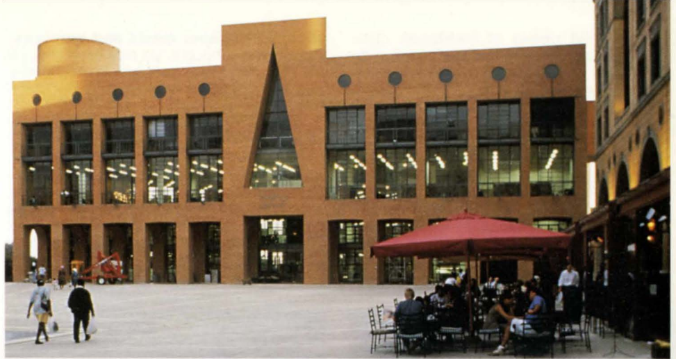
1. West elevation, viewed from Sandton Square.
