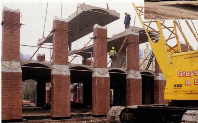
11. Placing a floor unit.
