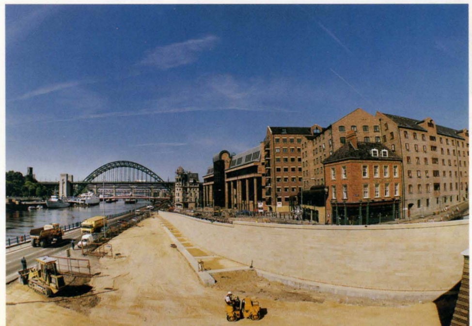
12. Below: Completed retaining wall A, September 1993.
