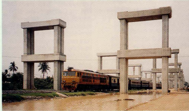
3. An SRT train between part of the two-storey BERTS structure.
