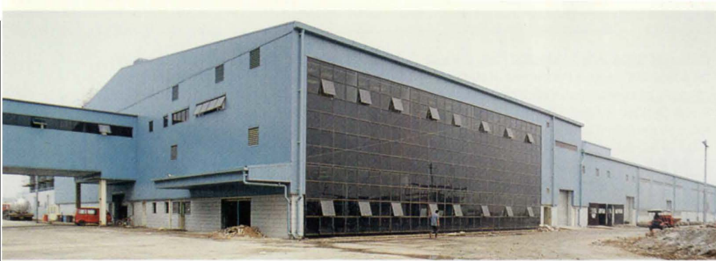
6. Offices in northwest corner of process building.
