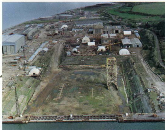
2. Nigg dry dock looking north before the start of the refurbishment works.
