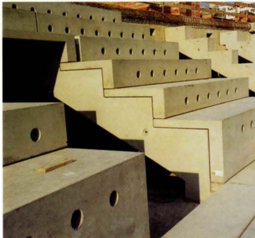
9. Seating units showing air diffuser holes.
