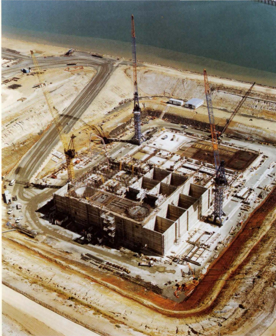
2. Caisson slipforming in progress, December 1995.
