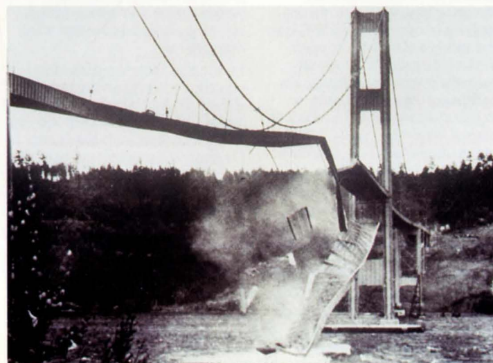
3. Tacoma Narrows Bridge - The need for smart structures?
