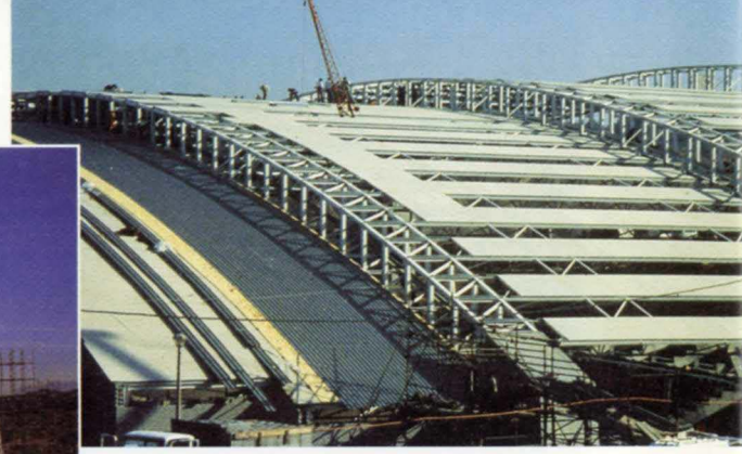
4 Above: Roof cladding in progress, May 1997.
