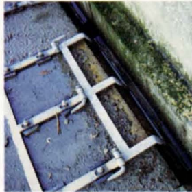
Replacement north nib bearings on their support frames.
