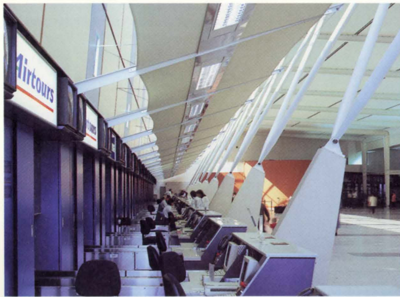
6. Check-in hall showing the division of check-in desks by pre-cast concrete piers.
