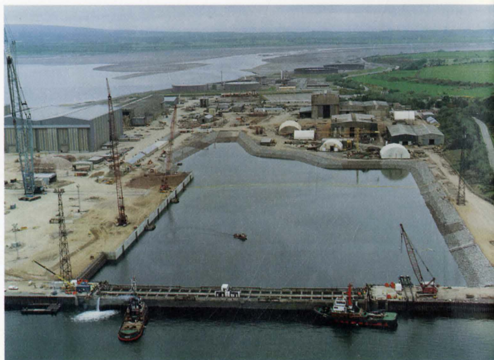
3. Dry dock flooded following completion of the new quay wall (left in picture) and slope works.
