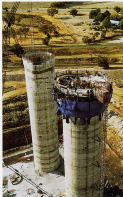
4. Shaft slip-forming, April 1996.
