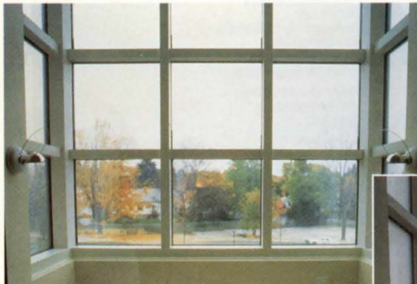
1. Smart glazing: clear to opaque.
