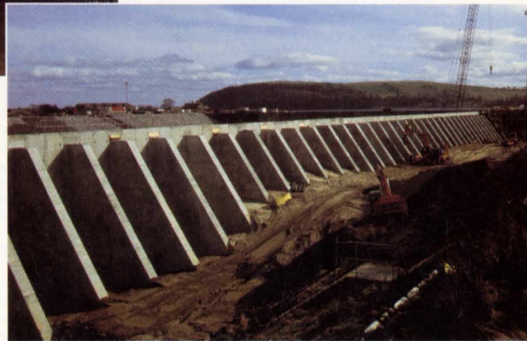
7. Back filling of the wall.
