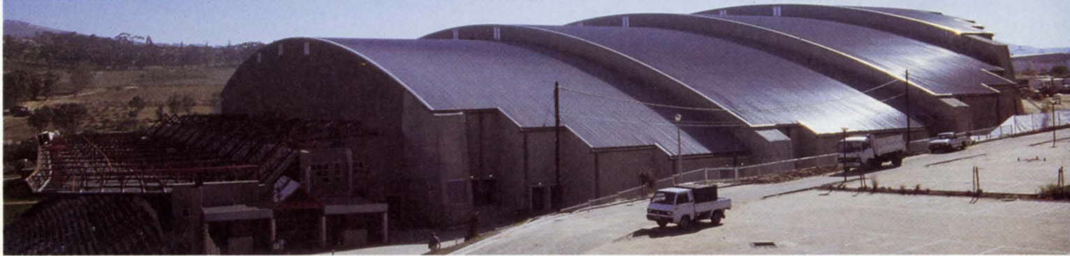
7. View of completed exterior, July 1997.
