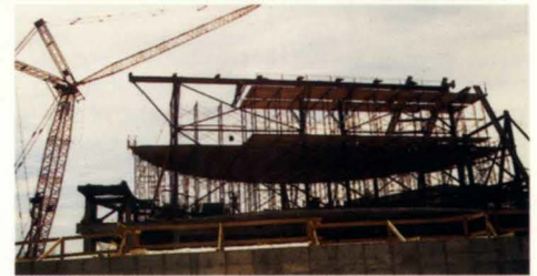
12. Temporary formwork for Gathering Space roof structure.
