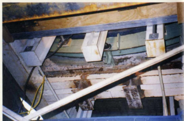
12. The disc still supported by the existing structure after being raised. The three vertical beams are part of the grillage. The new structure is installed below, ready for load transfer of the disc.
