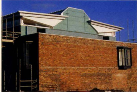
9. The condenser's location, behind the louvres.
