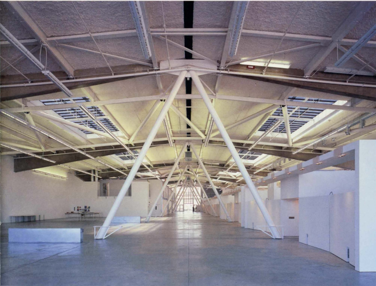
7. Interior view showing chevron braces and diaphragm trusses. Moveable partitions for graduate studios are to the right; enclosed classrooms and second floor graduate studios are to the left.
