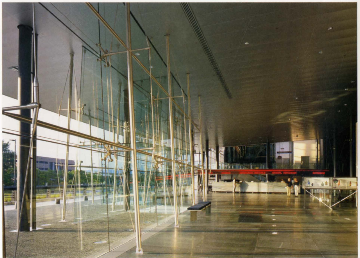
5 below: Glass curtain wall at entry level of Orientation Center.
