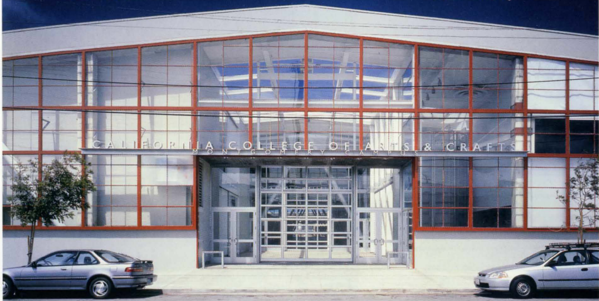
1. New main entrance to CCAC: the café is to the right and the Logan Galleries to the left.
