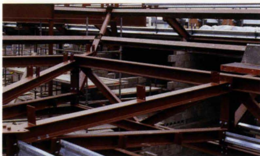
11. Roof steelwork at valley.
