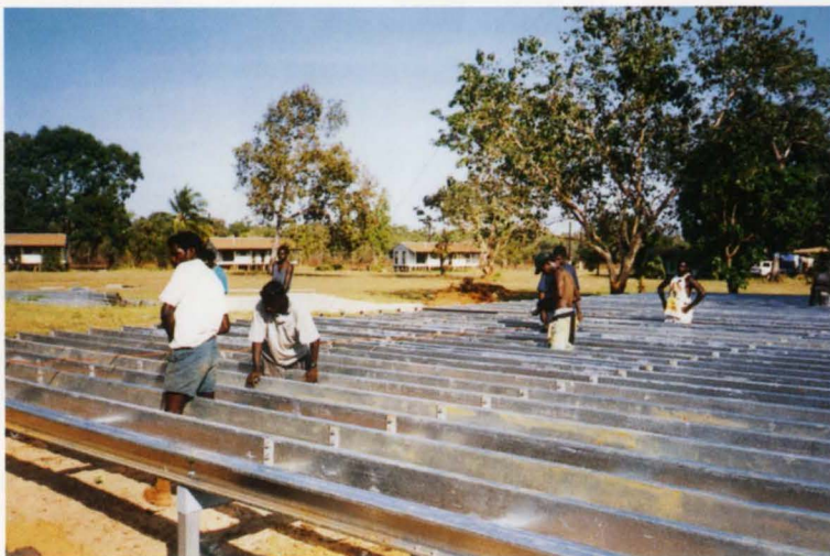
4. Community workers on housing site in the Northern Territory.
