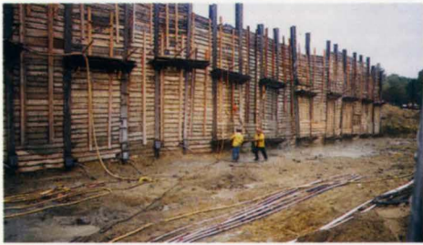
9. Waling structure for deep basements.
