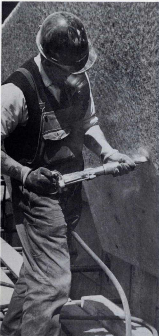
Fig. 12 Block 6. Pick-hammering with a chisel bit
