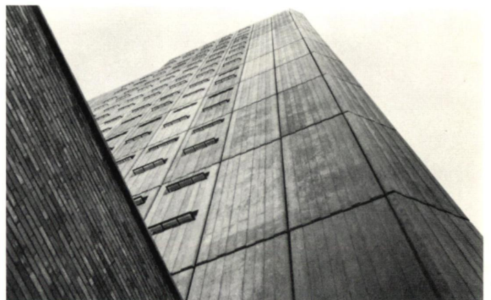
Fig. 24 Precast cladding units (Photo: Ove Arup & Partners Zimbabwe)
