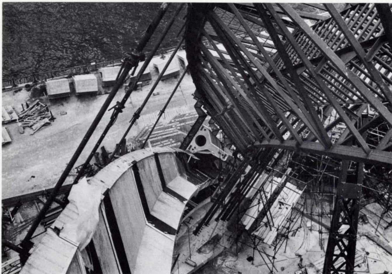
Fig. 17 View down a rib under construction. (Photo: G. Wood)
