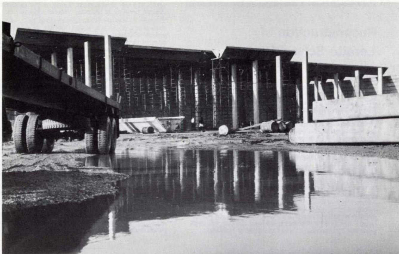
Fig. 11 top left Internal view Note method of ventilation control (Photo: Colin Westwood)
