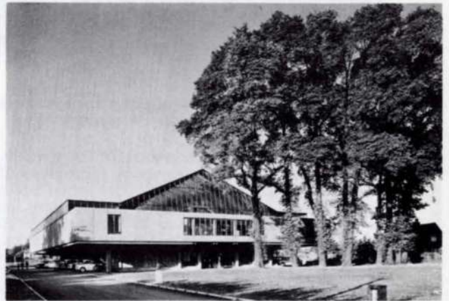
Fig. 11 Swimming Pool, Walton-upon-Thames, showing the twin beams which are bolted to the columns with glued interfaces. (Photo: Colin Westwood)
