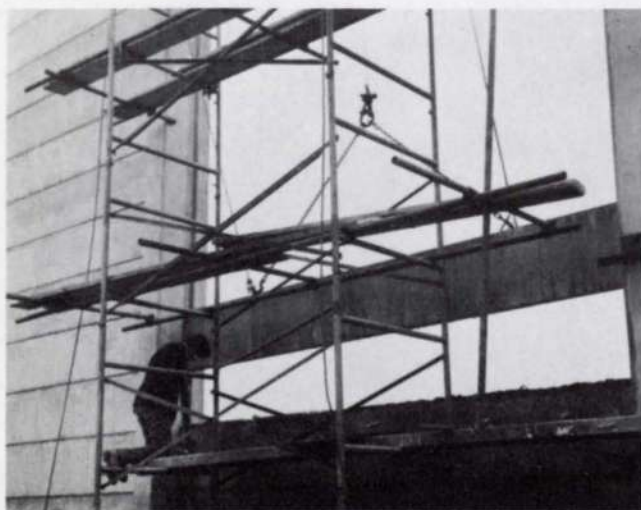
Fig. 16 below right Lifting hook on end diaphragm of roof unit (Photo: A. B. Gourlay)
