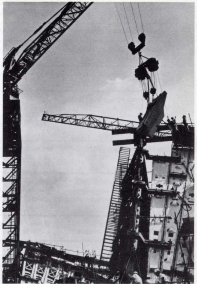
Fig. 16 Lifting a rib segment into position. (Photo: Max Dupain)
