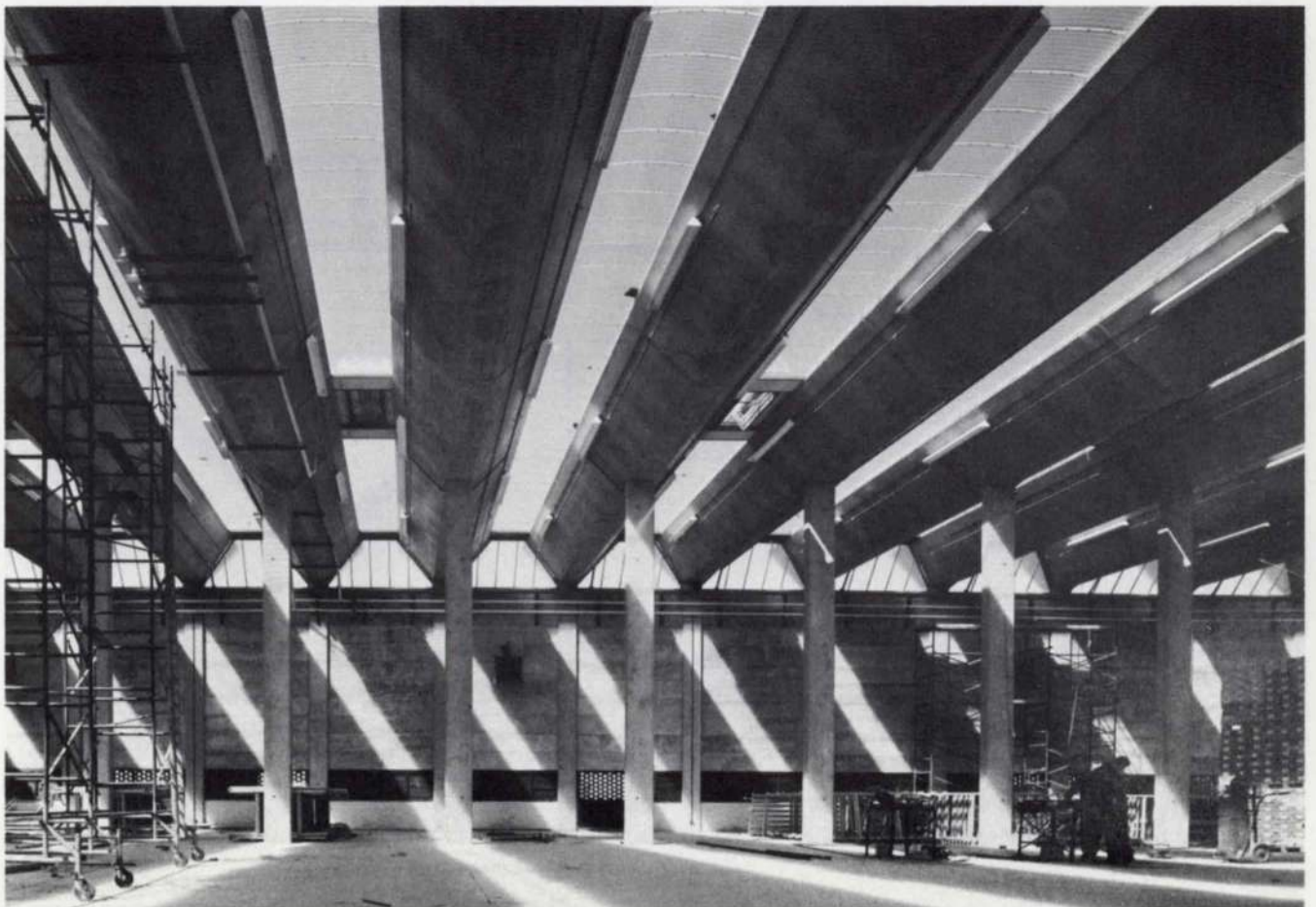
Fig. 6 above Precast concrete roof unit type B
