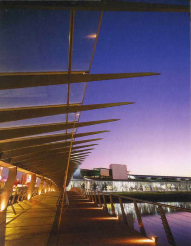
3: View along open side of footbridge to Southbank.
