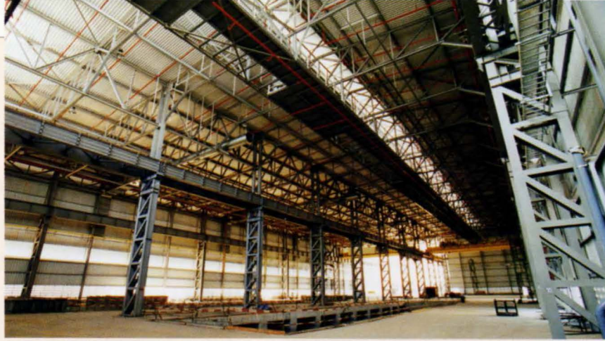
10. Thailand press shop prior to press installation.
