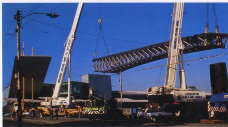
7: Installation under way.
