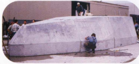
11. Shroud at the precasting yard.
