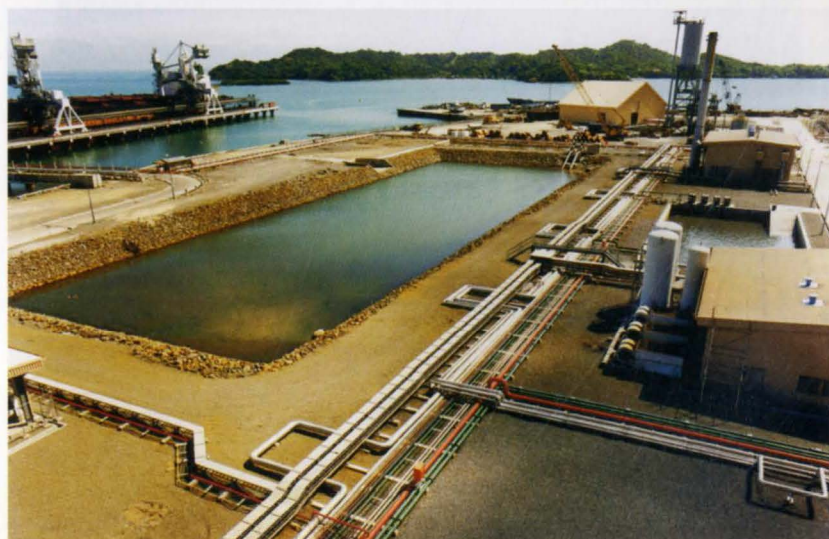
10 below: Site-wide services, including electrical distribution, potable water, seawater, fire-fighting, etc.
