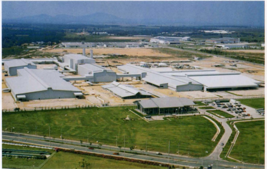
8. Aerial view of Thailand plant.
