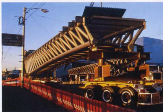
6: New bridge section sitting on existing bridge waiting to be installed.
