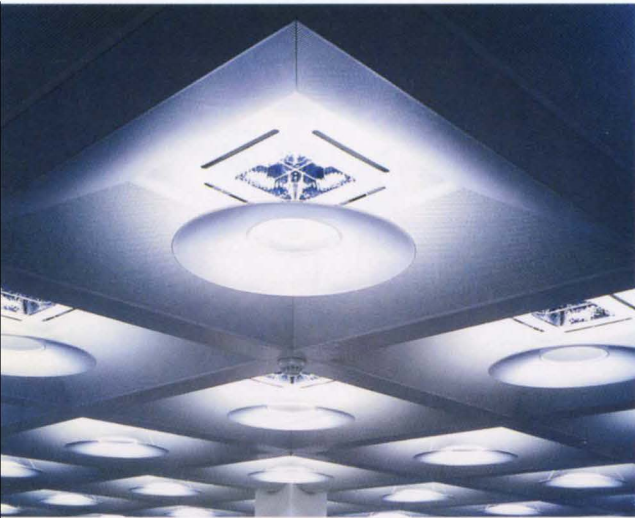
5. The specially designed luminaires for the dealer floor combine the recommended provision for VDU use with an uplit ceiling from a single standard fitting. This increases the apparent height of the space and avoids the gloomy interior that can result from sole use of a Category 1 luminaire.
