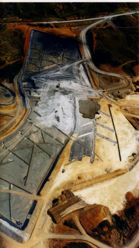
11. Ash disposal site, showing two storage cells under construction.
