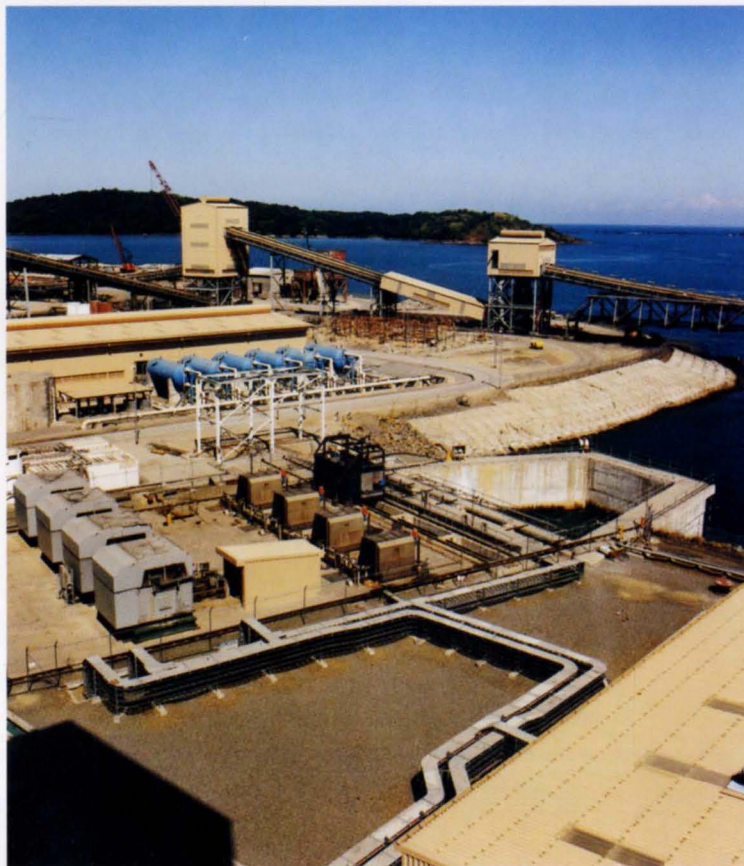
8. Cooling water intake and pumphouse.
