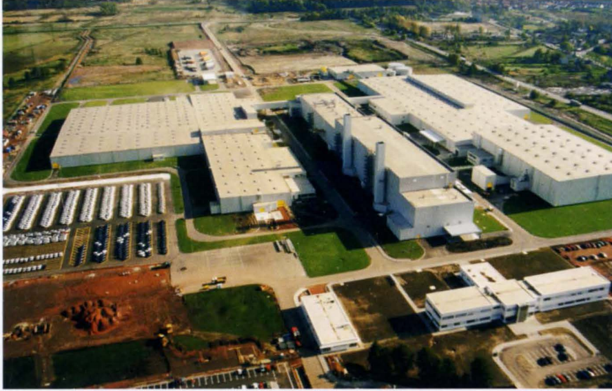
7. Aerial view of Poland plant.
