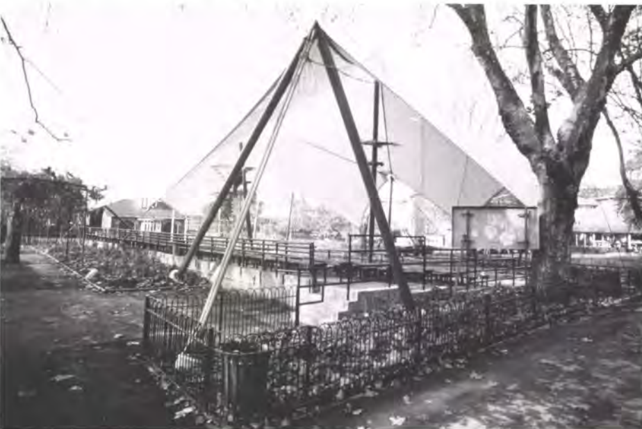
Fig. 7 London Zoo: PTFE coated glass canopy over Hummingbird Amphitheatre
