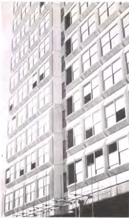
Fig. 9 Office block with loadbearing facade elements of precast concrete (Photo: Poul Beckmann)
