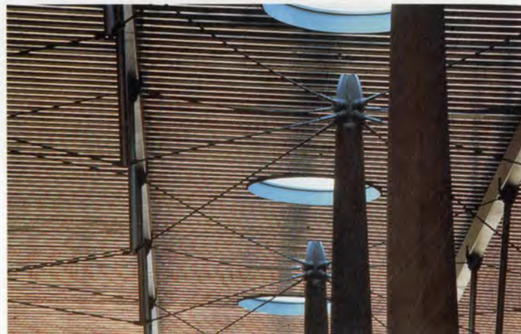
10. Skylight lenses over columns.
