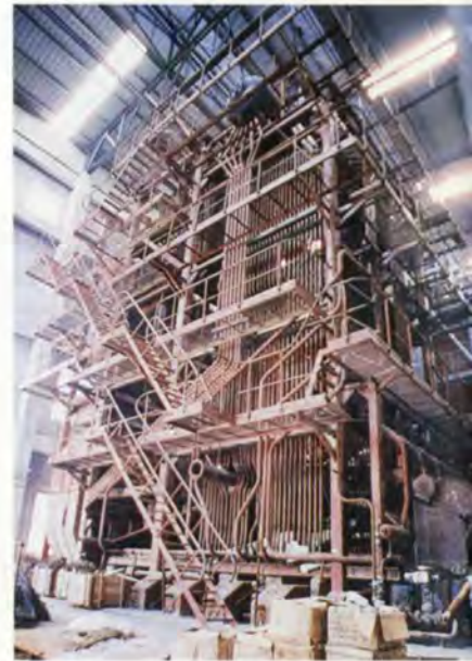
9. Boiler under construction in the Energy Centre.
