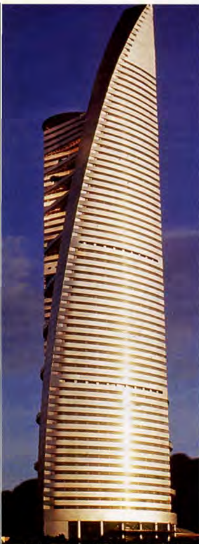
6. Telekom Malaysia HQ, Kuala Lumpur, planned to achieve level 5 integration.
