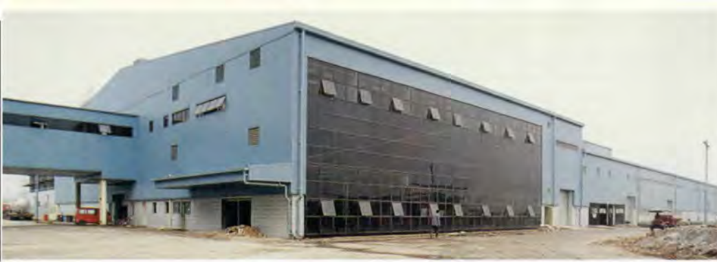
6. Offices in northwest corner of process building.
