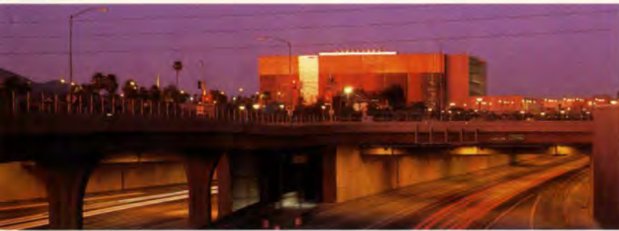
11. Library as seen atop I-10 freeway overpass.
