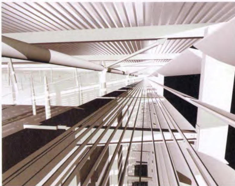
4. Aluminium louvres at roof level on the south façade.
