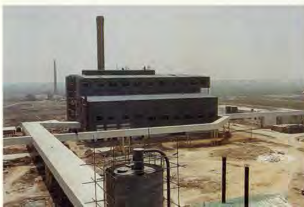
4. Construction progress, looking south at April 1996, showing the Energy Centre.
