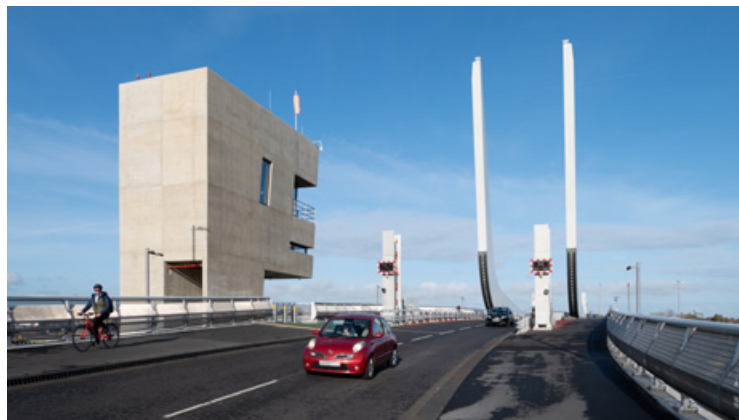
16: The drainage system can withstand a one-in-100-year rainfall event with a six-hour storm duration
