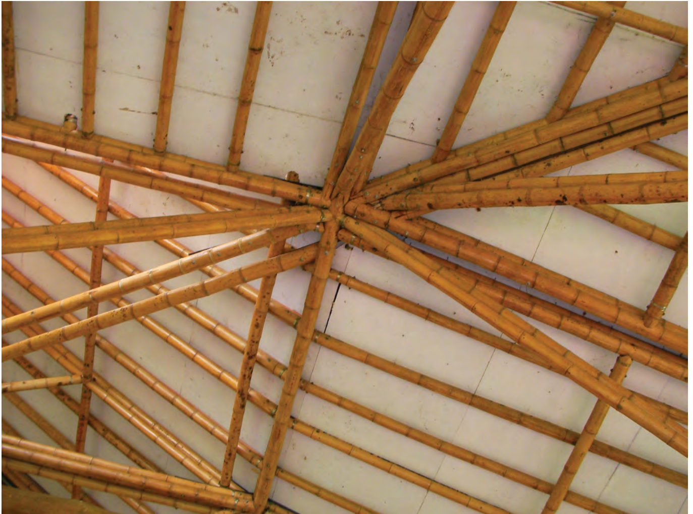
Figure 4.3: Joints that rely on the confluence of many elements can be problematic
