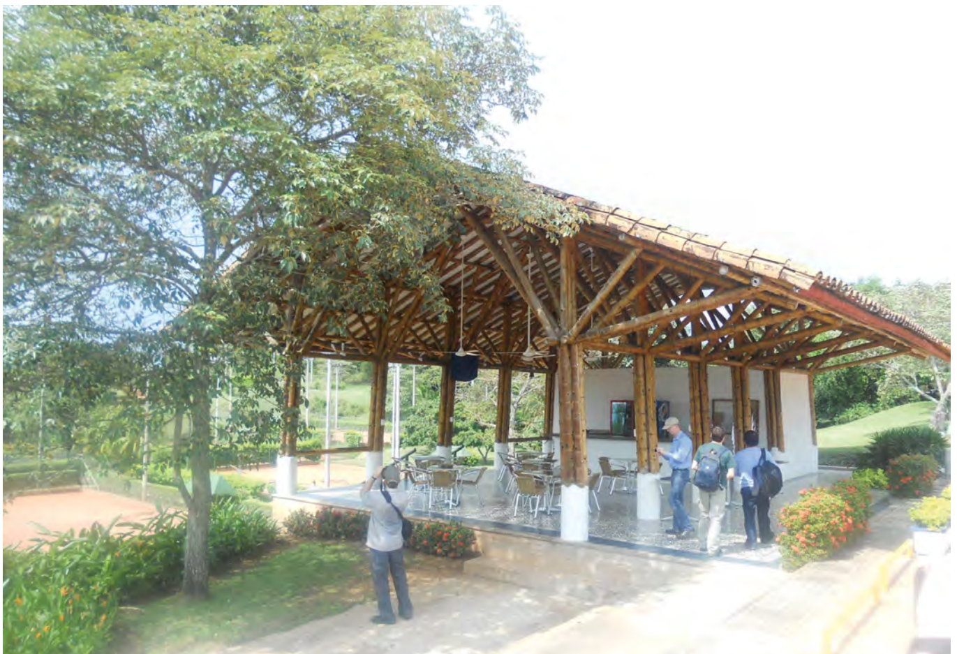
Figure 4.1: Fan-shaped roof truss
