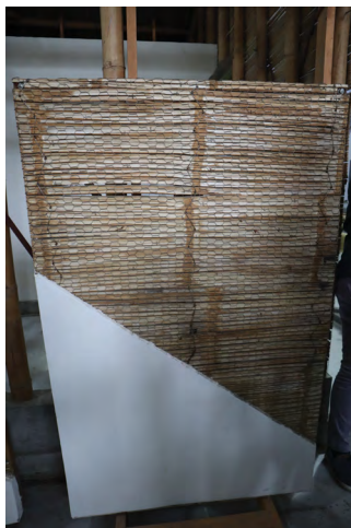
a) Chicken wire mesh on flattened bamboo
