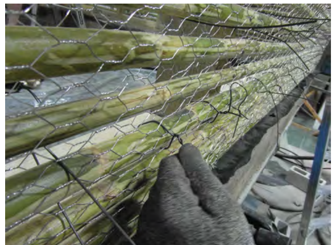
b) Chicken wire mesh either side of small-diameter cane
