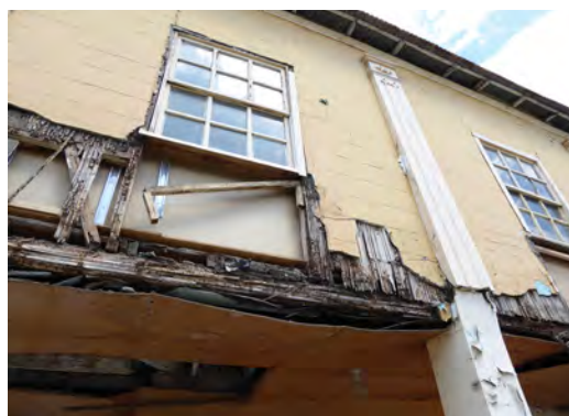
c) Rotten timber and bamboo inside a wall (water trap)
