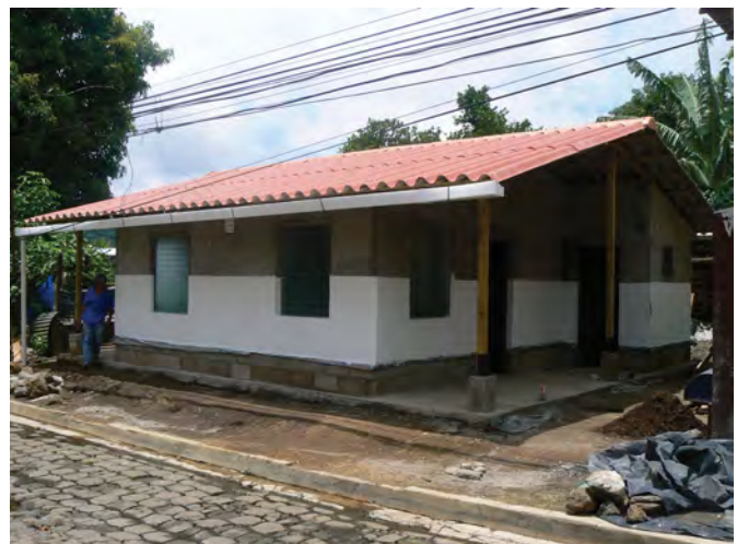
b) A modern bamboo house in El Salvador. The upstand elevating the structure, the render protecting the bamboo wall and the large roof overhang minimise the impact of driving rain
