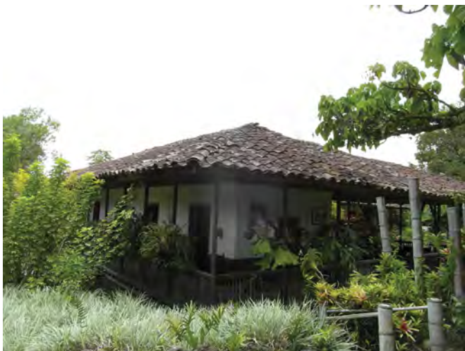
a) A traditional bamboo house in Colombia, over 100 years old. The perimetral veranda fully protects the walls from driving rain
