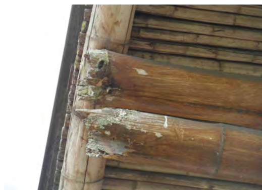
d) Rotten bamboo where a beam was exposed and collected water
