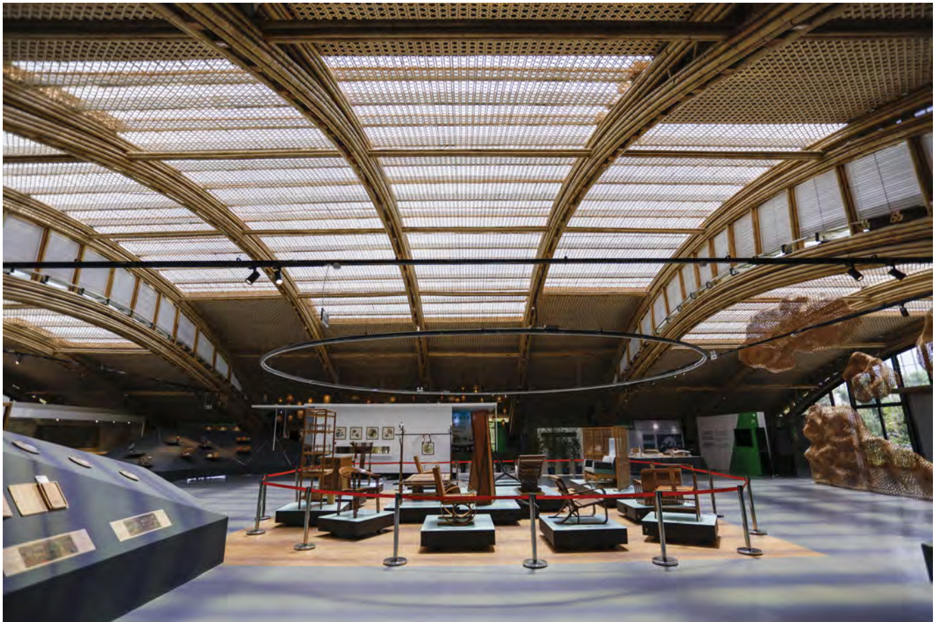
Figure 4.2: An arch structure using bamboo: INBAR Pavilion at 2019 Beijing International Horticultural Expo
