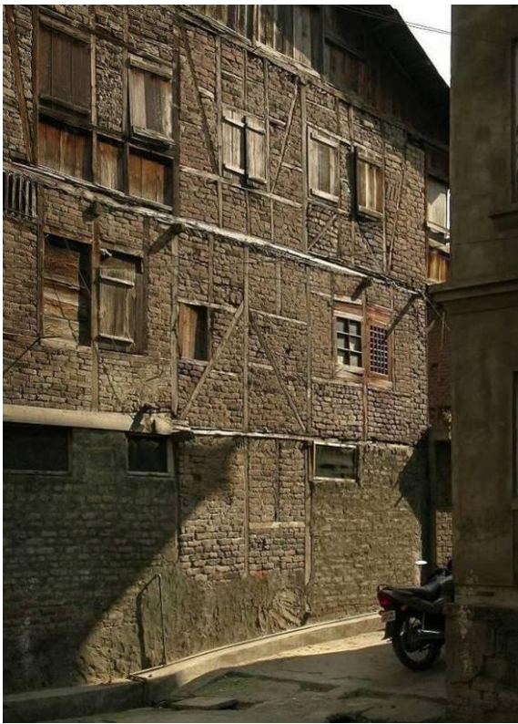
Figure A1-2 . Multi-storey Dhajji building in Shrinagar, India. Photo source © Randolph Langenbach.
