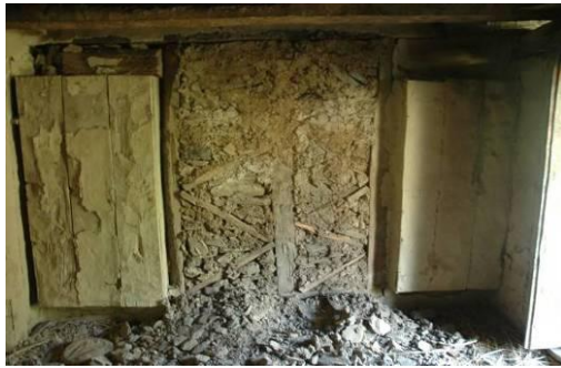
FigureA2-36 Wall built before the 2005 earthquake
