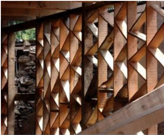
FigureA2-12 Timber frame ready to receive stone infill. Bracing has a zigzag pattern and bracing does not coincide/node-out.
