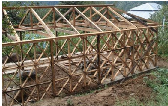
FigureA2-21 A view showing roof and braced timber frame
