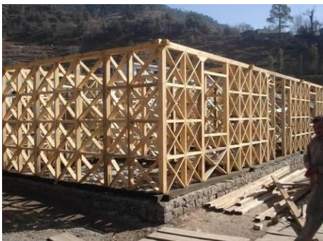
FigureA2-39 “Engineered” Dhajji building frame under construction
