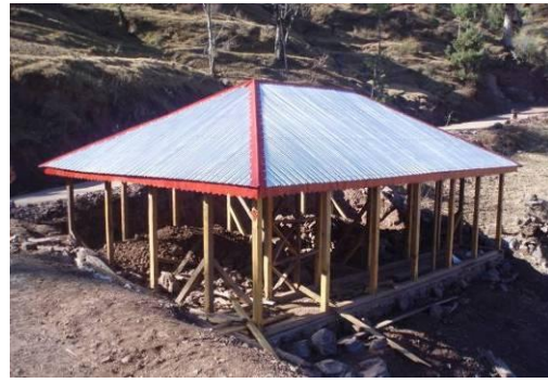
FigureA2-47 Simple frame at the start of the process of converting the posts into Dhajji walls with hipped roof. Note that gutters are not provided to any of the roofs.
