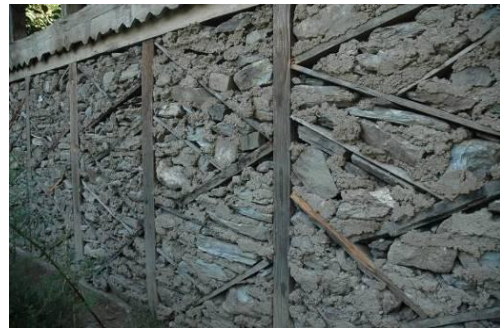
FigureA2-37 Wall built after the 2005 earthquake
