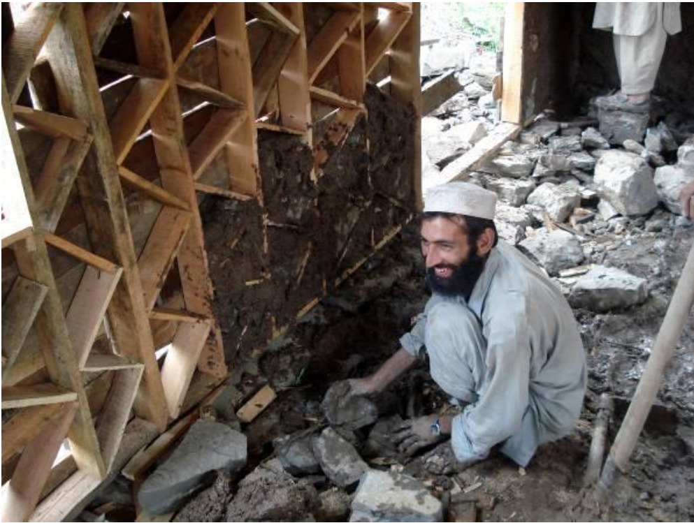
Figure 2-2 Typical dhajji dewari building under construction
