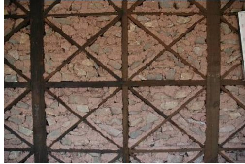
FigureA2-35 Reasonably cut stone laid with a lot of mud mortar. Note that the timber has been soaked in old engine oil as a way to give it some better protection against rotting.
