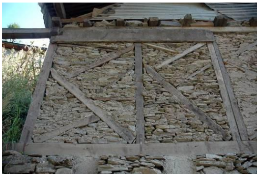
FigureA2-32 Bracing using large timber braces as timber resources are less constrained in the higher altitude. Note the more layered infill effect due to the type of locally available rock
