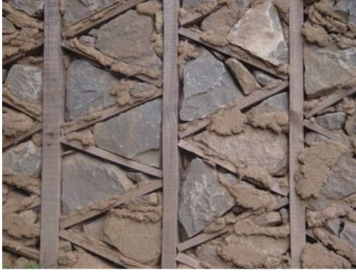
FigureA2-16 A completed wall, note large stones
