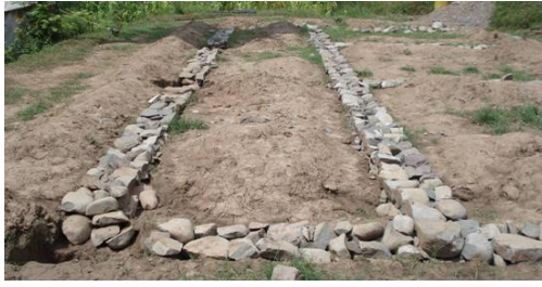
FigureA2-4 Stone strip footing under construction to raise the timber frame off the ground (new building)
