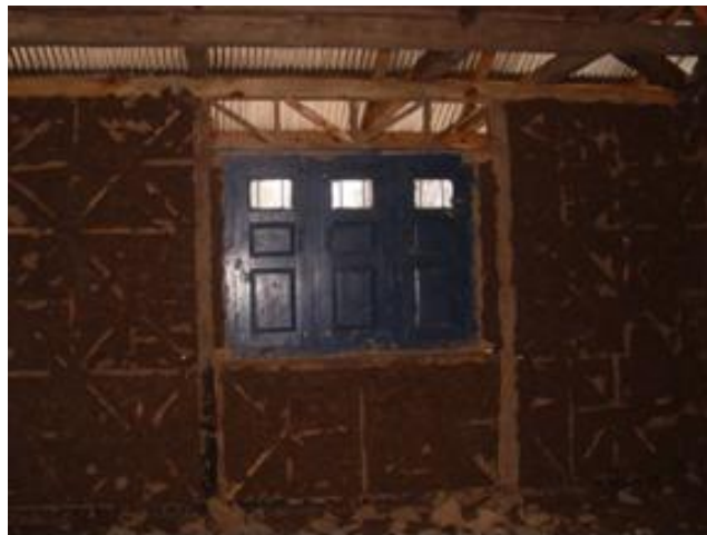
FigureA2-15 A wall ready to receive final coats of mud plaster (view taken from inside a building).
