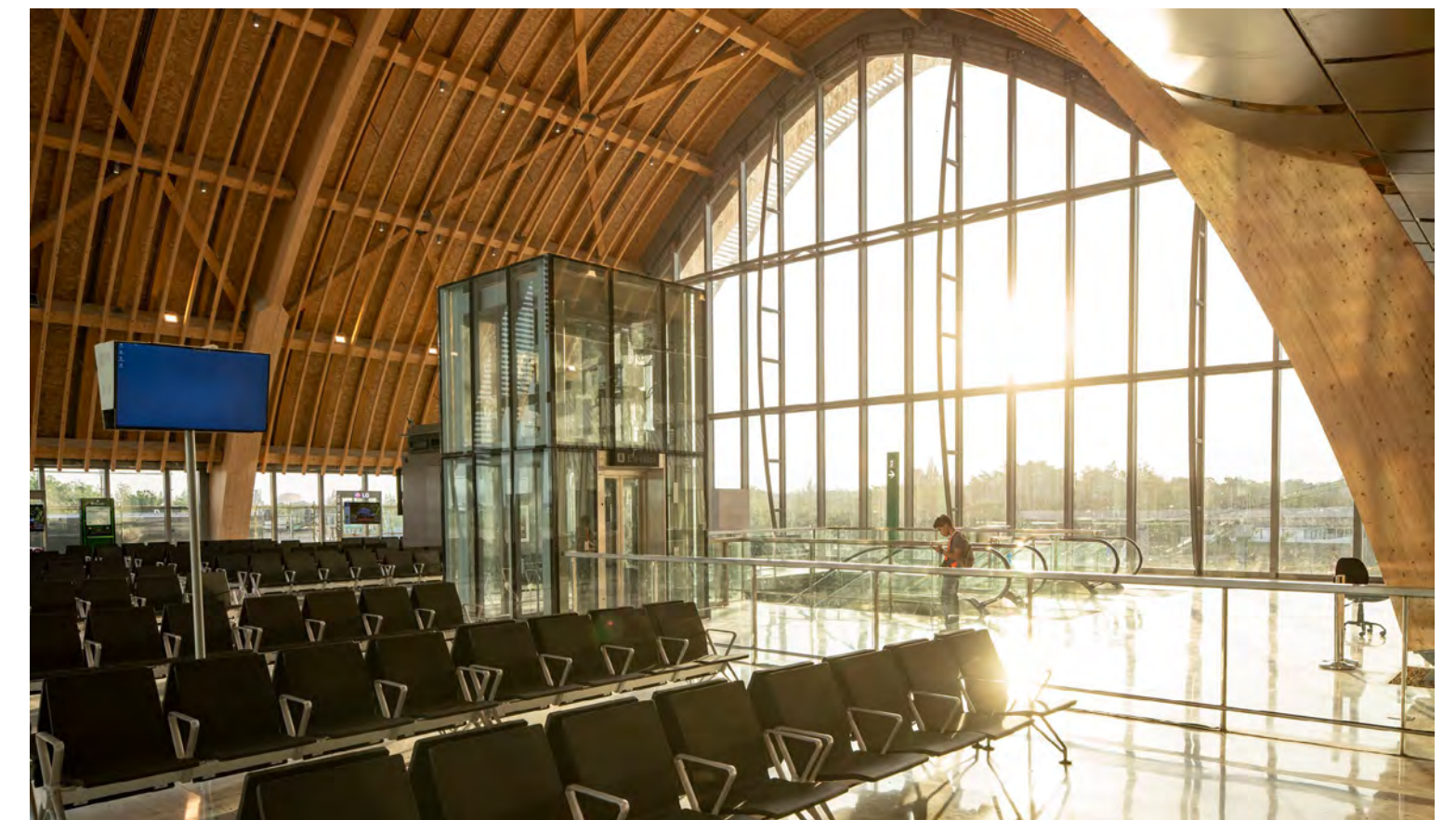
Terminal 2, Mactan Cebu Airport, Philippines
