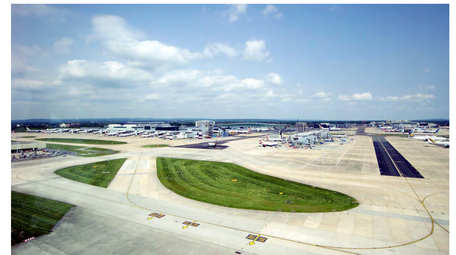
London Gatwick Airport Bridge, UK
