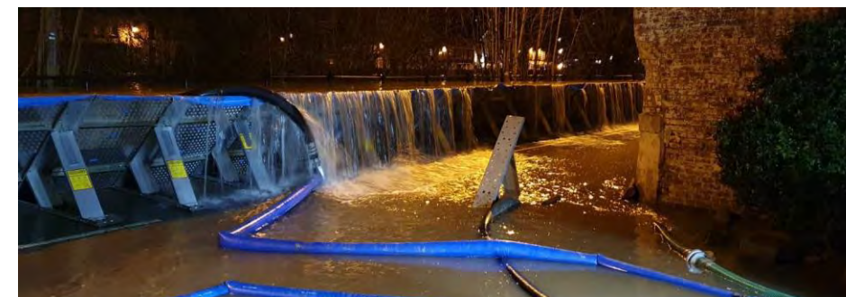
Figure 5: Flood barriers at Bewdley, England overtopping in February 2020.
